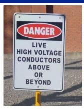
This sign is placed at locations to indicate the presence of live conductors adjacent to the work area. It will be accompanied, where necessary, by barriers or additional signs.
