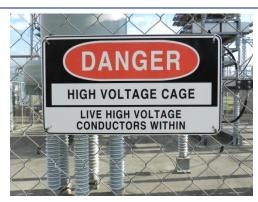
This sign is placed at locations to indicate a fully fenced or walled area, with a locked means of access, containing high voltage exposed conductors which do not maintain standard safety clearances.
