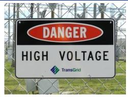
This sign is placed at locations to indicate that there are conductors, which should be regarded as live and from which persons need to maintain safe approach distances.
