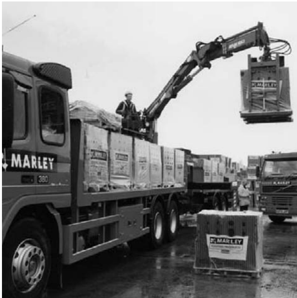
Figure 5.2 Unloading roofing tiles
