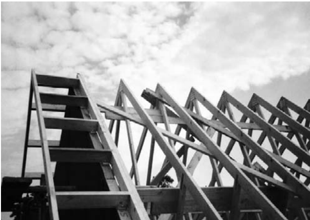
Figure 3.26 A trussed roof with diagonal wind bracing and showing a gable ladder (left of picture)
