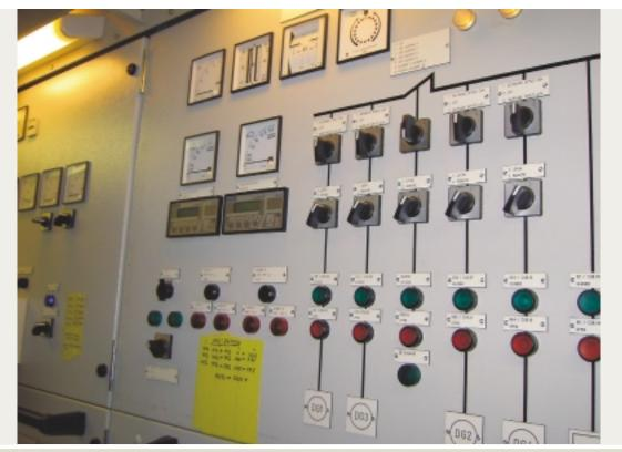
Fig. 6 - Back-up control at the main switchboard in case of PMS failure.
