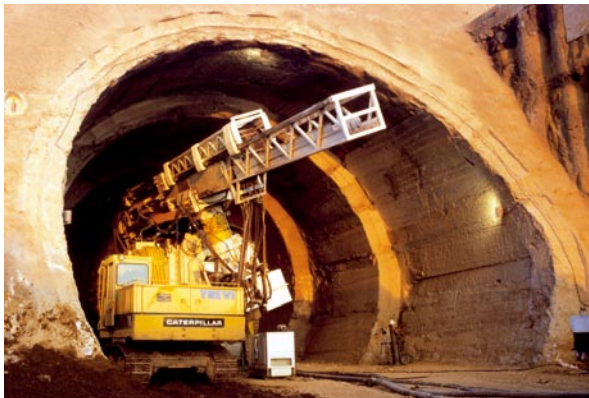
Fig. 9.6 Pretunnel operations (high speed/high capacity Rome-Naples railway line, Castello 1 tunnel)
