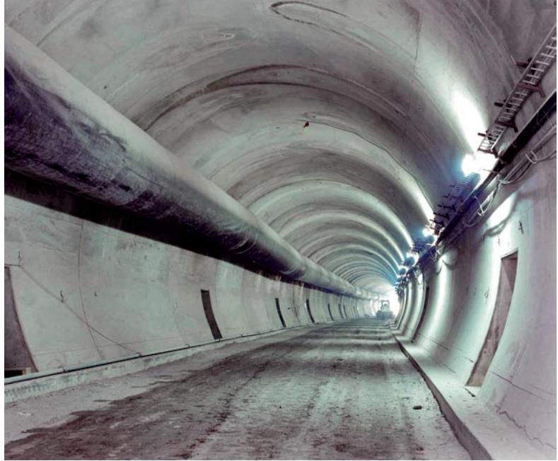
Cavity confinement by means of a final lining: final lining in concrete (Ancona-Bari railway line, Vasto tunnel, 1996, ground: clayey silts, max. overburden: ~ 100 m)
