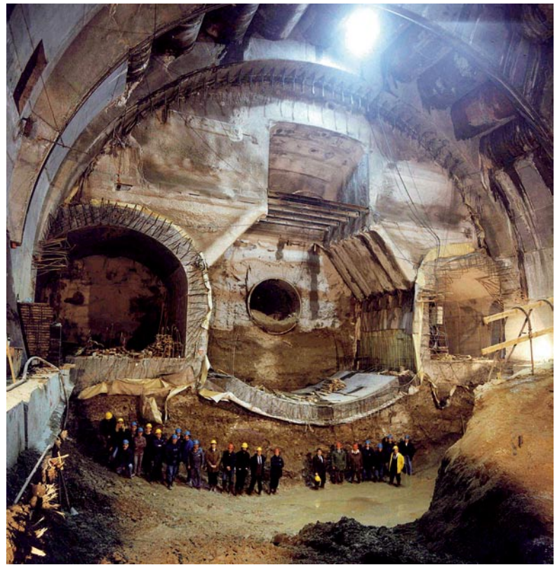
Fig. D.6 Venezia Station on the Milan urban link railway line: the full cross section
