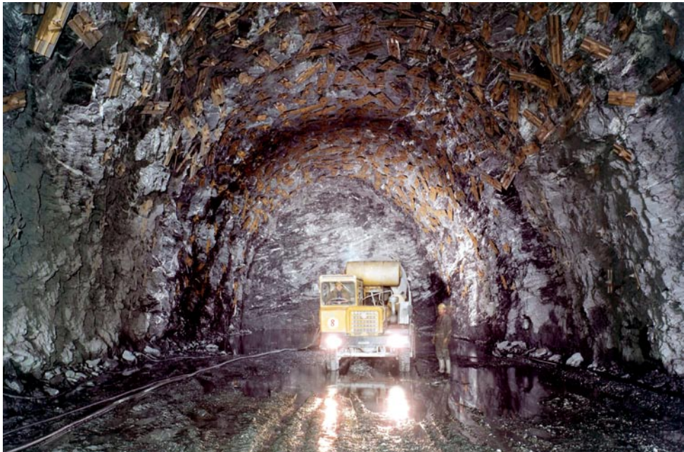
Radial bolting (Frejus motorway tunnel)
