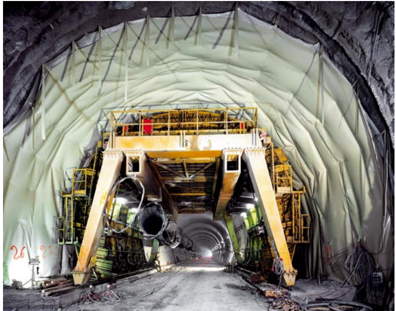
Waterproofing: the PVC sheath placed just before the final lining is cast (Ancona-Bari railway line, Vasto tunnel, 1996, ground: clayey silts, max. overburden: ~ 100 m)
