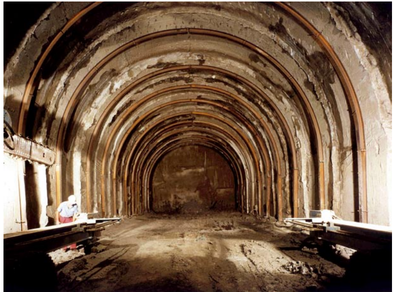
Cavity preconfinement by means of full face mechanical precutting: view of preliminary lining consisting of mechanically precut tiles in the same tunnel as above
