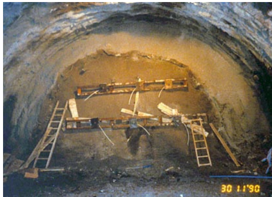
San Vitale Tunnel: the half cross section face supported by I-beams and tie rods after tunnel advance was abandoned
