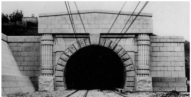
Bologna-Florence Direttissima Line, the Grand Apennine Tunnel: the portal on the Florence side
