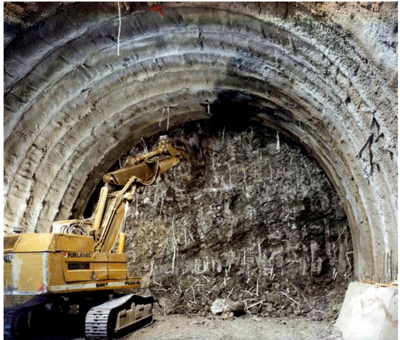
Excavation: mechanical excavation of the core-face using a hammer (Caserta-Foggia railway line, S. Vitale tunnel, 1993, ground: scaly clay, overburden: ~ 130 m)
