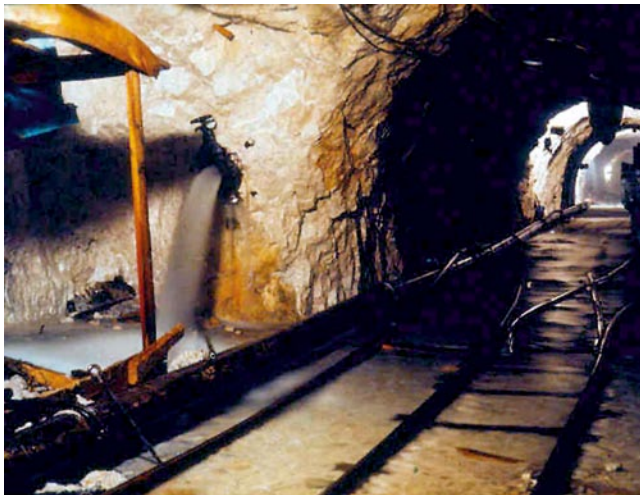
Wall drain (Gran Sasso tunnel)
