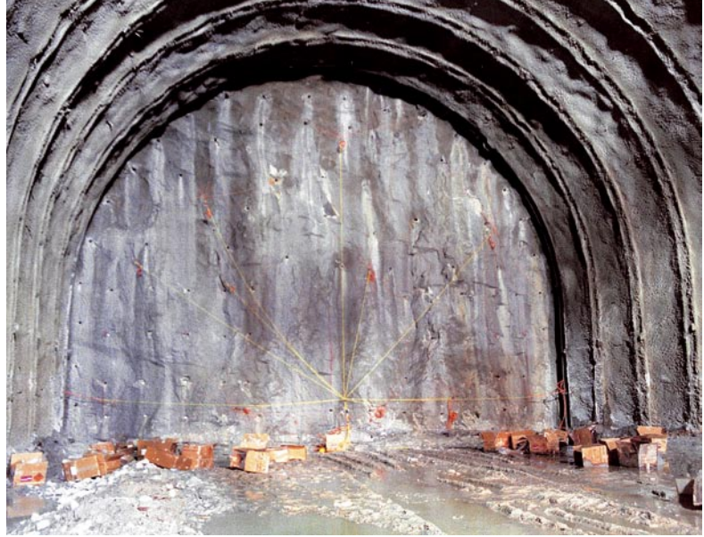
Excavation: the core-face with the charges set before detonation (new high speed/high capacity railway line between Bologna and Florence on the Pianoro tunnel, 1999, ground: weakly cemented sandstone, overburden: ~ 70 m)
