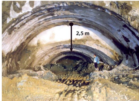
The Tasso tunnel which collapsed during half face advance (NATM)
