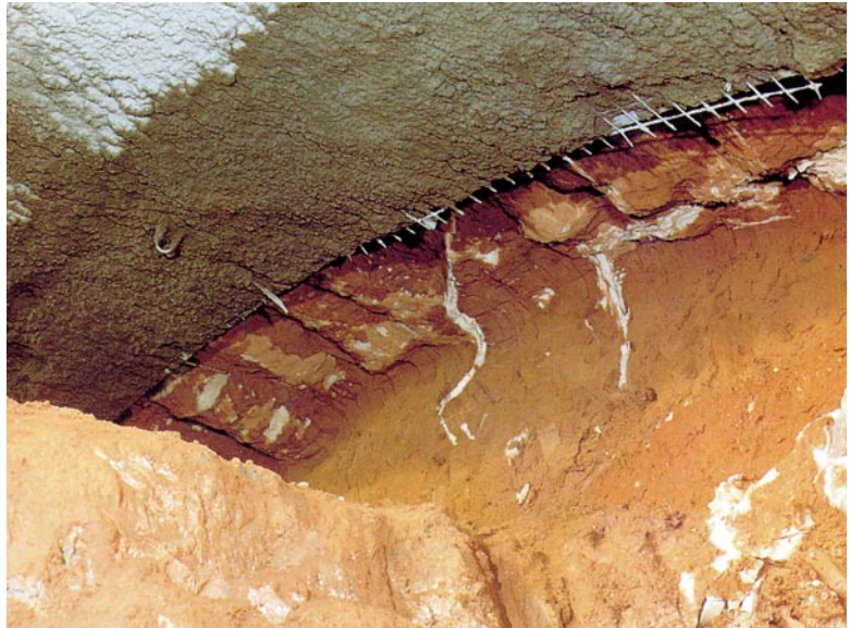
Cavity preconfinement by means of truncated cone 'umbrellas' consisting of sub horizontal columns of ground, side by side, improved by means of jet-grouting: detail of the treatment (underpass of the Campinas railway yard in Brazil, 1987, ground: sand, overburden: 2.5–4 m)
