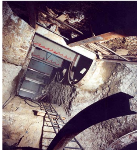
Venezia Station on the Milan urban link railway line: the cut of the pipes (minitunnels) for creating the transverse arches
