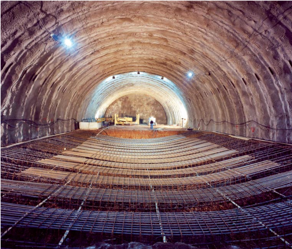
Reinforcement of the tunnel invert (Appia Antica tunnel, Rome motorway ring road)
