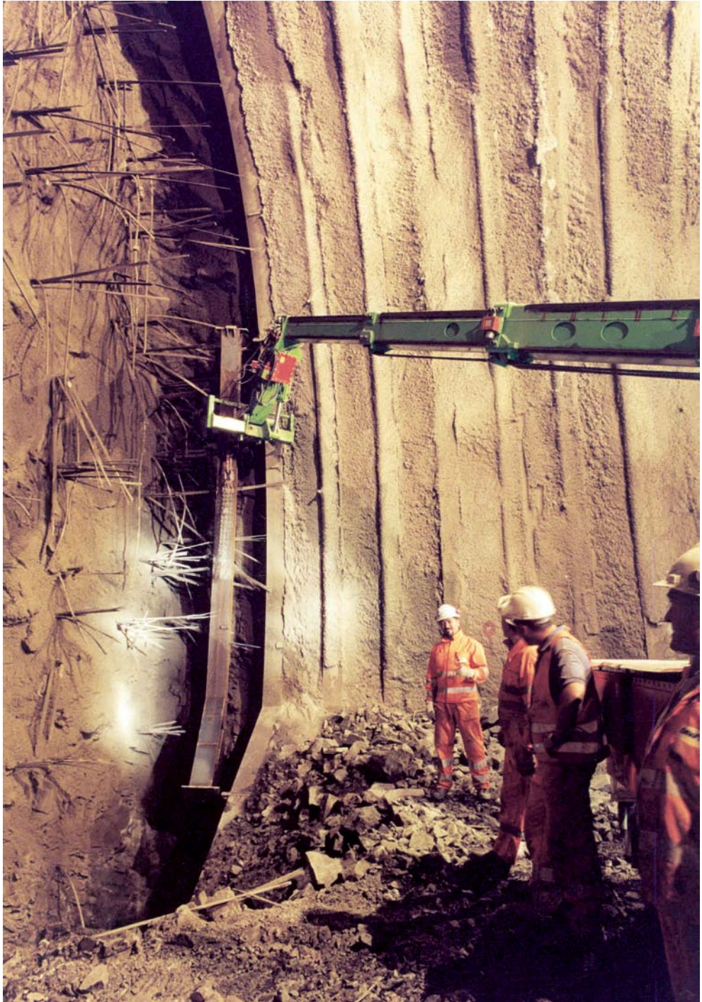
High speed/capacity Bologna-Florence railway line, Pianoro tunnel. Placing a steel rib next to the face
