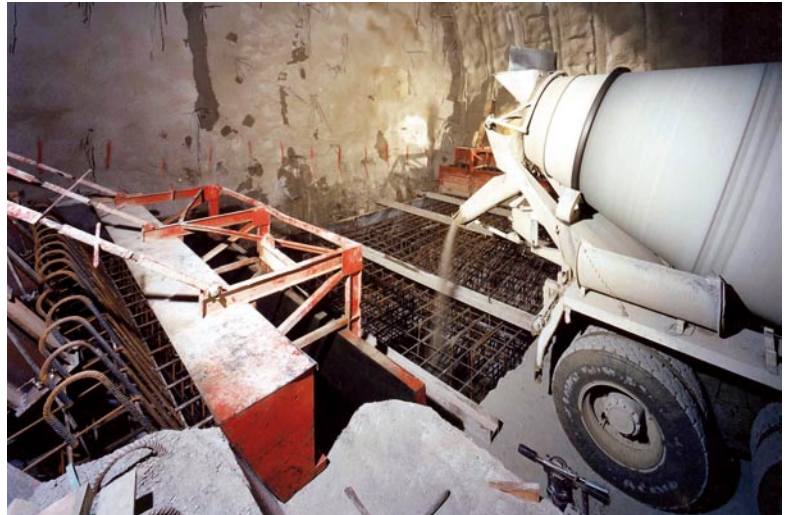
Cavity confinement by means of a tunnel invert: casting the tunnel invert immediately behind the face (TGV Méditerranée, Lyon-Marseille railway line, Tartaignille tunnel, 1997, ground: clay, max. overburden: ~ 110 m)
