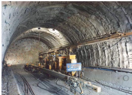
San Vitale Face: the face during fibre glass reinforcement operations with full face advance
