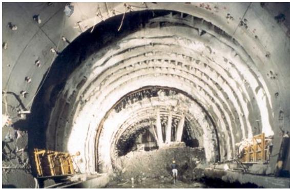
Fig. 2.5 Collapse of the cavity (S.Stefano Tunnel)
