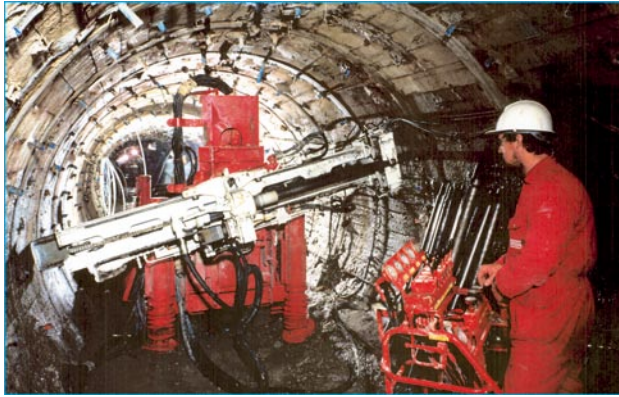
Fig. 9.28 Conventional cement injections from a pilot tunnel
