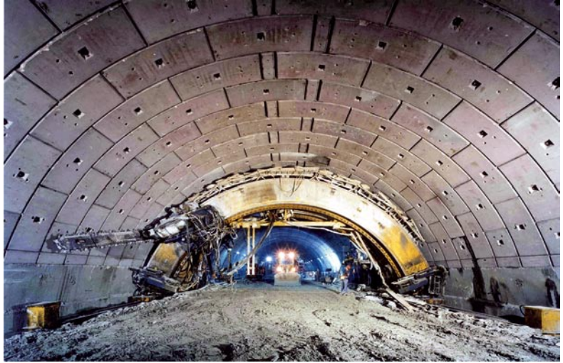
Cavity preconfinement by means of full face mechanical precutting: 21.5 m span mechanical precutting machine (line A of the Rome metro, Baldo degli Ubaldi Station, 1996, ground: clay with sand strata, overburden: ~ 18 m)
