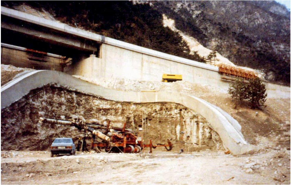
A shell of columns of ground improved by vertical jet-grouting constructed for the portal of the S. Leopoldo tunnel under the motorway embankment
