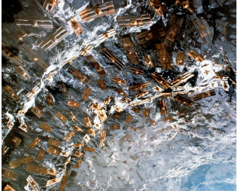
Confinement of the cavity by means of radial rock bolts: intervention using Anchral rock anchors (Frejus motorway tunnel, 1978, ground: crystalline schistose limestone, max. overburden: ~ 1700 m)
