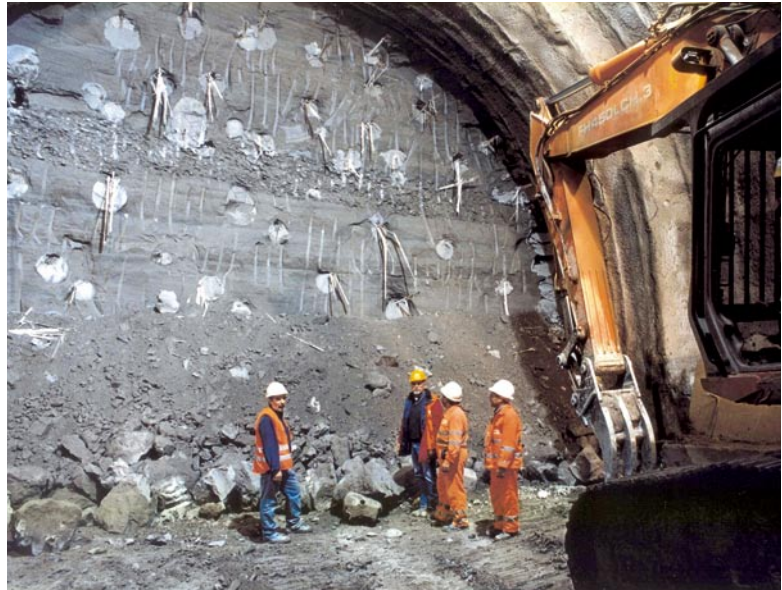
Cavity preconfinement after reinforcement of the core-face with fibre glass reinforcement: the face reinforced with fibre glass elements inserted into micro-columns of ground created by means of jet-grouting (high speed/high capacity railway line between Bologna and Florence, Firenzuola tunnel, 2000, ground: silt and silty sand with interbedded gravel, overburden: ~40 m)
