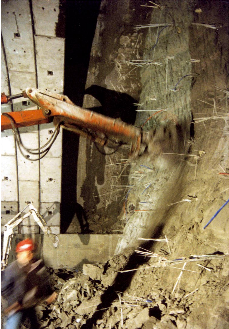
Excavation: giving the face a concave shape (line A of the Rome metro, Baldo degli Ubaldi Station, 1996, ground: clay with sand strata, overburden: ~ 18 m)
