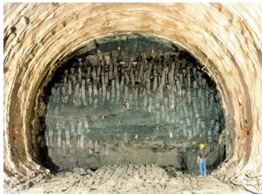
The Tasso tunnel during full face advance after reinforcing the advance core with fibre glass tubes
