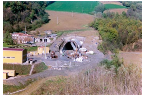
Pianoro Tunnel (new high speed/capacity railway line between Bologna and Florence): the progression of the works for the South portal built in semi-cohesive ground using jet-grouting technology
