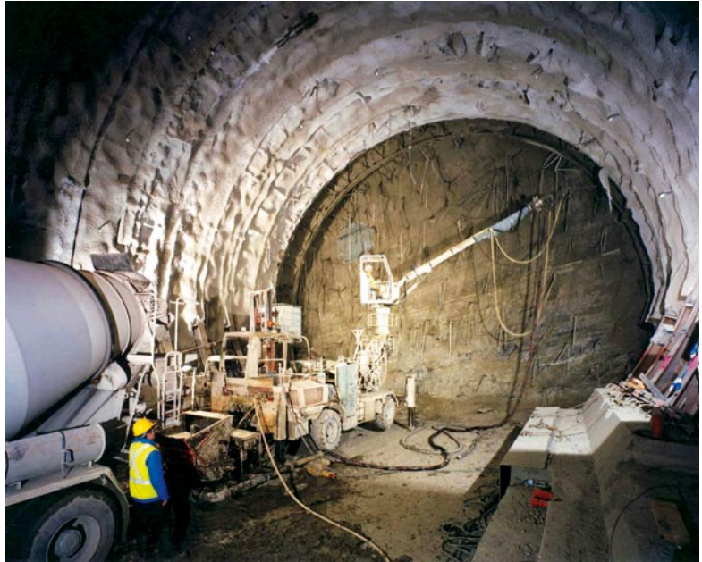
Confinement of the cavity by means of a preliminary lining shell of shotcrete: placing of the shell (TGV Méditerranée, Lyon-Marseilles railway line, Tartaignille tunnel, 1997, ground: clay, max. overburden: ~ 110 m)
