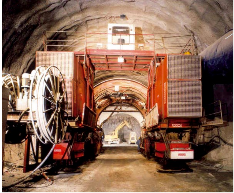
Cavity preconfinement by means of full face mechanical precutting: the equipment (tunnels on the high speed/high capacity Milan-Rome-Naples railway line between South Arezzo and Figline Valdarno, 1988, ground: sandy silt, max. overburden: ~ 90 m)
