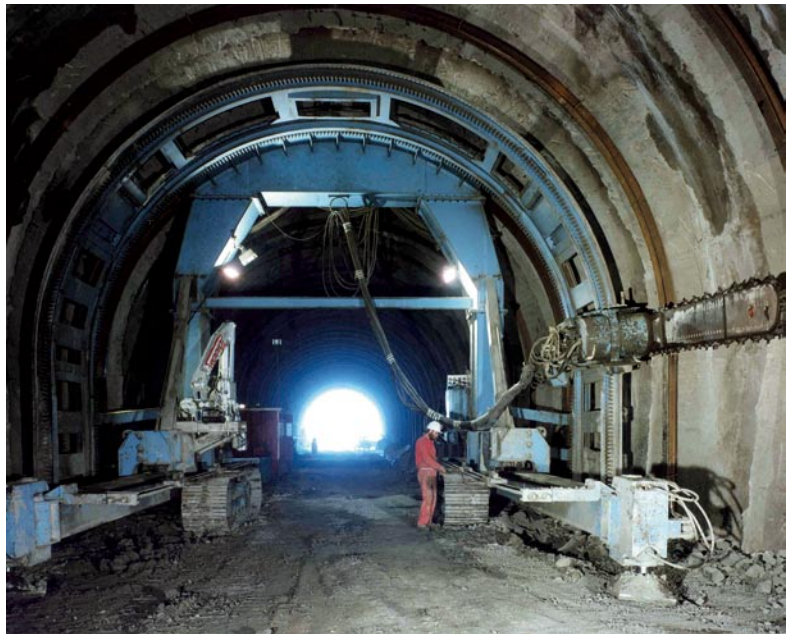
Cavity preconfinement by means of full face mechanical precutting (Sibari-Cosenza railway line, tunnel 2, 1985, ground: clay and silt, max. overburden: ~ 110 m)
