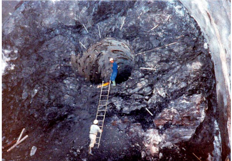
Confinement of the cavity by means of radial rock bolting: effect of rock bolting performed from a pilot tunnel (Udine-Tarvisio railway line, Malborghetto tunnel, 1986, ground: Ugovizza Breccia, overburden: ~ 70 m)
