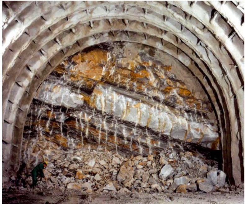
Excavation: the rock face after detonation of the charges (Genoa- Ventimiglia railway, S. Stefano tunnel, 1984, ground: clayey sandy-schists, overburden: 120 m)
