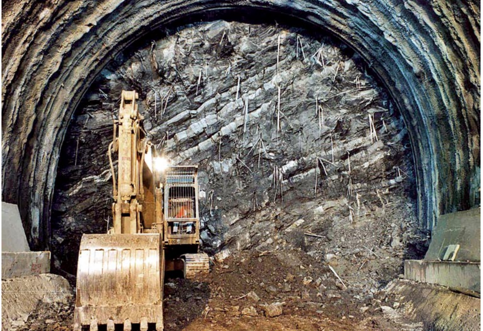
Monte Bibele Tunnel. View of the face while tunnelling through the Monghidoro Flysch, overburden: ~ 200 m)
