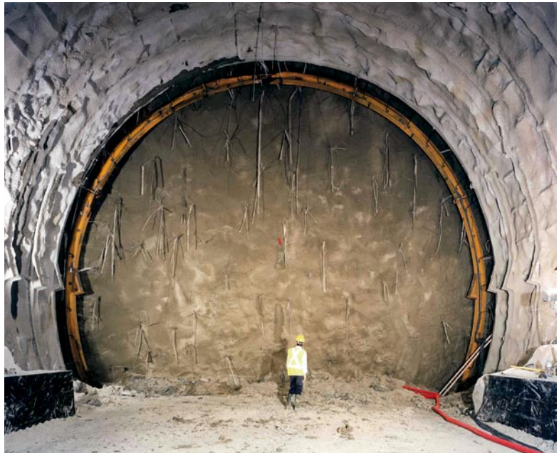
Confinement of the cavity by means of a preliminary lining shell of shotcrete: view of the sprayed face (TGV Méditerranée, Lyon-Marseilles railway line, Tartaignille tunnel, 1997, ground: clay, max. overburden: ~ 110 m)
