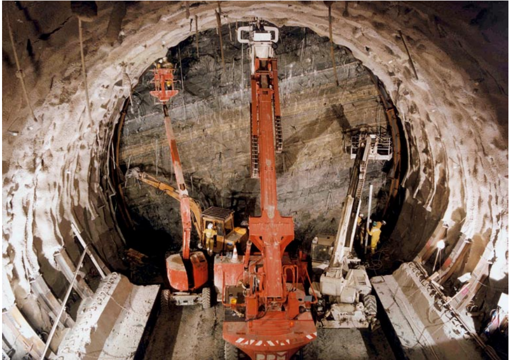
Fig. C.8 Placing of steel ribs
