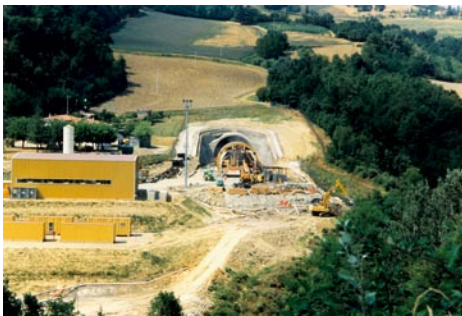
Pianoro Tunnel (new high speed/capacity railway line between Bologna and Florence): the progression of the works for the South portal built in semi-cohesive ground using jet-grouting technology
