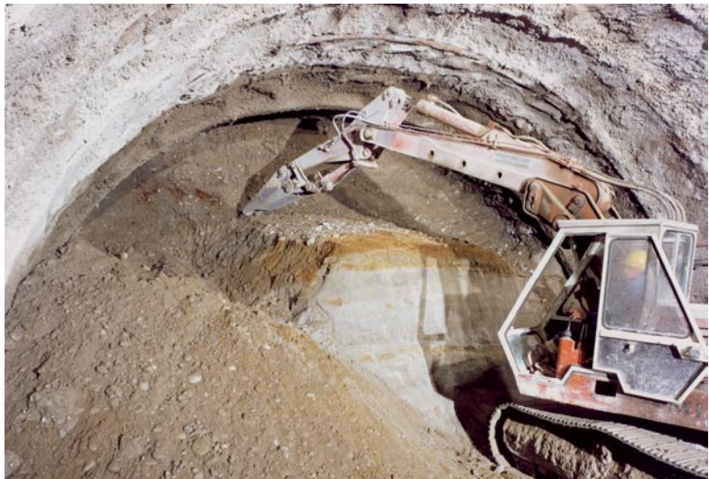
Mechanical excavation using a hydraulic demolition hammer
