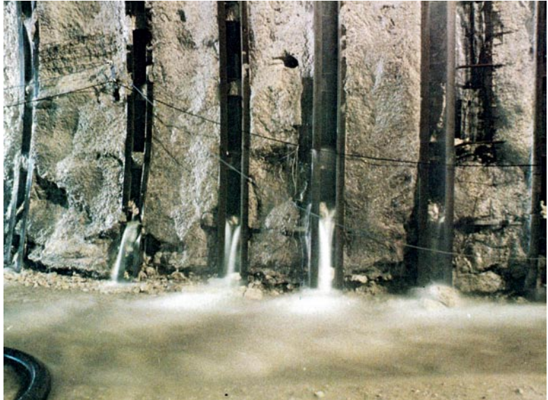
Cavity preconfinement by means of truncated cone 'umbrellas' of drainage pipes ahead of the face: water drainage through NP jointed steel ribs (Gran Sasso motorway tunnel, construction site on Casale S. Nicola side, 1974, ground: limestones, overburden: ~ 800 m, water head: ~ 600 m)
