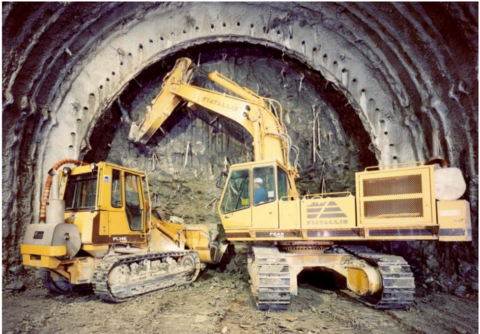
The "Vasto" tunnel (Ancona-Bari railway line), 1991, ground: clayey silts, overburden <math>< 50\text{ m}</math>. Top: reinforcement of the advance core with fibre glass reinforcement; bottom: excavation for tunnel advance
