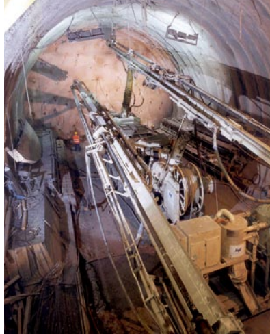
Raticosa Tunnel. Two moments in the reinforcement of the advance core using fibre glass structural elements. Drilling and insertion (left); cementation (right)
