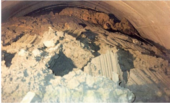
Fig. 2.14 Failure of the core-face because of extrusion (Vasto Tunnel)
