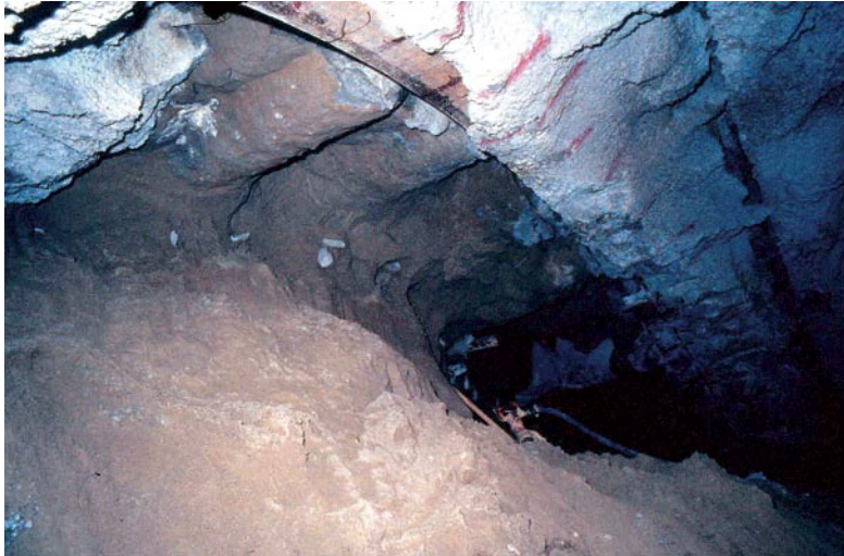
Fig. 9.23 Detail of columns of ground improved by means of horizontal jet-grouting (Milan-Chiasso railway line, M. Olimpino 2 tunnel, 1984, ground: alluvial, overburden: ~ 50 m)
