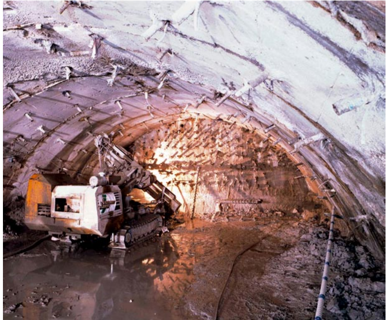
Cavity preconfinement by means of truncated cone 'umbrellas' of ground improved by conventional grout injections (Ancona-Bari railway line, Vasto tunnel, 1996, ground: silty clay, overburden: ~ 35 m)
