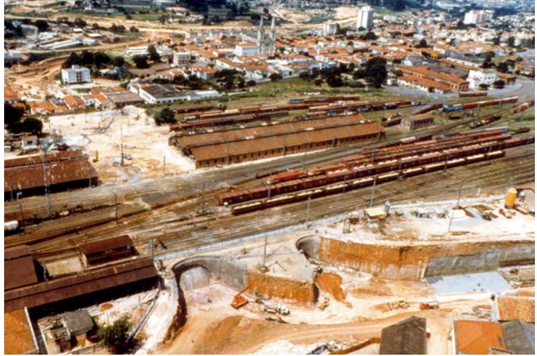
Cavity preconfinement by means of truncated cone 'umbrellas' consisting of sub horizontal columns of ground, side by side, improved by jet-grouting: view of the construction site for the construction of the underpass of the Campinas railway yard in Brazil (1987, ground: sand, overburden: 2.5–4 m)
