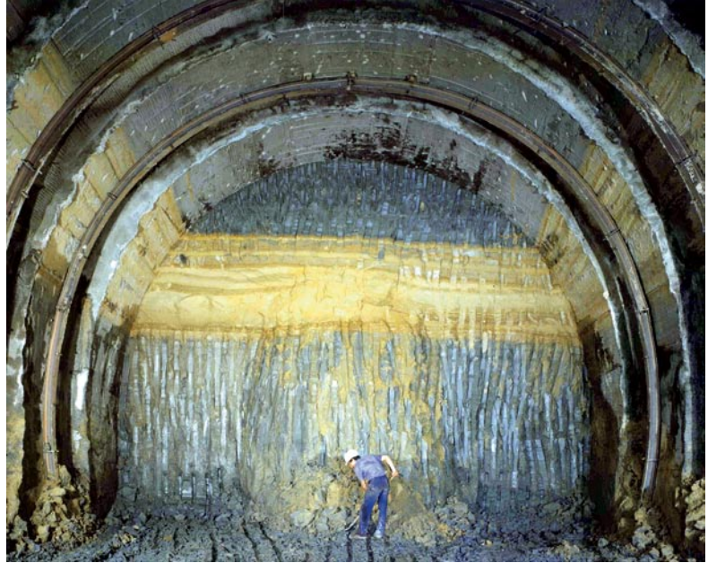
Cavity preconfinement by means of full face mechanical precutting: view of the core-face protected by a mechanically precut shell (Sibari-Cosenza railway line, tunnel 2, 1985, ground: clay and silt, max. overburden: ~ 110 m)
