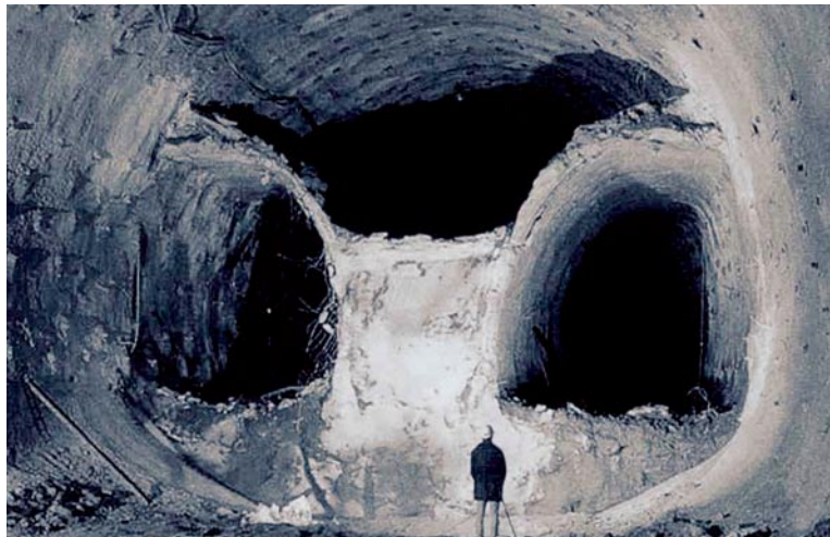
Typical tunnel advance following complete division of the face, advised by the NATM in “squeezing” or loose grounds
