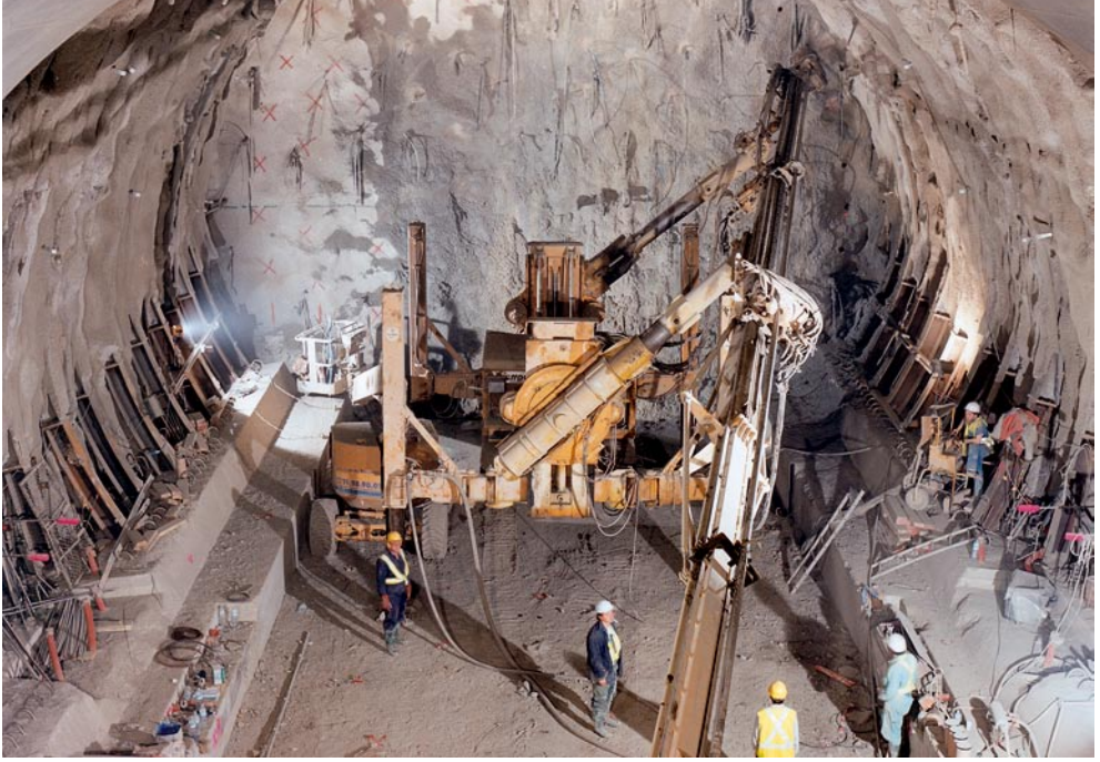
Fig. C.7 Reinforcement of the advance core
