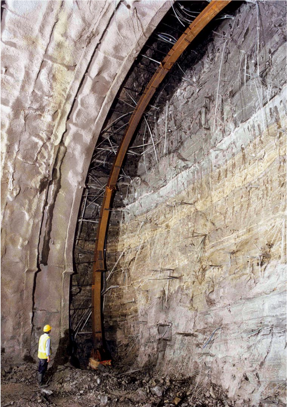
Cavity preconfinement after reinforcement of the core-face with fibre glass reinforcement: detail of the reinforced face (TGV Méditerranée, Lyon-Marseille railway line, Tartaguille tunnel, 1997, ground: clay, max. overburden: ~ 110 m)
