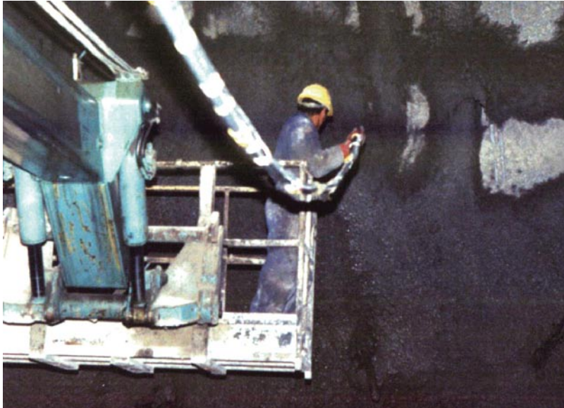
Fig. 3.4 Installation of a sliding micrometer to measure core-face extrusion
