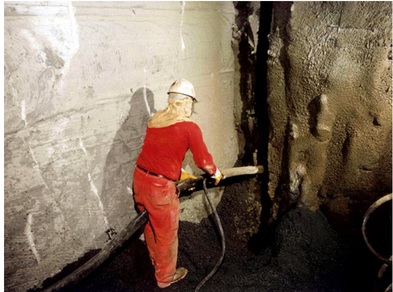
Cavity preconfinement by means of full face mechanical precutting: manual filling of the precut with shotcrete (tunnels on the high speed/high capacity Milan-Rome-Naples railway line between South Arezzo and Figline Valdarno, 1988, ground: sandy silt, max. overburden: ~ 90 m)
