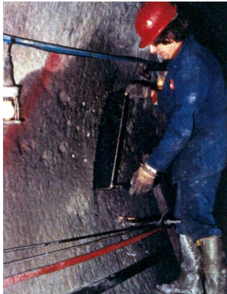
Placing of a flat jack
