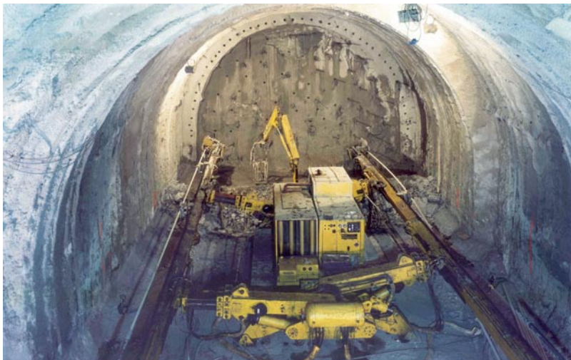
Fig. 2.17 Reinforcement of the core-face (Vasto Tunnel)
