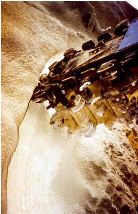
Pretunnel: details of the cutter head
