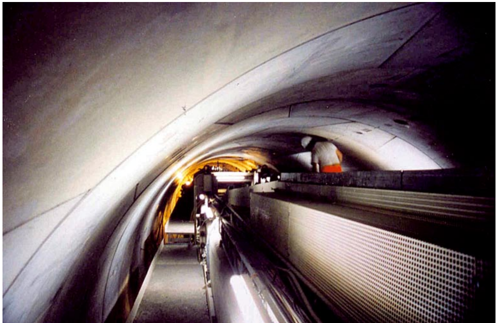
Ginori service tunnel: the "tail" of the TBM inside the tunnel already lined
