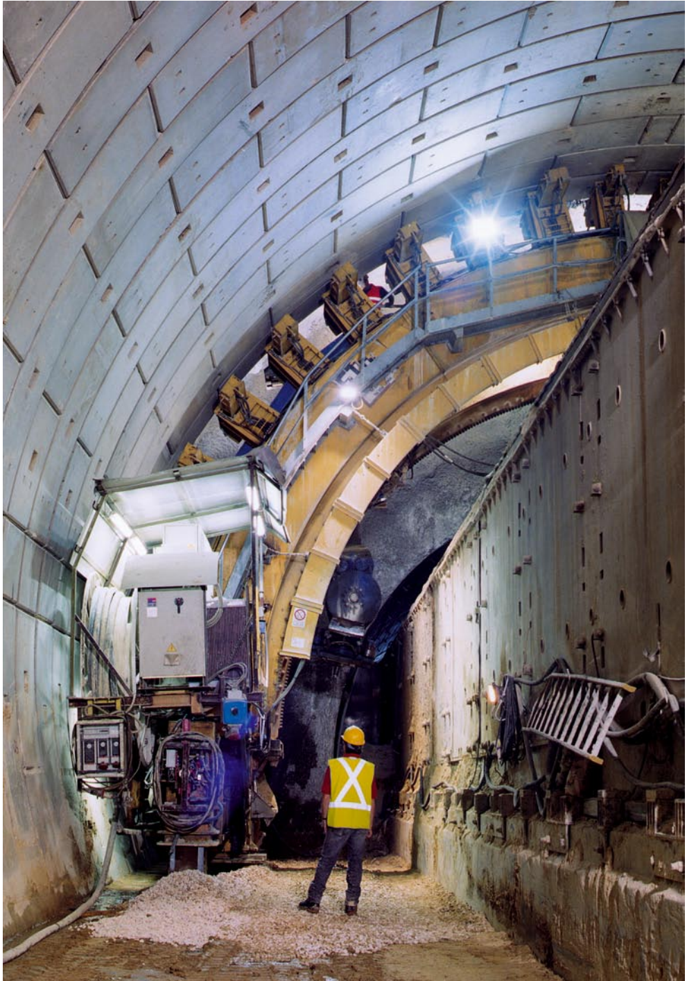
Widening of tunnels without interrupting traffic: Milan-Rome motorway, Nazzano tunnel, placing an arch of the lining constructed using prefabricated segments (2005)
