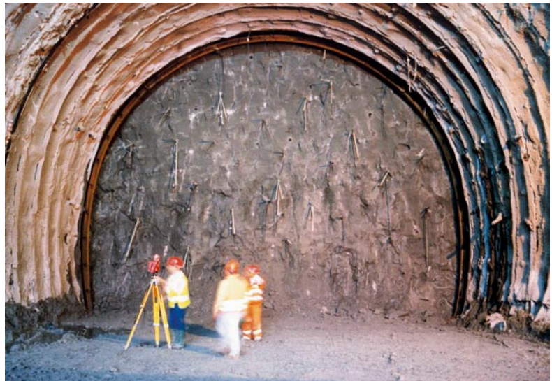
Fig. 6 Pianoro Tunnel (new high speed Milan-Rome-Naples railway line between Bologna and Florence, 1999, ground: cemented silty sand, overburden: 150 m, diameter: 13.30 m). View of the face reinforced with fibre glass structural elements
