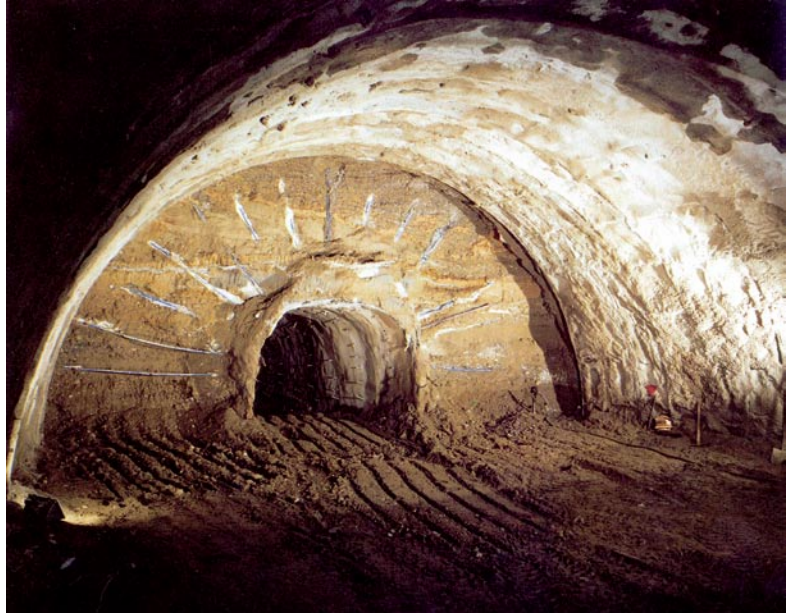
Cavity preconfinement by means of ground improved by radial injections: the effect of treatment performed from a central pilot tunnel (Line 3 of the Milan metro, 1985, ground: sand and gravels, overburden: 20 m)
