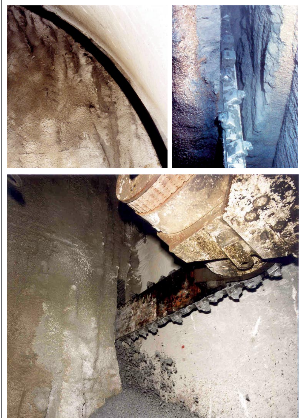
Cavity preconfinement by means of full face mechanical precutting: close-ups of operations (tunnels on the high speed/high capacity Milan-Rome-Naples railway line between South Arezzo and Figline Valdarno, 1988, ground: clayey silt, max. overburden: ~90 m)
