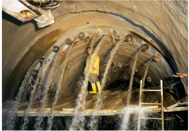
Cavity preconfinement by means of truncated cone 'umbrellas' of drainage pipes ahead of the face (Sibari-Cosenza railway line, tunnel 4, 1998, ground: silty sand, overburden: ~ 40 m)
