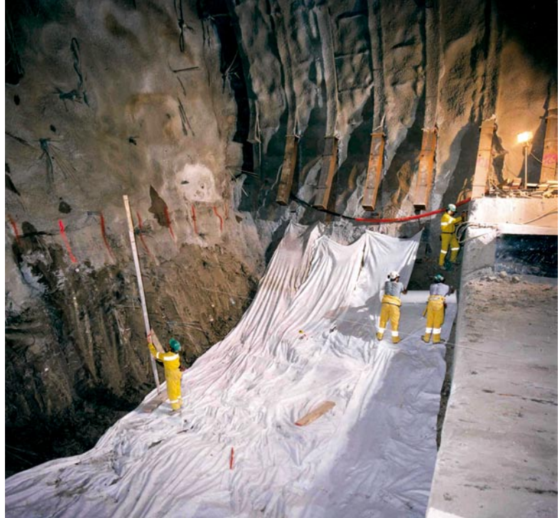
Cavity confinement by means of a tunnel invert: laying of the waterproofing for the tunnel invert (TGV Méditerranée, Lyon-Marseille railway line, Tartaignille tunnel, 1997, ground: clay, max. overburden: ~ 110 m)
