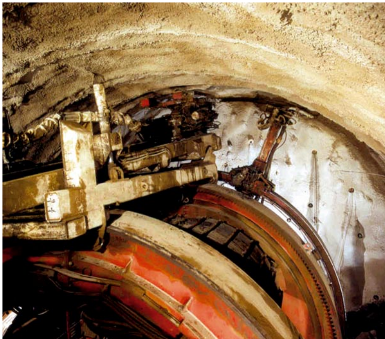
Cavity preconfinement by means of full face mechanical precutting: execution and filling of the precut (tunnels on the high speed/high capacity Milan-Rome-Naples railway line between South Arezzo and Figline Valdarno, 1988, ground: clayey silt, max. overburden: ~ 90 m)
