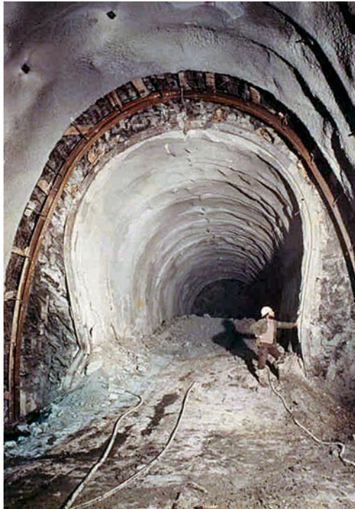
Convergence of the walls of a tunnel in plasticised rings or bands
