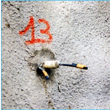
Fig. 9.17 Detail of fibre glass reinforcement injected with cement grout
