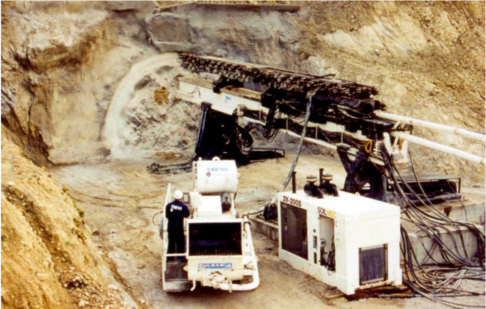
Pretunnel: experimentation on a test site (1996)
