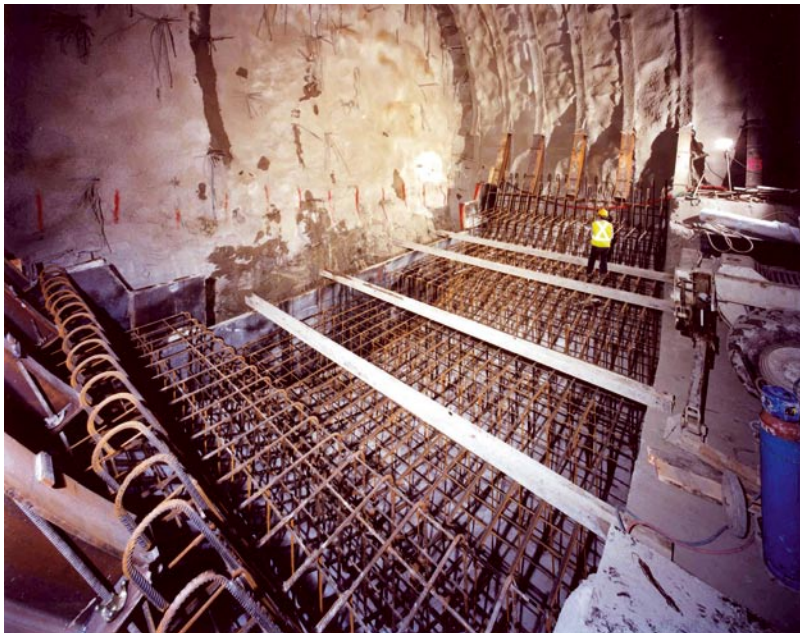
Fig. 9.39 Reinforcement for the tunnel invert (Tartaiguille tunnel)
