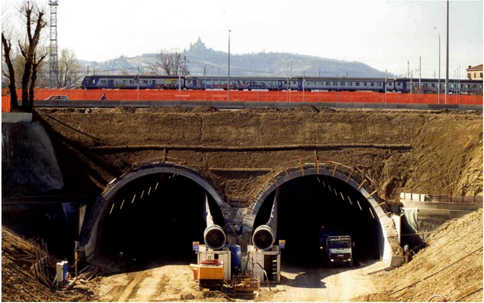
Cavity preconfinement by means of truncated cone 'umbrellas' consisting of sub horizontal columns of ground, side by side, improved by jet-grouting: portal of the double bore underpass of the Ravone railway yard in Bologna (2000, ground: silty sand and gravel in a sandy-silty matrix, overburden: ~ 7 m)
