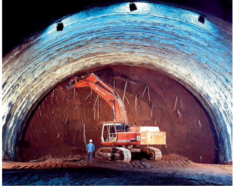
Excavation: mechanical excavation of the core-face using a ripper (Rome motorway ring road, Appia Antica tunnel, 1999, ground: granular pyroclastites, overburden: ~ 4 m)
