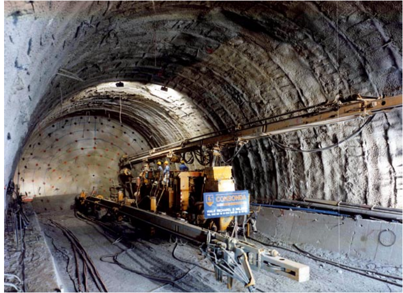
Cavity preconfinement after reinforcement of the core-face with fibre glass reinforcement: drilling for insertion of the reinforcement (Caserta-Foggia railway line, S. Vitale tunnel, 1993, ground: scaly clay, overburden: ~ 130 m)
