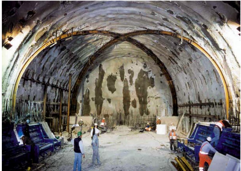
S. Giorgio access tunnel. Construction of the junction with the Firenzuola running tunnel (ground: Clays of the Mugello Basin, overburden: ~ 30 m)
