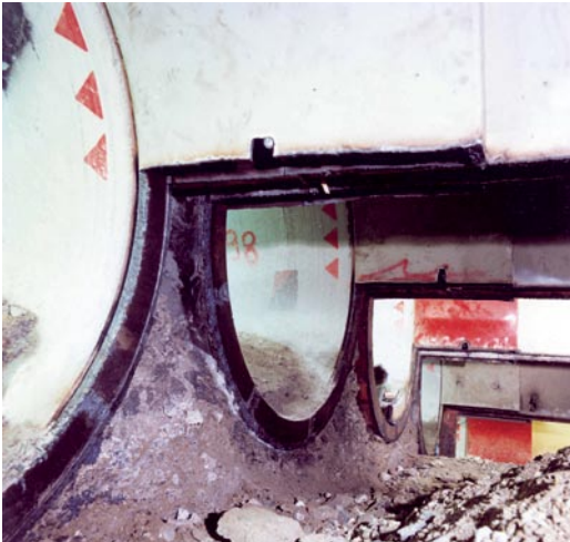
Venezia Station on the Milan urban link railway line: the cut of the pipes (minitunnels) for creating the transverse arches
