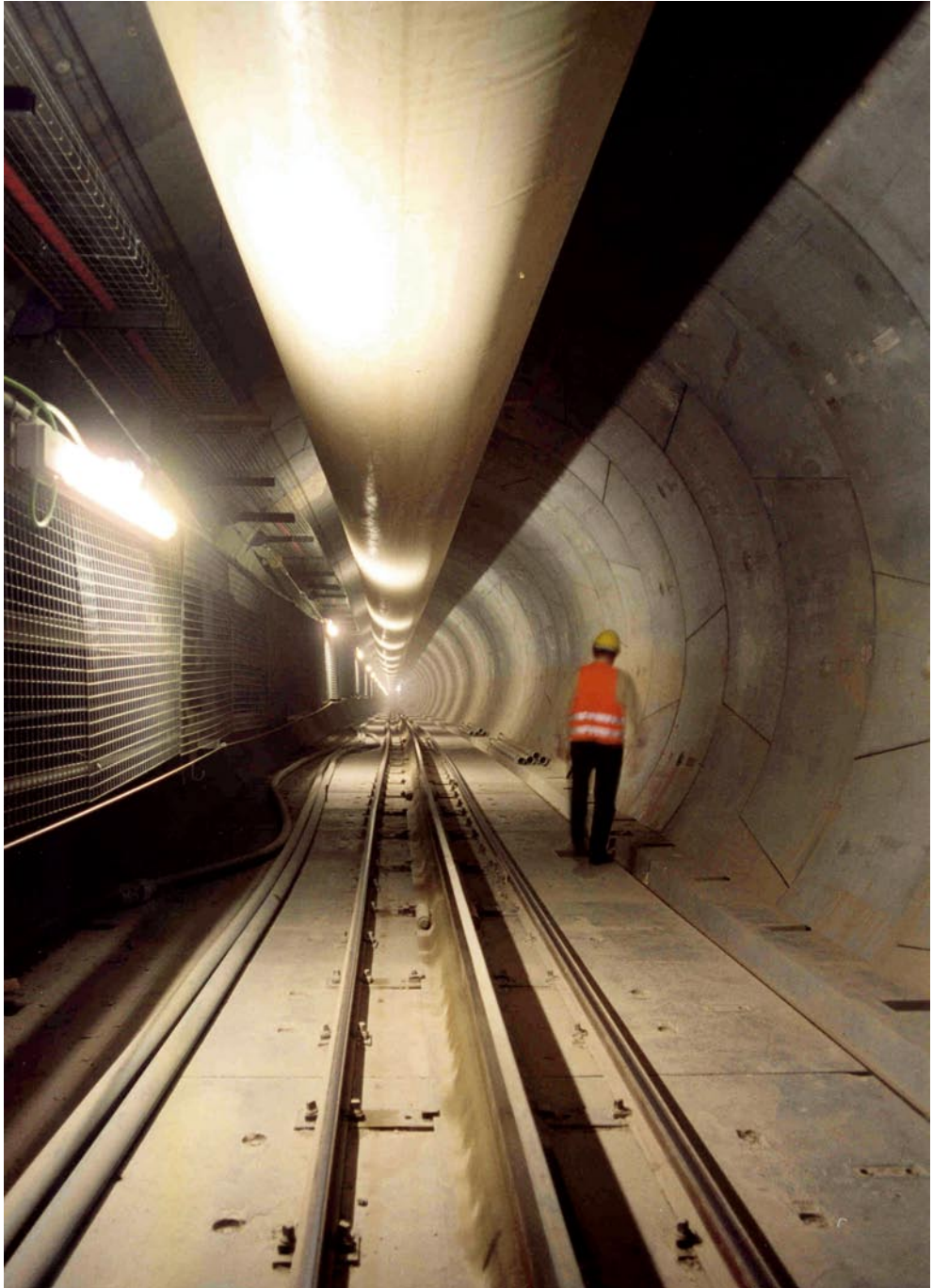
Cavity confinement by means of a final lining: final lining of prefabricated segments in RC (high speed/high capacity railway line between Bologna and Florence, Ginori service tunnel, 2001, ground: limestones and marls, max. overburden: ~ 600 m)
