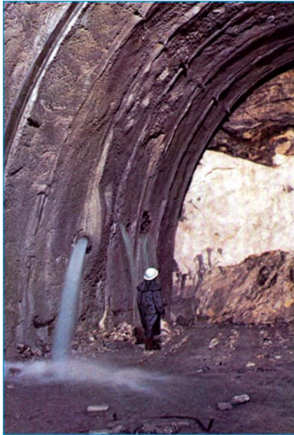
Fig. 9.29 Advance through an aquifer under 60 bar of hydraulic pressure (Gran Sasso motorway tunnel)
