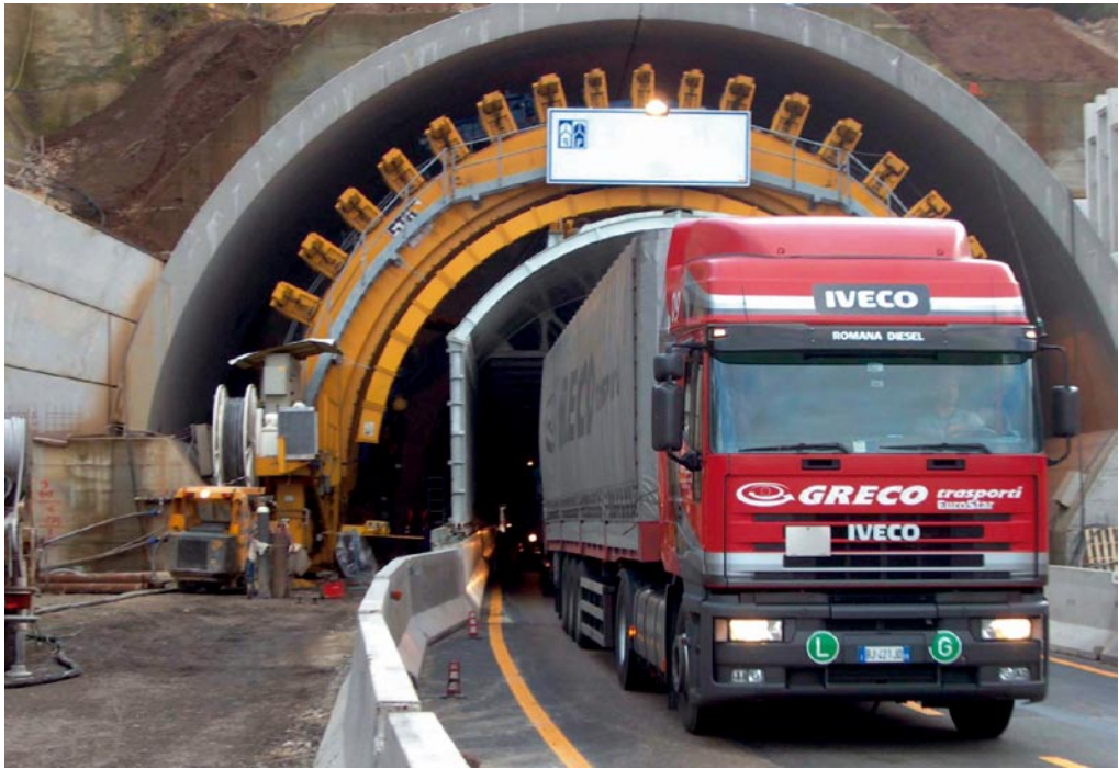
Fig. G.13 The work to widen the tunnel was performed with the motorway in service
