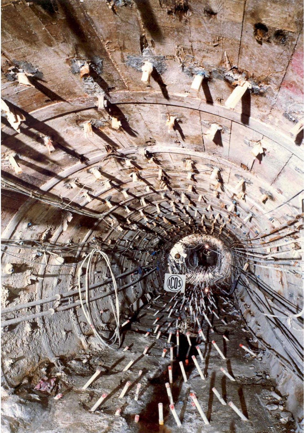
Cavity preconfinement by means of ground improved by conventional grout injections: treatment from a central pilot tunnel (Milan urban railway link line)
