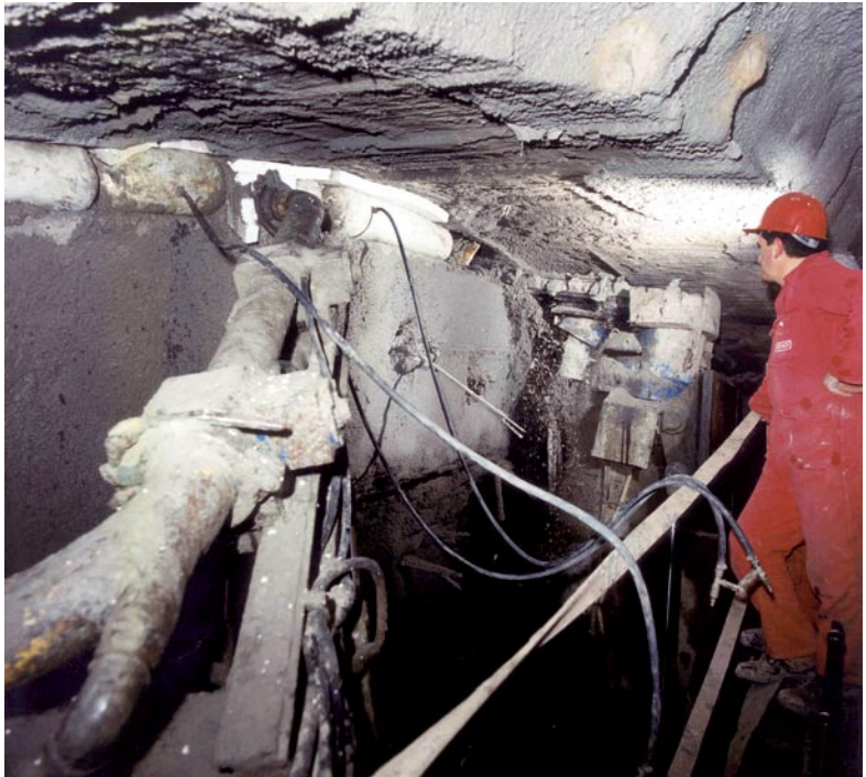
Cavity preconfinement by means of full face mechanical precutting: execution and filling of the 21.5 m span precut with pumped concrete confined using pneumatic formwork (line A of the Rome metro, Baldo degli Ubaldi Station, 1996, ground: clay with sand strata, overburden: ~ 18 m)
