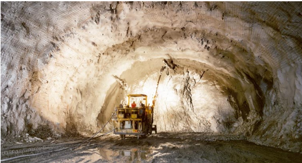
Band of reinforced ground around the cavity (cavern for the Brunico sewage plant)
