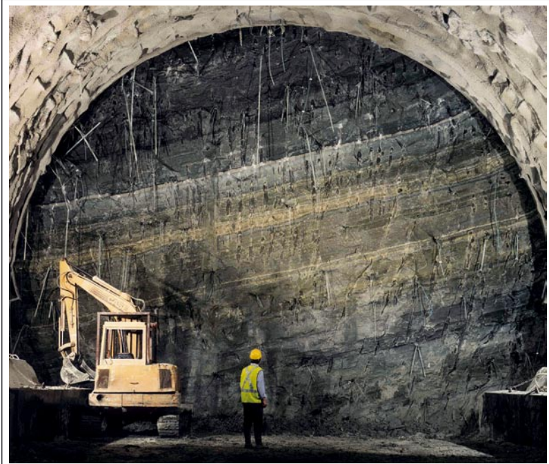
Fig. 5 Tartaignille tunnel (France, TGV Méditerranée, Lyon-Marseilles railway line, 1998, ground: Swelling clay [75% montmorillonite], overburden: 100 m, diameter: 15 m). View of the face ( 180\text{ m}^2 cross section) reinforced with fibre glass structural elements
