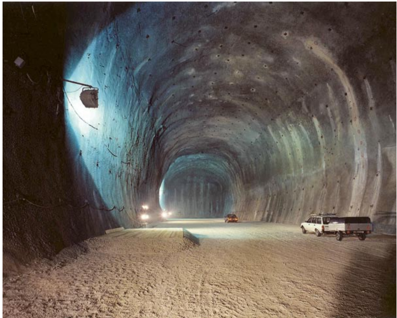
Confinement of the cavity by means of radial rock bolts: cavern-laboratory C, stabilised using fully bonded rock bolts and shotcrete (INFN laboratory of the Gran Sasso, 1984, ground: limestones, overburden: ~ 1400 m)
