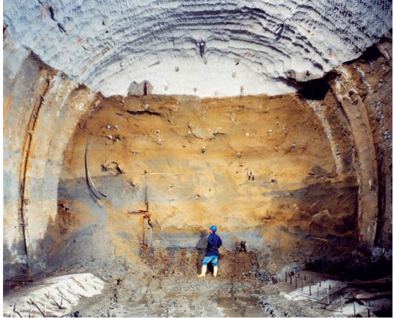
Cavity preconfinement by means of truncated cone 'umbrellas' of ground improved by conventional grout injections (Sibari-Cosenza railway line, tunnel 4, 1998, ground: silty sand, overburden: ~ 40 m)
