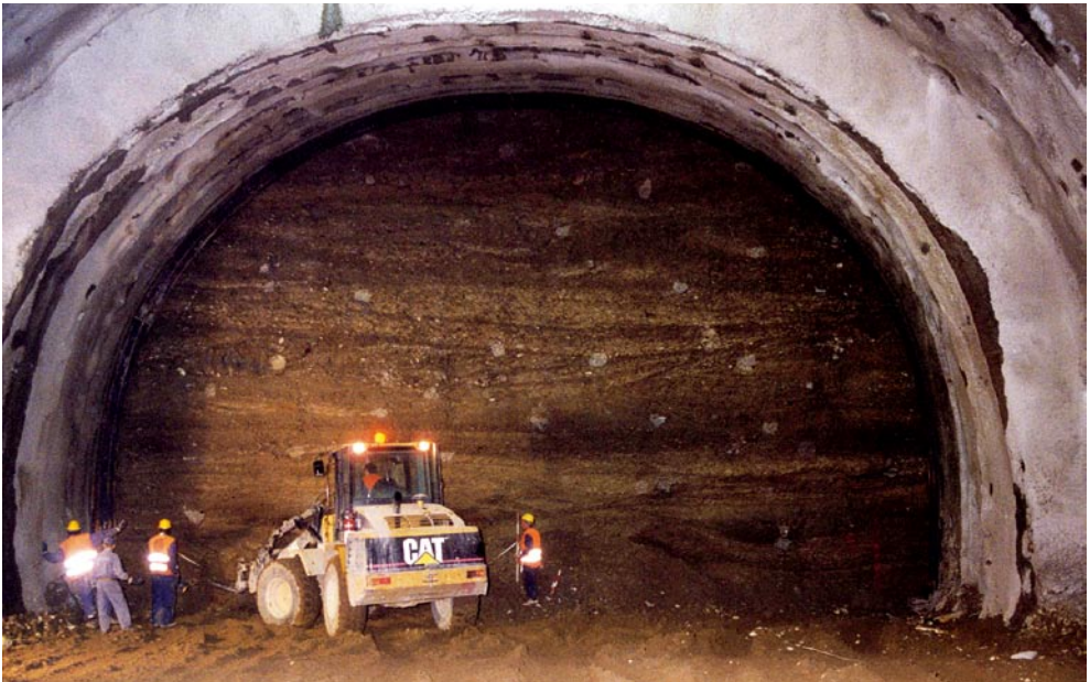
Cavity preconfinement by means of truncated cone 'umbrellas' consisting of sub horizontal columns of ground, side by side, improved by jet-grouting: view of the reinforced core-face (underpass of the Ravone railway yard in Bologna, 2000, ground: silty sand and gravel in a sandy-silty matrix, overburden: ~ 7 m)
