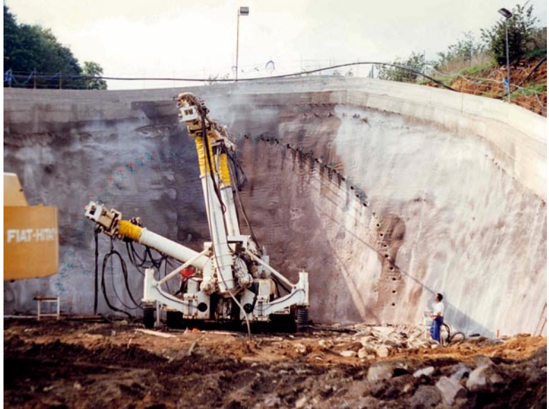
Colli Albani Tunnel. Horizontal jet-grouting to improve the ground for the South portal
