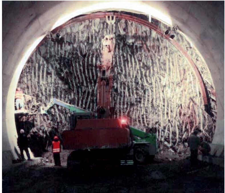
Colle Pece Tunnel. Positioning a steel rib. Ground: scaly clays, overburden: 25 m
