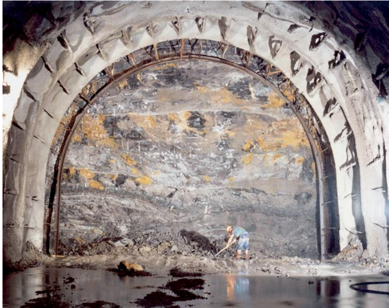
Fig. 5.2 Two examples of tunnels with stable core-face deformation behaviour. Top: S. Rocco Tunnel (Rome-L'Aquila motorway) 1967, ground: limestone, overburden ~ 400 m. Bottom: S. Stefano Tunnel (Genoa-Ventimiglia railway), 1984, ground: marly-sandy argillite flysch, overburden ~ 100 m
