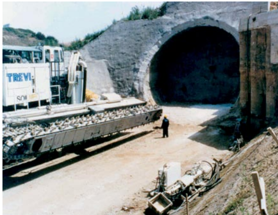
Pretunnel: the start of excavation (Castello 1 tunnel, high speed/high capacity Rome-Naples railway, 1996, ground: cineritic tuff, max. overburden: 9 m)
