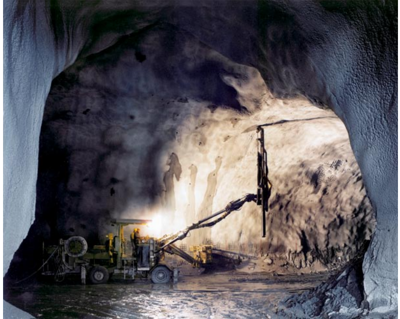
Confinement of the cavity by means of radial rock bolts: placing of a rock bolt (purifier in a cavern at Brunico, 1993, ground: quartziferous phyllites, max. overburden: ~ 125 m)
