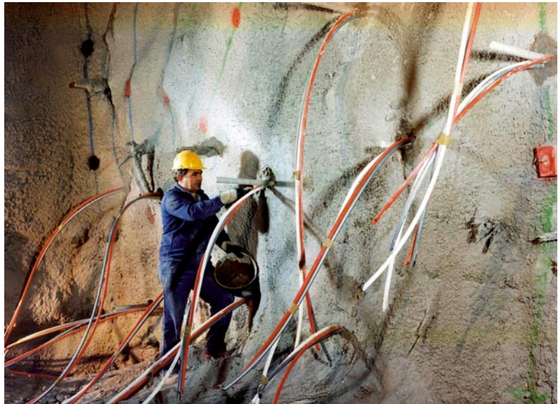
Cavity preconfinement after reinforcement of the core-face with fibre glass reinforcement: caulking with rapid setting cement before injection (Caserta-Foggia railway line, S. Vitale tunnel, 1993, ground: scaly clay, overburden: ~130 m)
