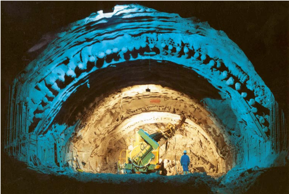
Presupport intervention with forepoles (Solignano tunnel)
