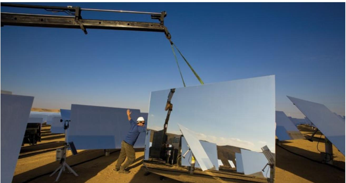
Construction workers installing heliostats at a Brightsource solar thermal power tower<sup>41</sup>
