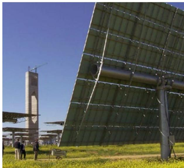
121 m<sup>2</sup> heliostat at Abengoa PS10 power tower, Spain<sup>11</sup>
