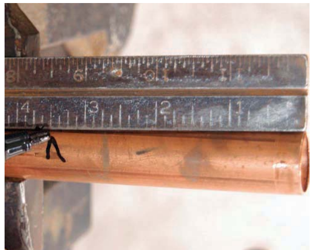
FIGURE 20-20 Measuring and marking the length of copper pipe. Larry Jeffus
