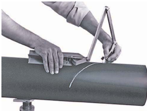
FIGURE 6-35 Pipe being laid out using a contour marker. Larry Jeffus
