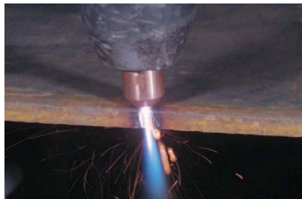
FIGURE 22-30 When the plasma cut begins, move the torch at a constant speed down the plate. Larry Jeffus
