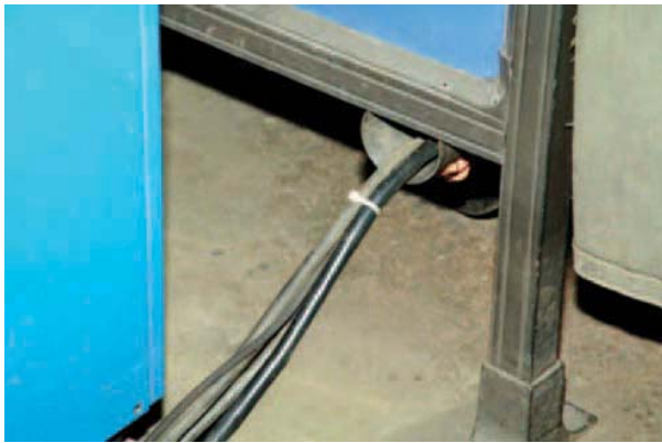
FIGURE 15-9 A bracket holds the leads off the floor. Larry Jeffus
