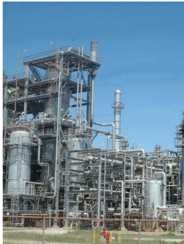
FIGURE 1-9 An oil refinery is an example of a structure that requires critical welds to ensure its safe operation.
