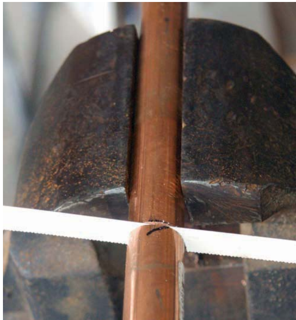
FIGURE 20-21 Cutting the copper pipe to length. Larry Jeffus
