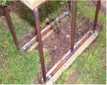
CLAMP ARCH PIPE TO BASE
