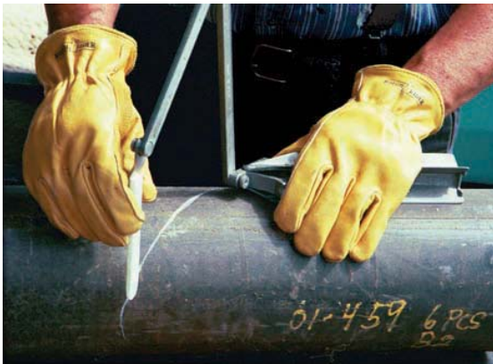
FIGURE 10-42 Laying out a 45° angle on a pipe using a Curv-O-Mark® tool. Larry Jeffus
