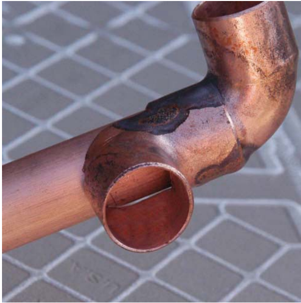
FIGURE 20-64C Check to see that the fitting is clean. Larry Jeffus
