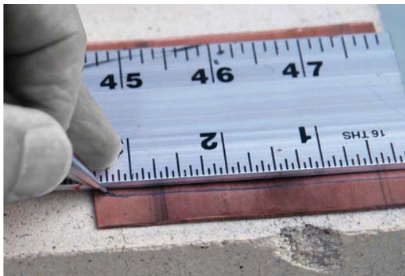
FIGURE 20-26 Draw a line to be cut. Larry Jeffus
