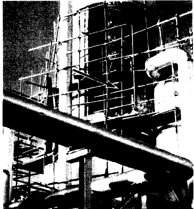
Figure 9.6—Stripper lowers with One of Six Equal Shell Sections Removed
