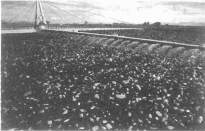
Figure 9-11. Trickling filter.
