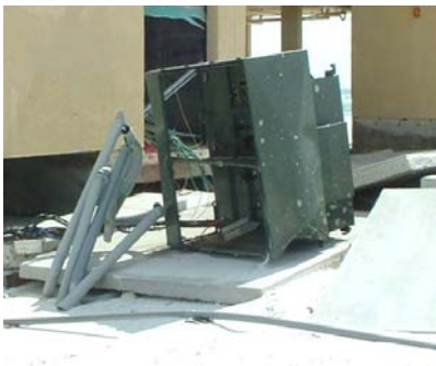
Figure 3.14. This figure shows images of hurricane damage to distribution system: (upper left) overhead line damage in a coastal area; (upper right) substation flooding; (lower left) a padmount transformer damaged from storm surge; (lower right) a concrete pole broken during a hurricane.
