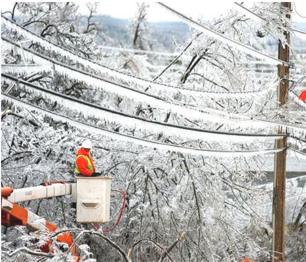
Figure 3.18. Ice buildup on trees, conductors, and third-party attachments. This weight of this ice can break tree branches, tree trunks, crossarms, conductors, and poles. The ice also increases susceptibility to wind damage due to increased surface area.
