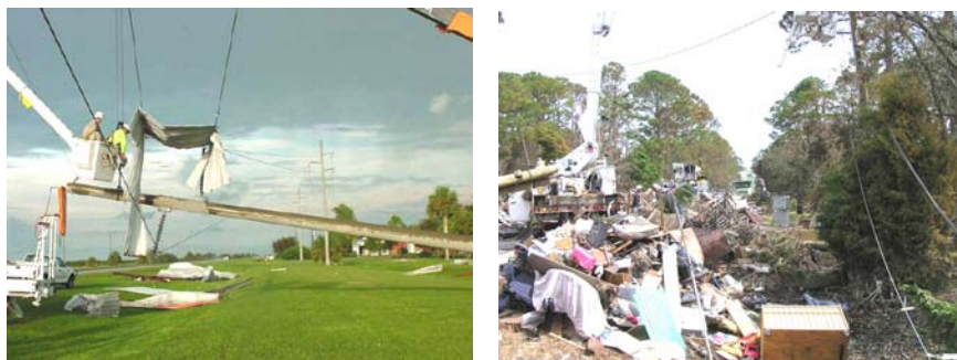
Figure 3.15. Debris is a major hurricane concern. The left image shows a corrugated steel roof that flew into power lines. The right image shows a pile of debris that may be covering undamaged pad-mounted equipment. When bulldozers clear this pile, the pad-mounted equipment is vulnerable to damage.
