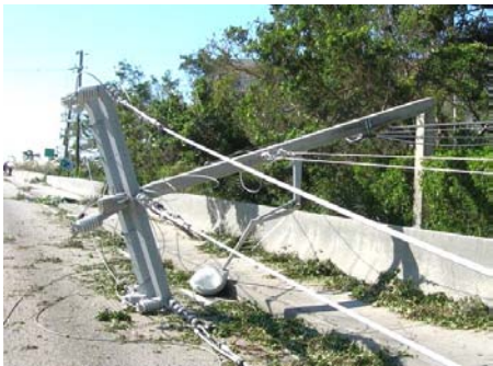
Figure 3.14. This figure shows images of hurricane damage to distribution system: (upper left) overhead line damage in a coastal area; (upper right) substation flooding; (lower left) a padmount transformer damaged from storm surge; (lower right) a concrete pole broken during a hurricane.
