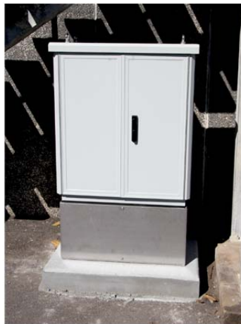
Figure 12 – FDA – Fibre distribution ancillary panel
