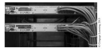
Figure 20–23b Ethernet Switches
