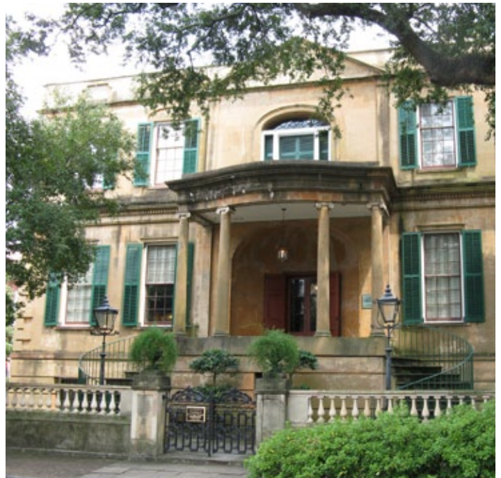
The Owens-Thomas House is a prominent feature of Oglethorpe Square, designed by renowned architect William Jay. It is the only trust lot residence that retains its original yard and outbuildings.
