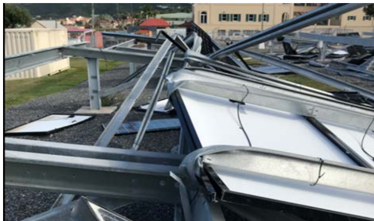
Figure 10. It might be the responsibility of the O&M provider to respond and ensure that storm damage is rendered safe both in terms of electrical hazards and loose components following an extreme weather event such as this damage in St. Croix in 2017. Photo by Andy Walker, NREL
