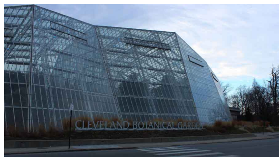
Emergency Power Setup Crucial for Cleveland Arboretum and Gardens
