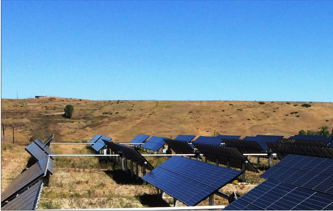
Figure 6. Although improving annual energy delivery, especially in summer, tracking mechanisms and controls require regular maintenance to be effective. Photo by Andy Walker, NREL
