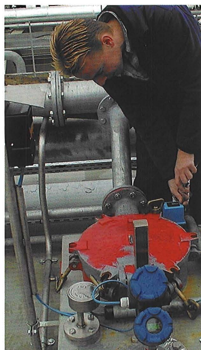
Testing cargo tank alarms
