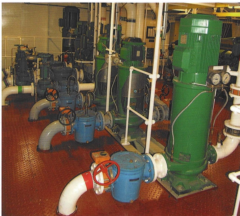
Engine room with IP 44 and higher motors
