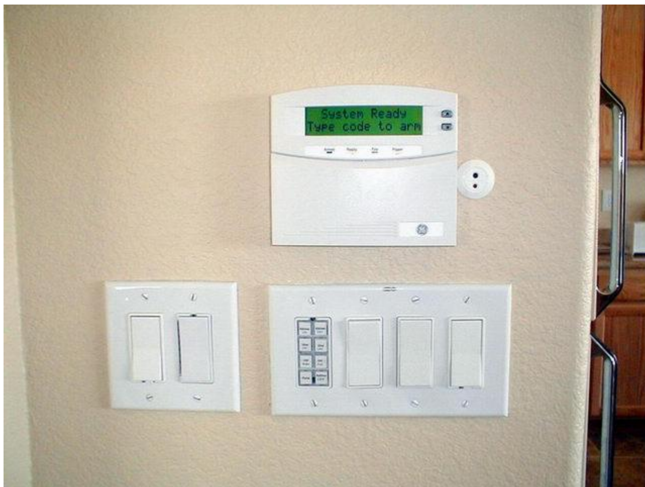
LCD Keypad, and (round) Glass Break Sensor
