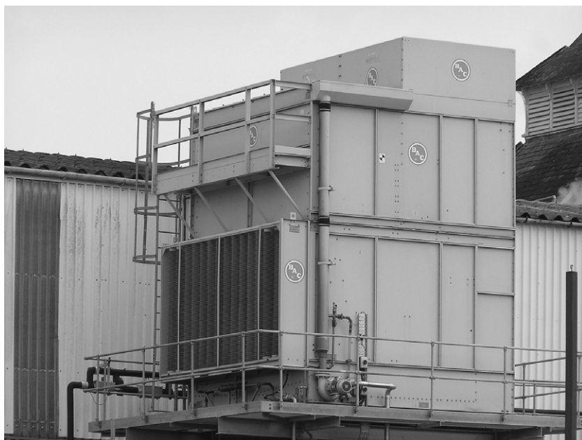
Figure 6.8 Evaporative condenser installation (Baltimore Aircoil)
