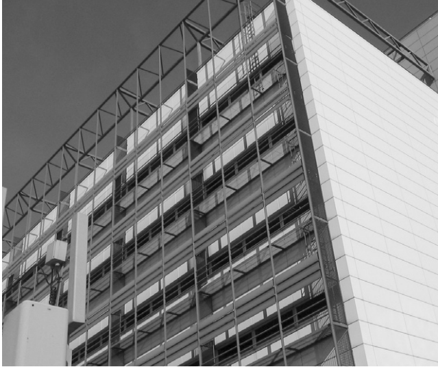
Figure 23.2 Solar shading (Business Edge)
