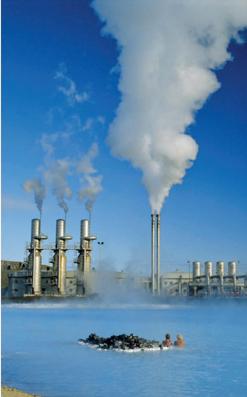
Discharged salt, algae, and silica-rich water from the Svartsengi Geothermal Power Plant in Iceland formed the famed Blue Lagoon.
