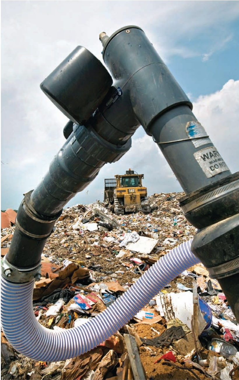
Methane gas is collected from wells at this Michigan landfill and then used to generate electricity.
