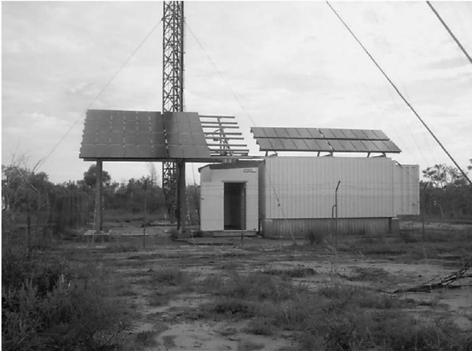
Figure 8.2. The first solar-powered mobile telephony base station in the Telstra network, located at Roebuck plains, Western Australia, (Used with permission of Silcar Pty Ltd. Design & Construction)
