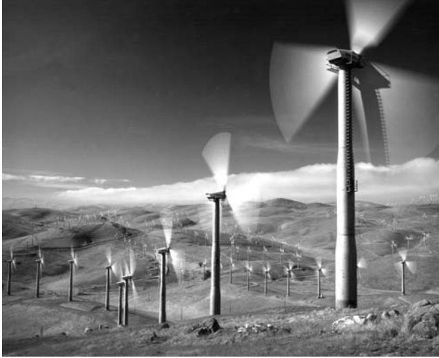
Figure 1.3 Example of a large wind farm of >100 WTs in California in the early 1980s
