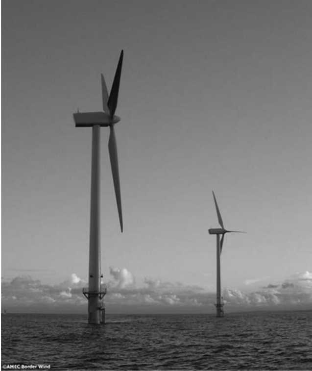
Figure 1.5 The first offshore wind farm in UK at Blyth, 2 Vestas V66 HAWTs [Source: AMEC Border Wind]
