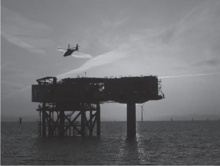
Figure 8.5 Example of substation installation at Horns Rev 2 [Source: Vattenfall]
