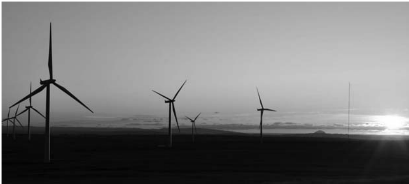
Figure 1.4 The largest wind farm in the United Kingdom at Whitelee near Glasgow with 140 Siemens 2.3 MW HAWTs
