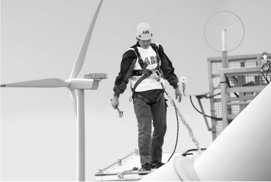
Figure 5.11 Offshore wind turbine commissioning [Source: ABB Drives]
