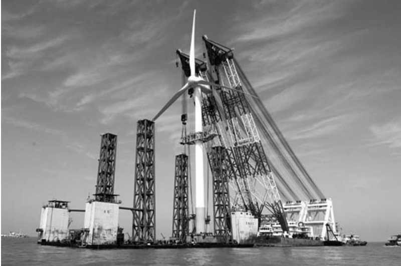
Figure 1.9 Installation of a 3 MW Sinovel WT at Dong Hai near Shanghai
