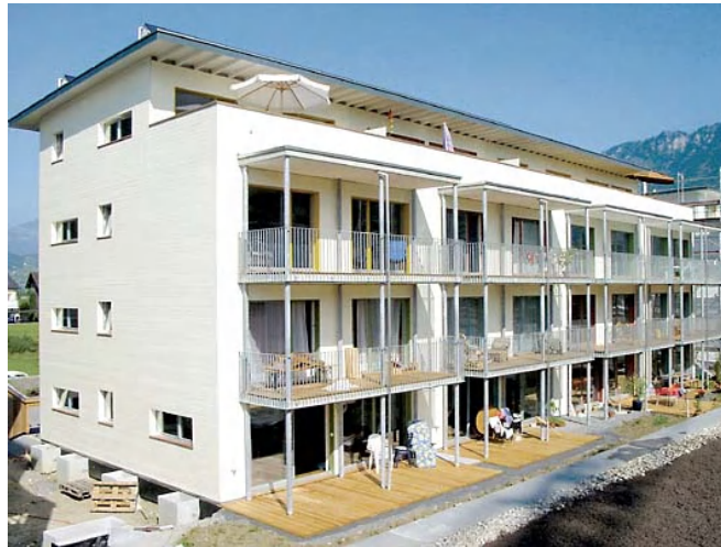
Figure 6.35. Wechsel Stans building in Switzerland
