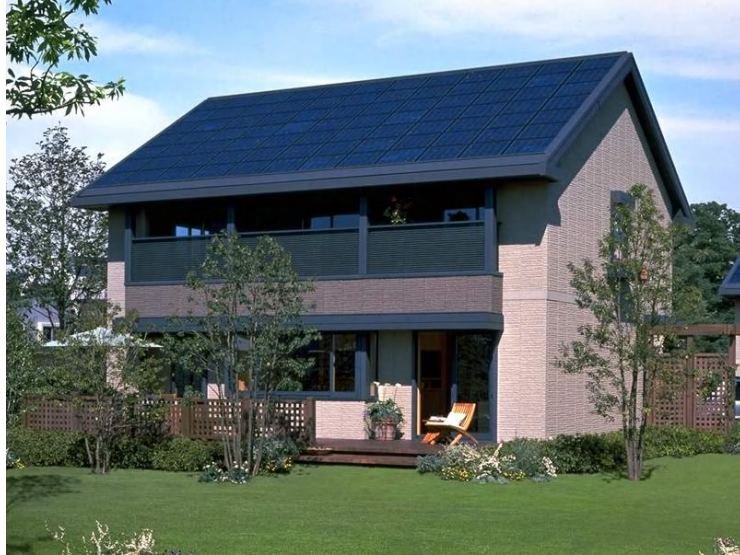
Figure 6.33. Zero-energy house from Misawa Home – Hybrid Z
