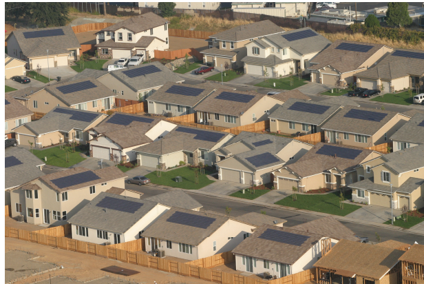
Figure 6.32. Premier ZEHs Premier Gardens, Sacramento, California (source: www.smud.org/residential/saving/zeroenergyhomes.html )
