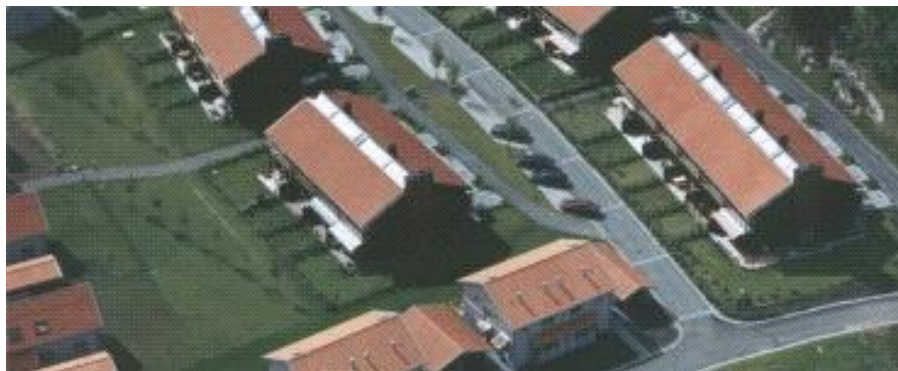
Figure 6.30. Houses without heating – Lindas, Sweden
