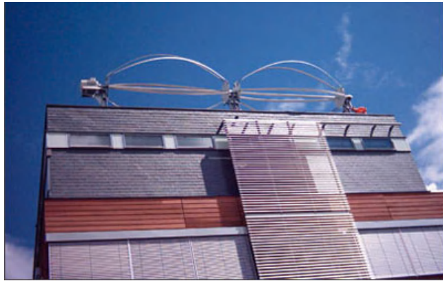
Figure 6.21. Horizontal shaft wind generator on a flat roof (source www.windwall.nl )
