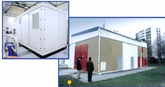
Figure 5.40. 200 electric kW and 220 thermic kW PAFC operating with natural gas. First cell installed by EdF-GdF at Chelles (Seine et Marne – France) in March 2000
