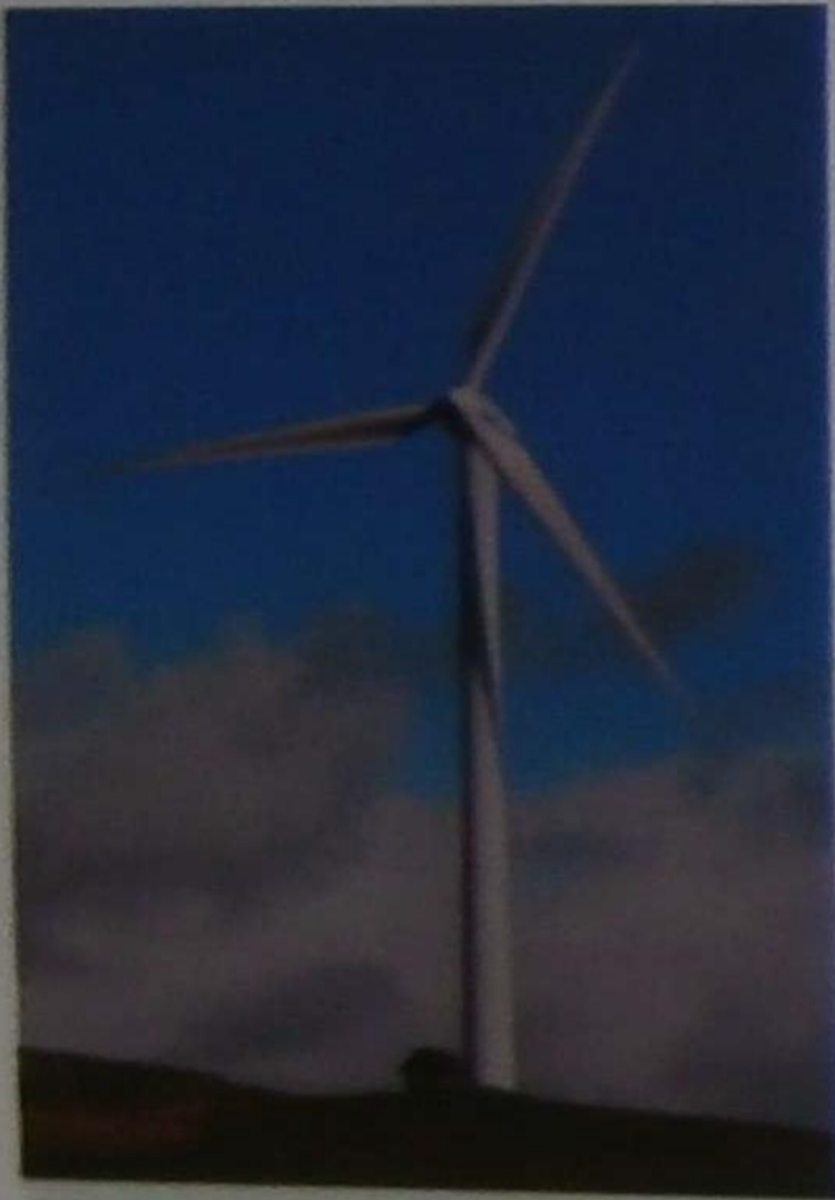
Figure 7.13 Three-bladed HAWT (Vestas V52 850 kW turbine)
