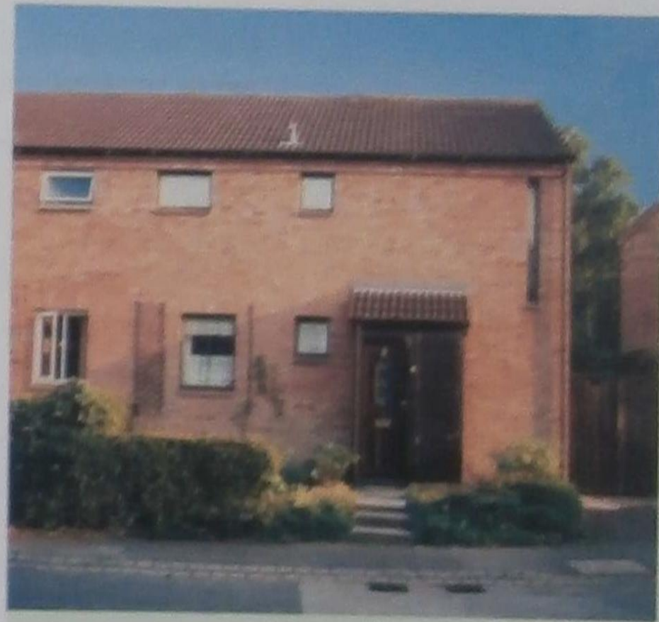
Figure 2.35 Passive solar housing at Pennyland – the north side has smaller windows
