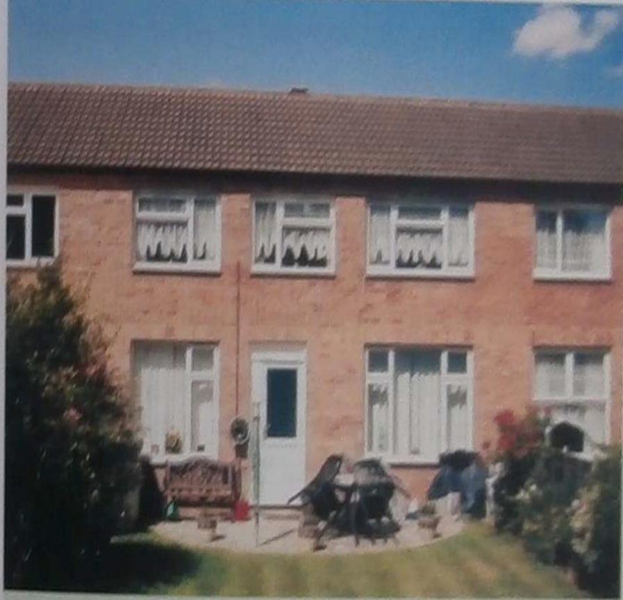
Figure 2.34 Passive solar housing at Pennyland – south elevation – the main living rooms have large windows and face south
