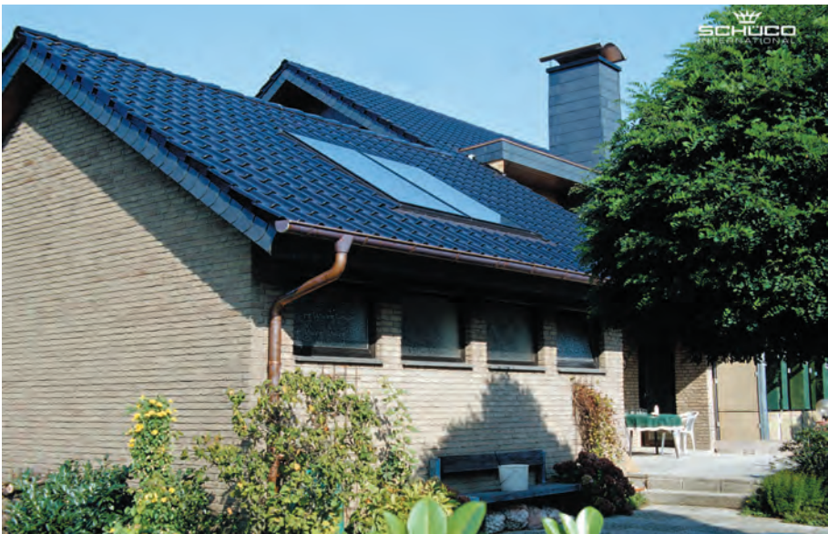
Figure 4.27. Example of in-roof installation. Source: Schüco, Bielefeld
