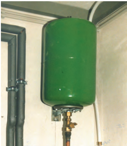
Figure 4.57 False expansion vessel connection from below
