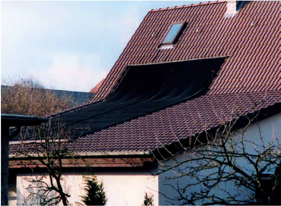
Figure 7.24. Private solar system for pool heating
