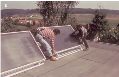
Figure 4.29c, d. Flat roof mounting Source: Wagner and Co., Cölbe
