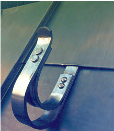
Figure 4.11. Left: roof hooks. Right: walk-on grating 30
