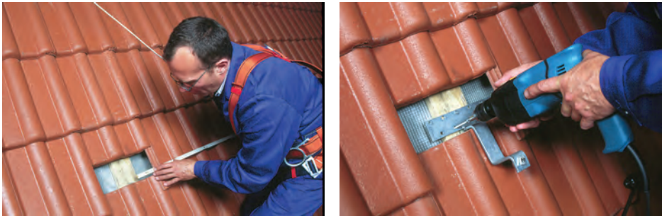
Figure 4.20. On-roof installation Source: Wagner and Co., Cölbe
