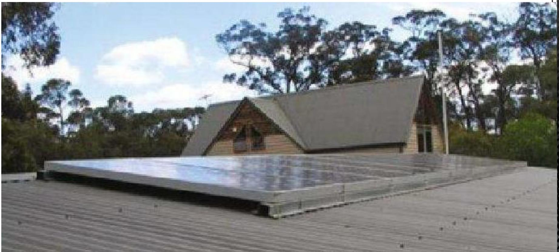
**Figure 6.2** This mounting scheme will not permit good airflow
