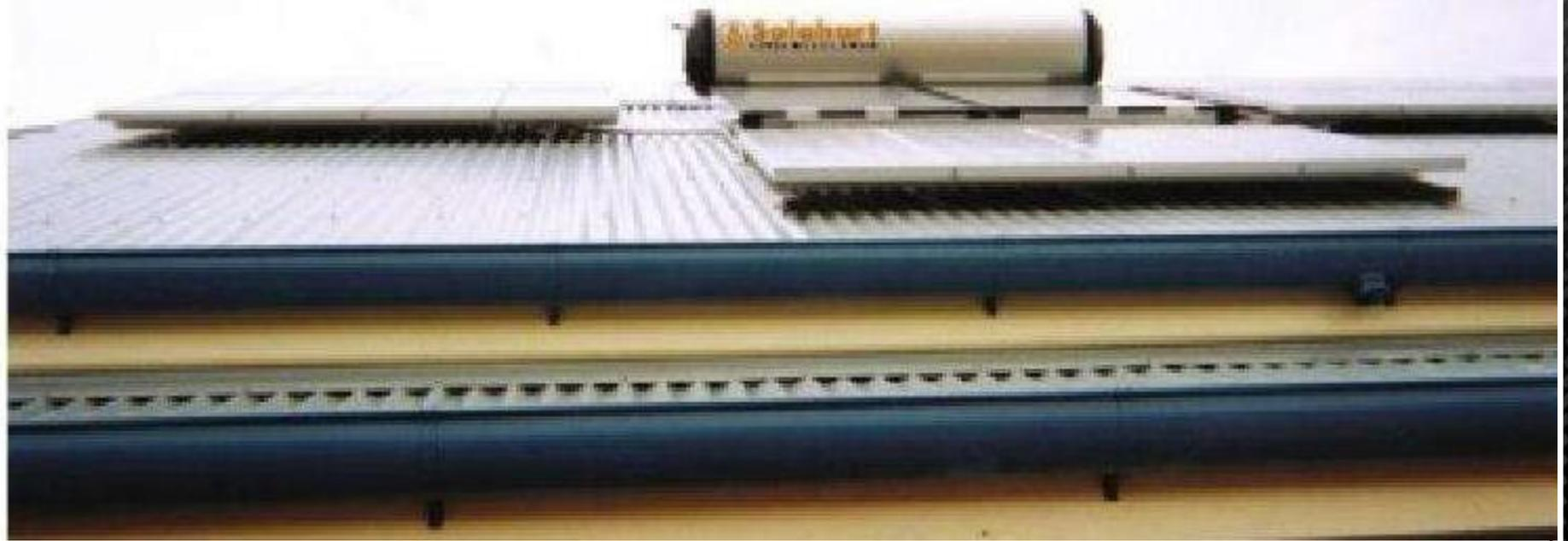
**Figure 6.1** This mounting scheme allows good ventilation. Mounting panels closer to the roof increases operating temperature and thereby lowers system performance
