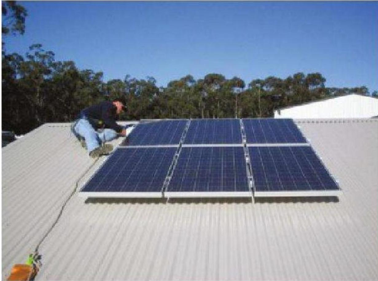
**Figure 10.6** An electrician installs a small white PV combiner box next to the array
