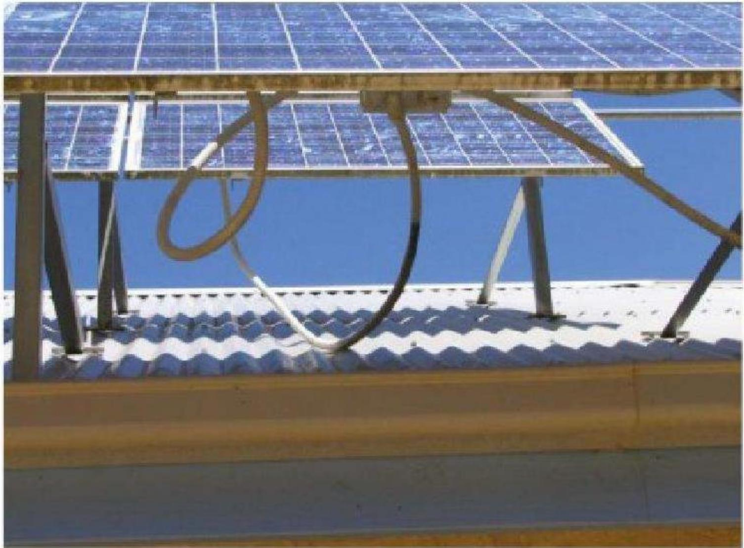
Figure 10.4 Photograph of a conductive loop
