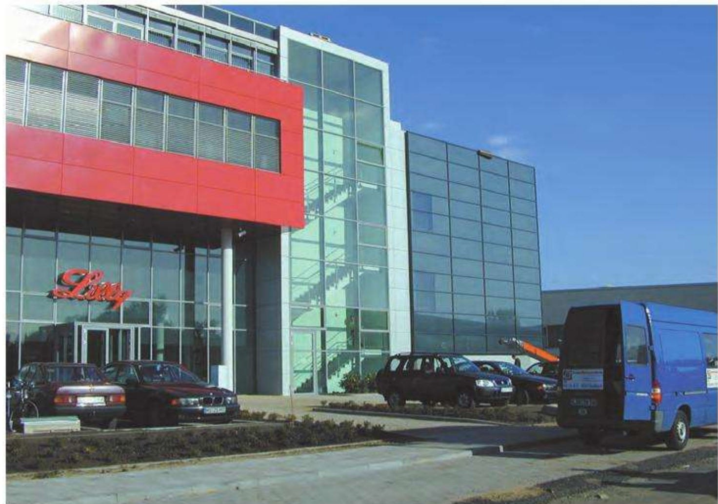
Figure 8.16. Solar air collector on the façade. Source: Grammer, Amberg
