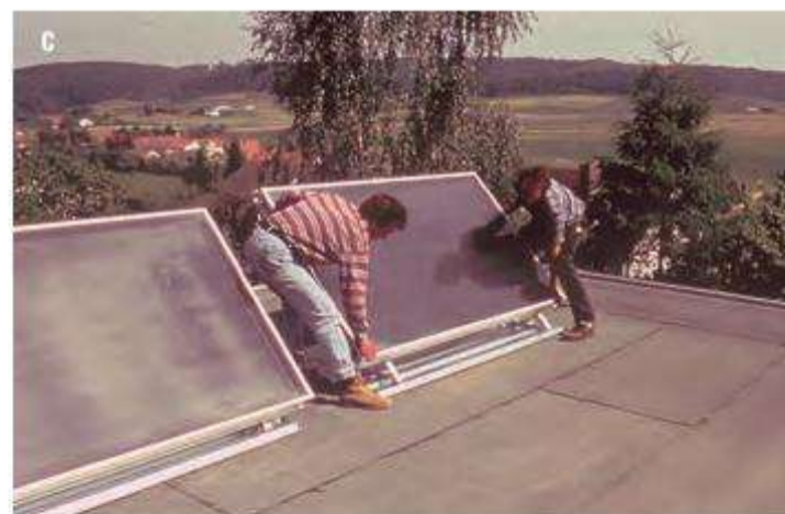
Figure 4.29c, d. Flat roof mounting Source: Wagner and Co., Cölbe
