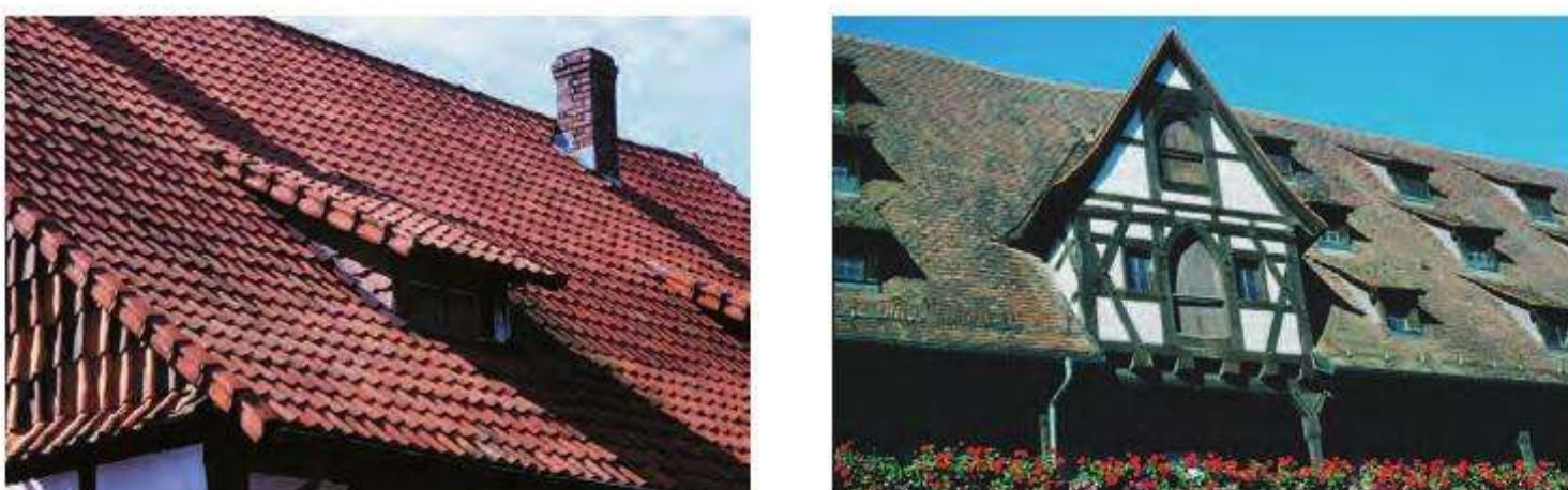
Figure 4.5. Left: pantiles. Right: wood shingles 27
