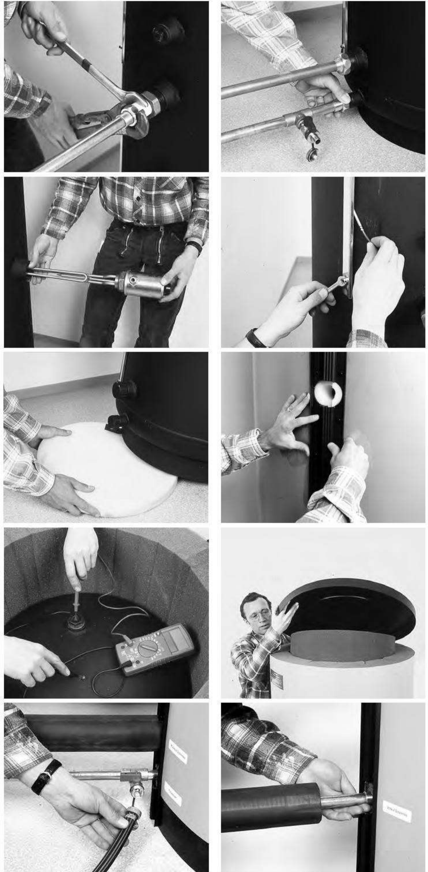
Figure 4.44. Connection and thermal insulation of a solar store Source: Wagner and Co., Cölbe
