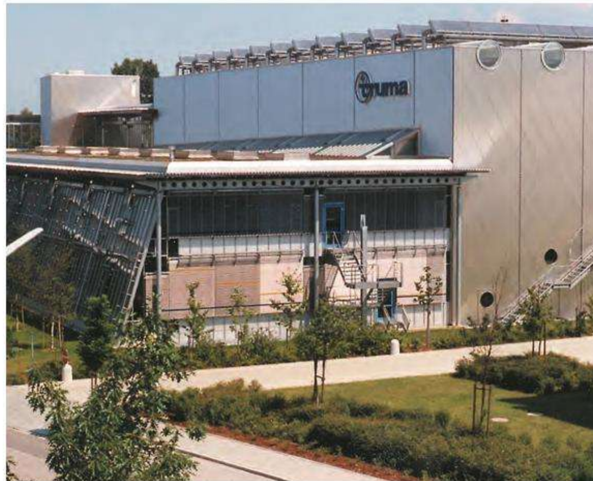
Figure 8.5. Air collectors placed on stands on the roof of a factory building. Source: Grammer, Amberg
