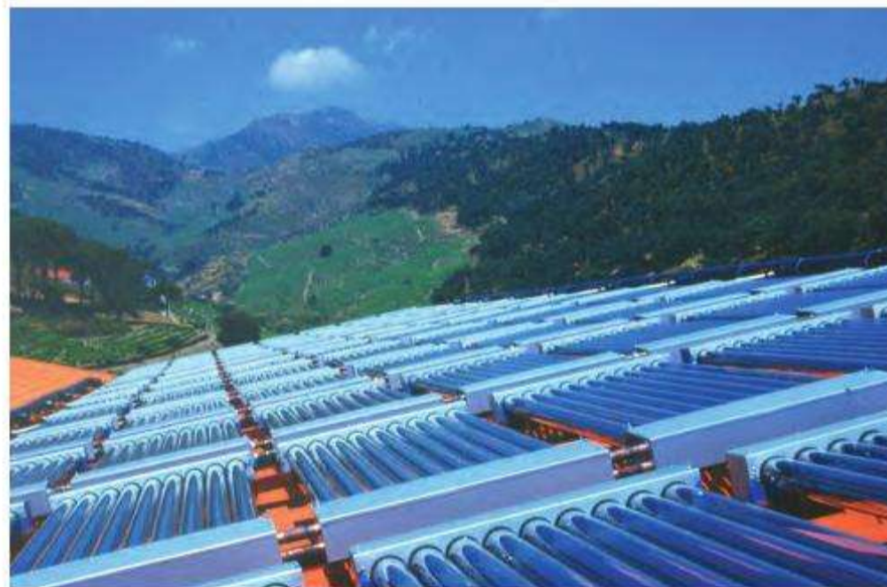
Figure 9.18. Solar absorption system for cooling of wine cellar in France
