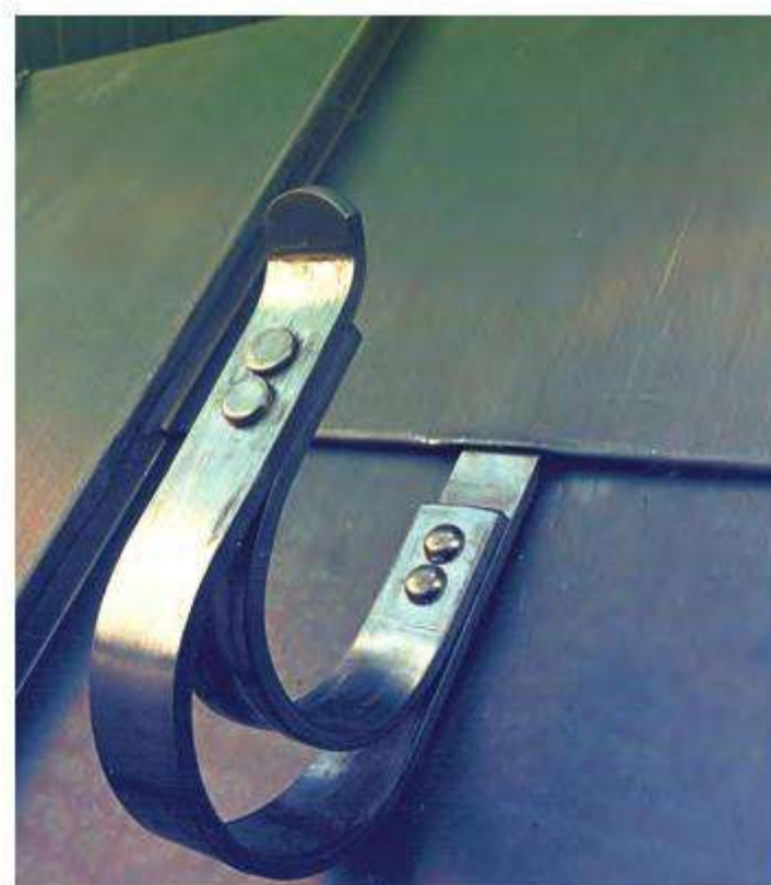
Figure 4.11. Left: roof hooks. Right: walk-on grating 30
