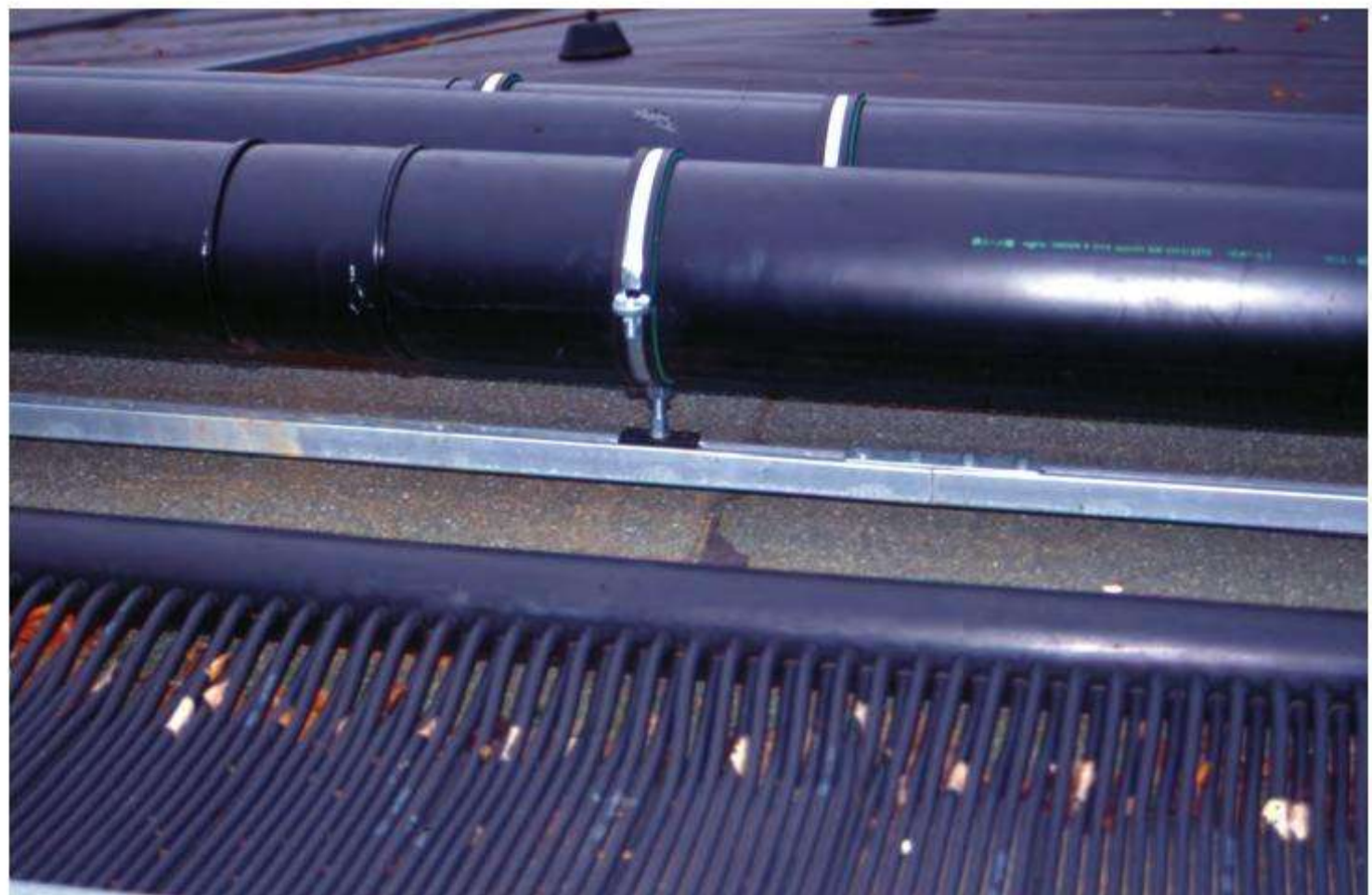
Figure 7.23. Example of sliding installation of pipe with anchor clamps
