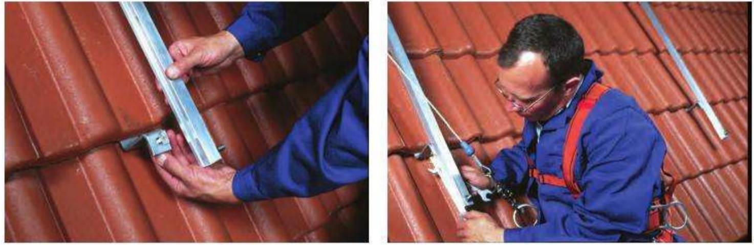
Figure 4.21. Example of on-roof installation Source: Wagner and Co., Cölbe
