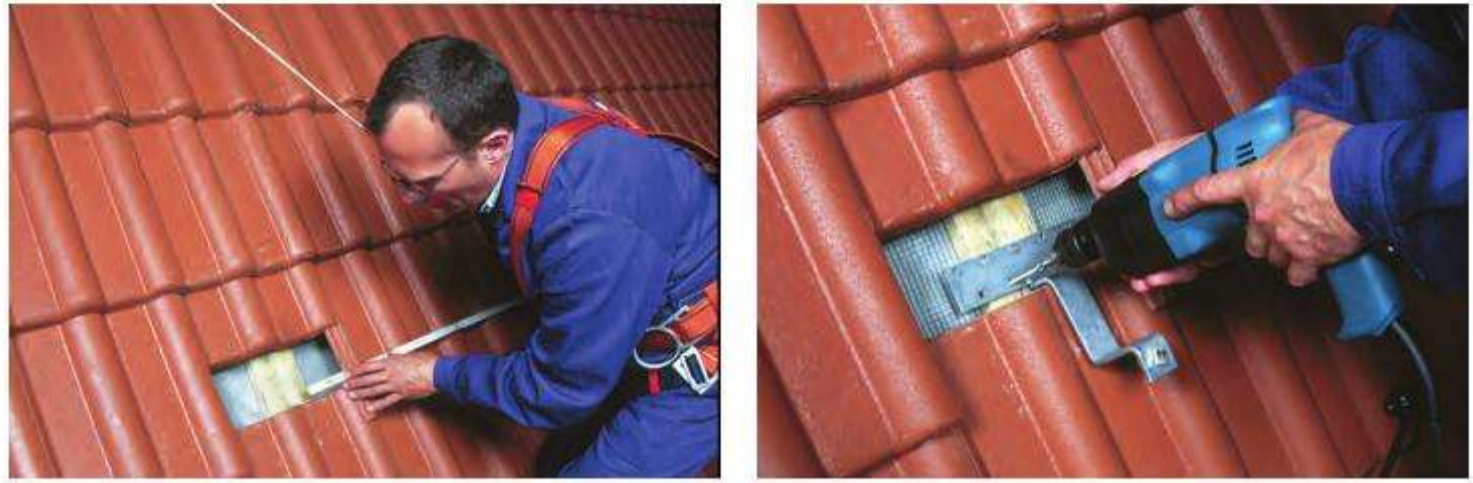
Figure 4.20. On-roof installation Source: Wagner and Co., Cölbe
