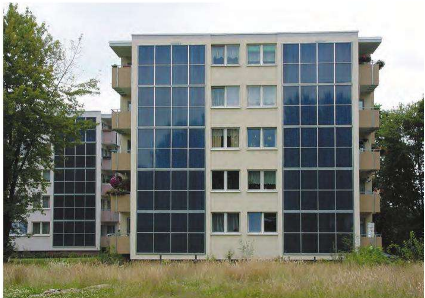
Figure 4.36. Façade installation of a large surface collector in Bielefeld. Source: Wagner & Co, Cölbe
