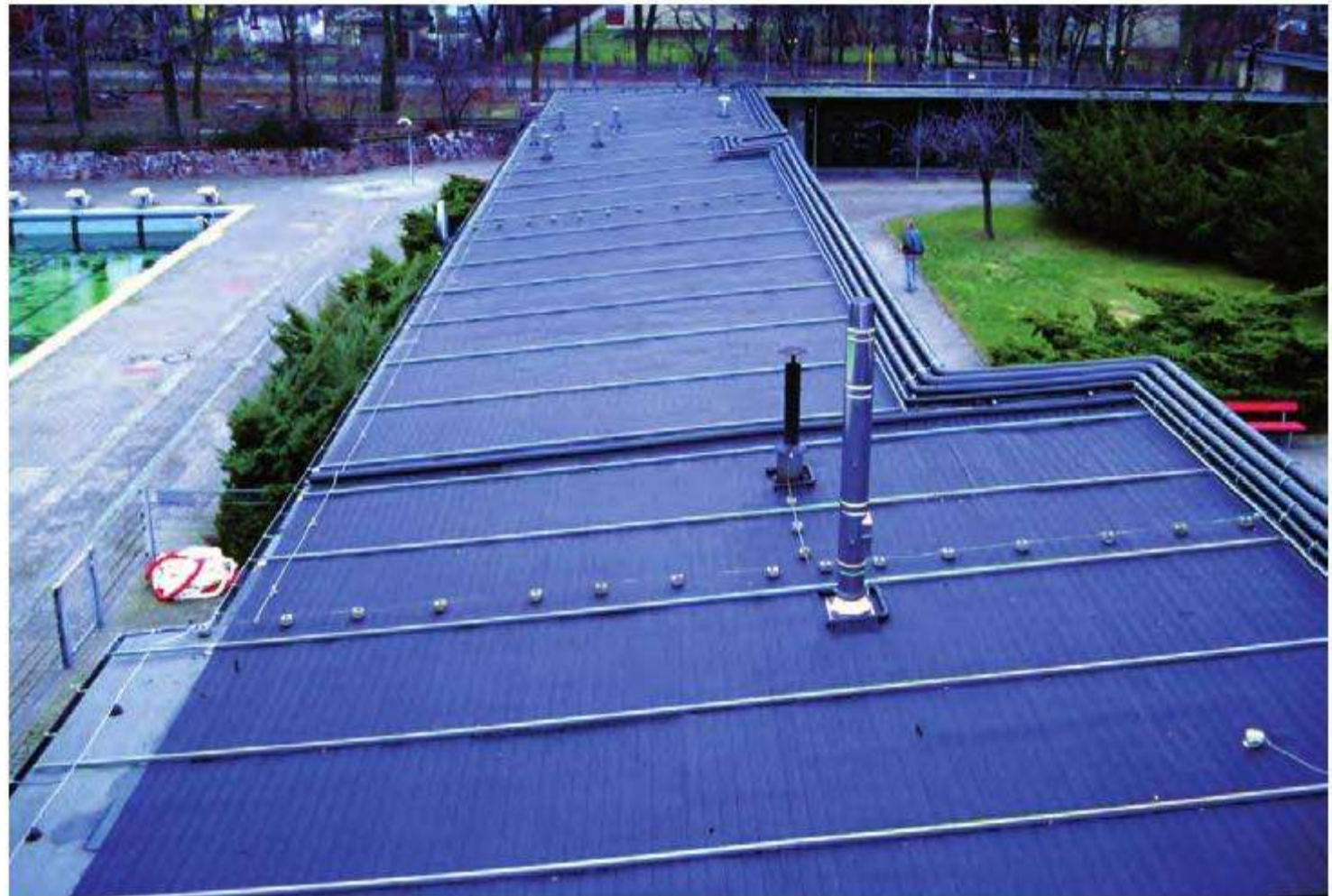
Figure 7.25. Solar system for heating open-air pool water in the Mariendorf summer pool, Berlin. Source: DGS
