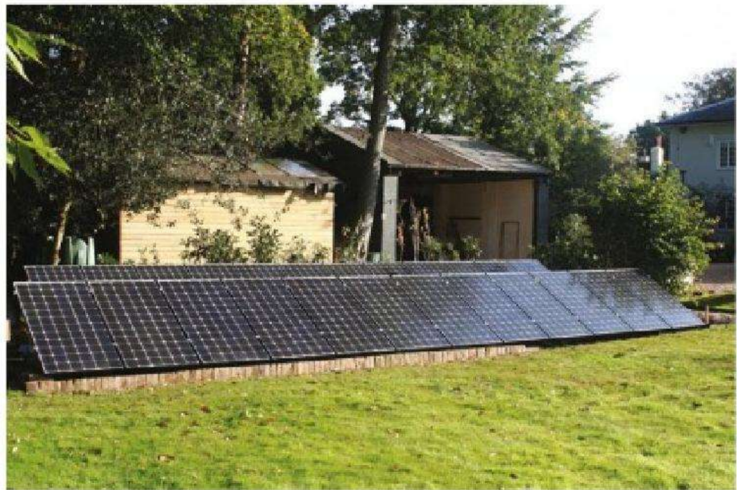
Figure 14.32 The PV array is surrounded by trees and occasionally experiences shading
