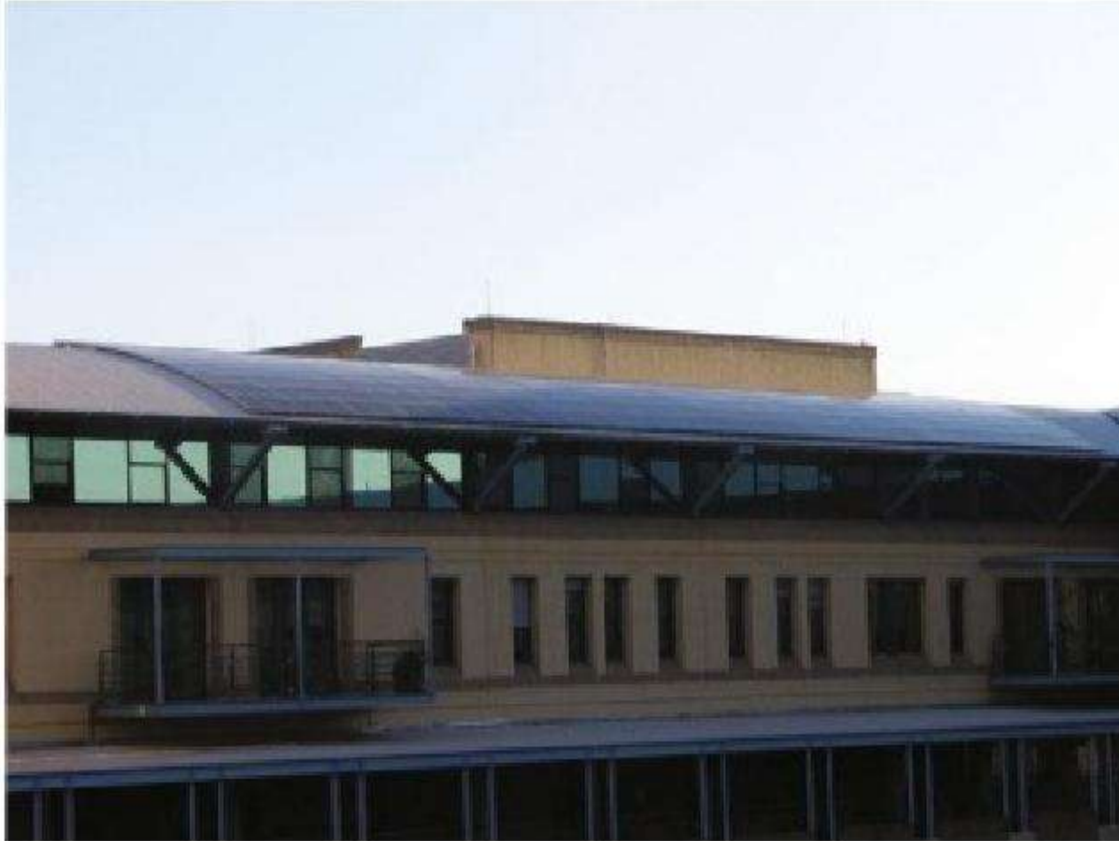
Figure 6.8 This PV system has been designed to discreetly blend in with the architecture through the use of a curved direct mounting system
