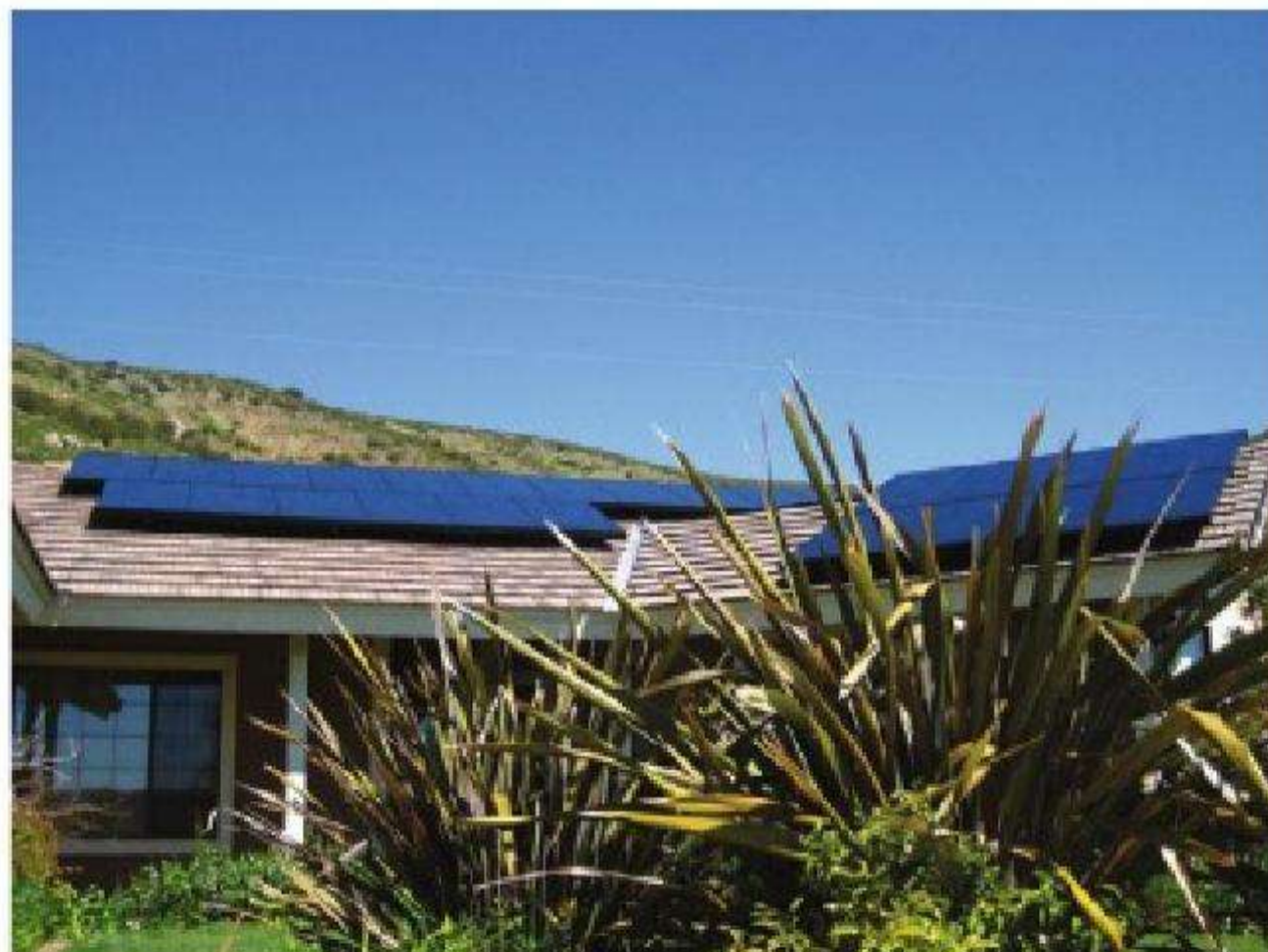
Figure 14.24 The completed system takes advantage of the available roof space in the most efficient way possible. The sleek, all black PV modules and low-profile racking are considered aesthetically attractive
