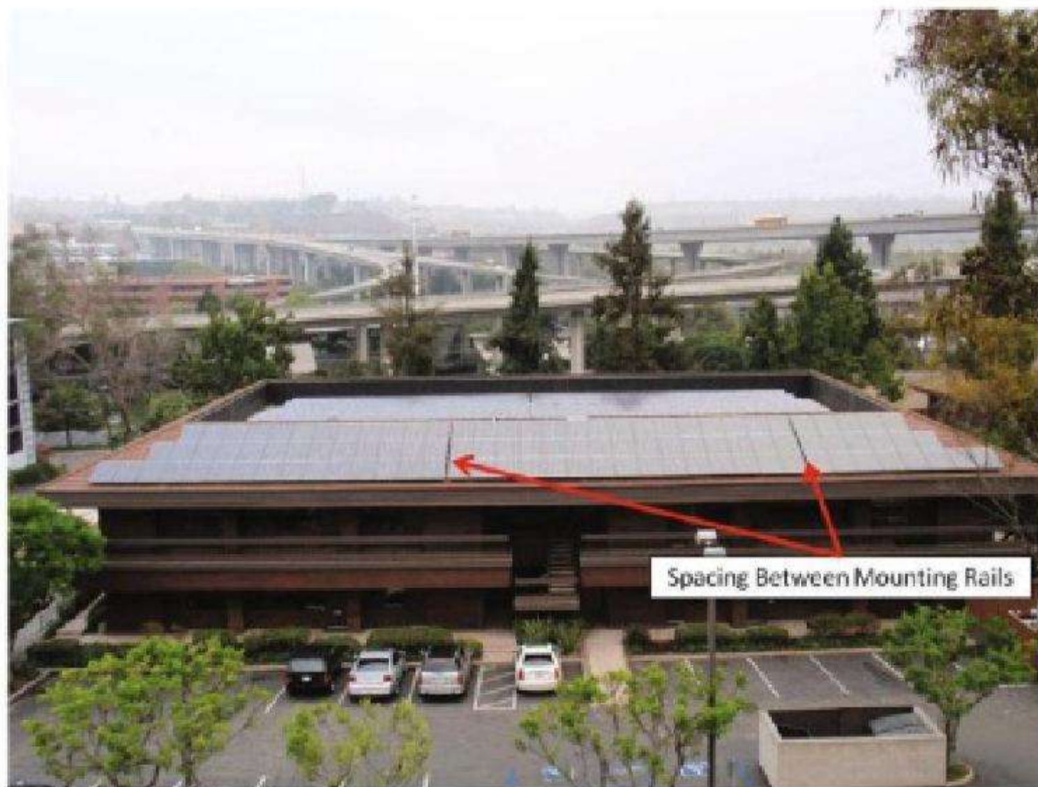
Figure 14.14 The mounting rails have been installed with periodic gaps between adjacent rails allowing the metal rails to thermally expand without damaging the mounting structure
