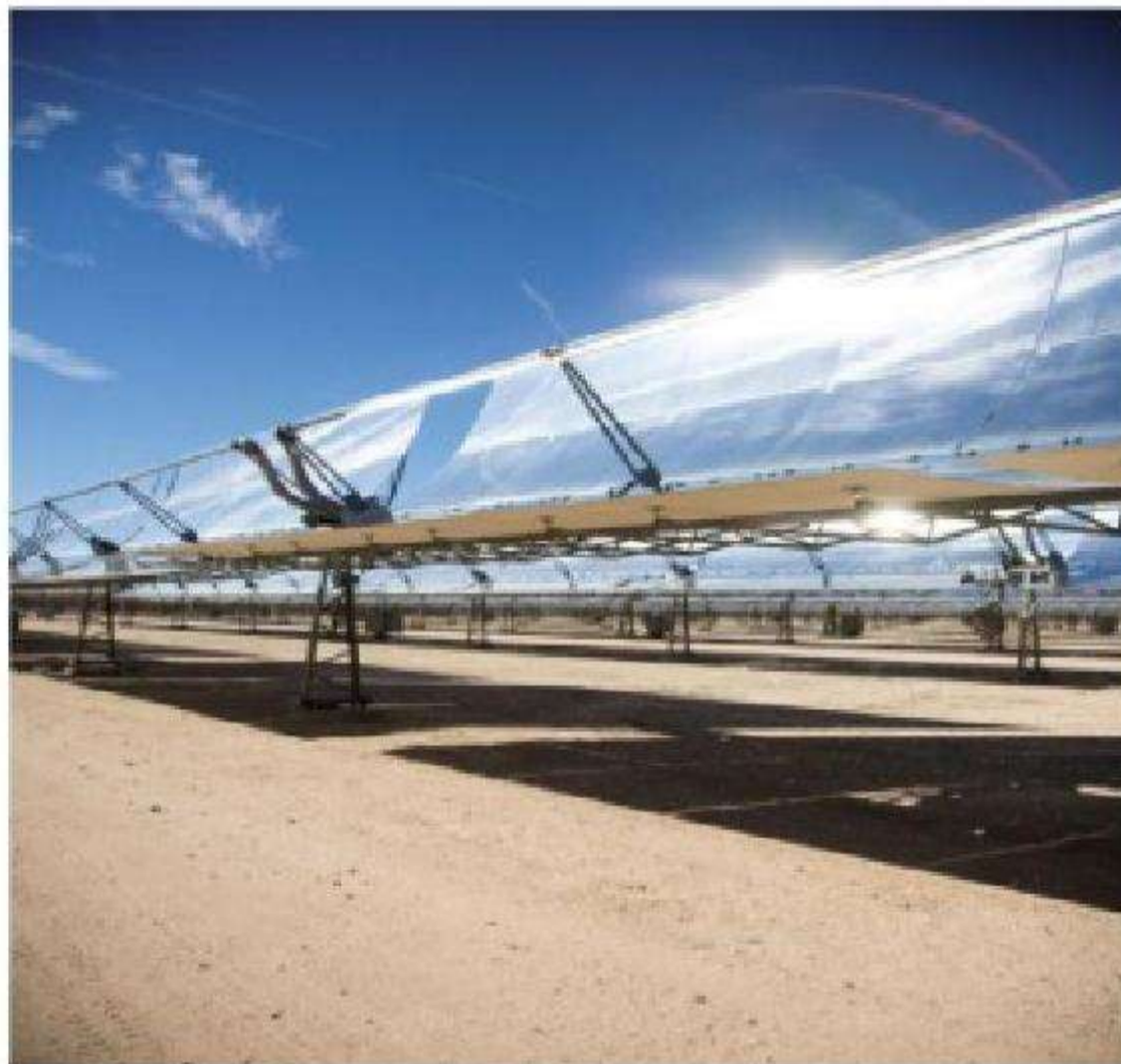
Figure 1.14 A CSP installation in the Nevada Desert. Parabolic mirrors concentrate sunlight to heat the water running through the thin tubes in front of the mirrors
