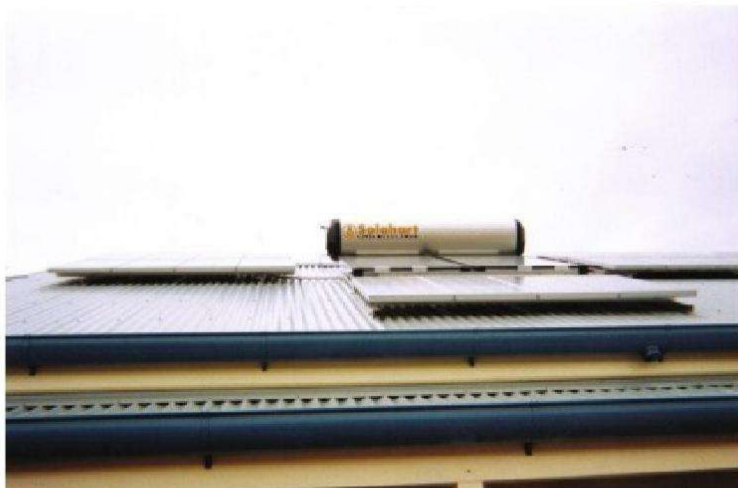
Figure 6.1 This mounting scheme allows good ventilation. Mounting panels closer to the roof increases operating temperature and thereby lowers system performance
