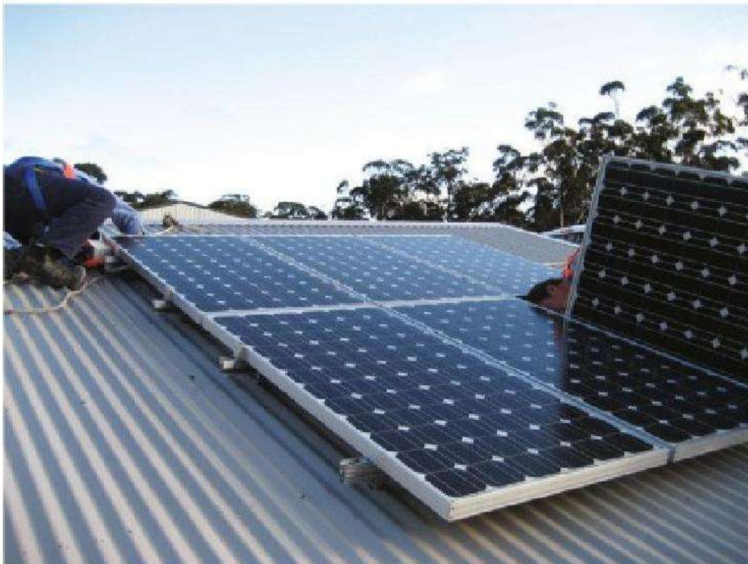
Figure 6.6 Corrugated metal roof installation
