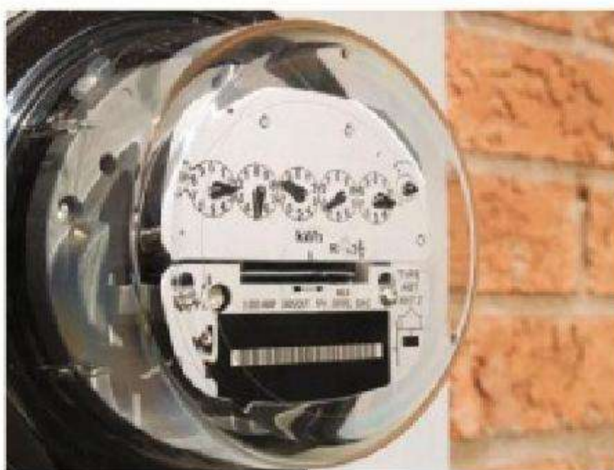
Figure 5.37 An electricity meter commonly used in the US
