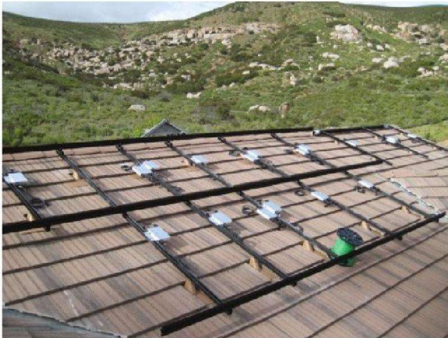
Figure 14.21 In order to overcome the challenges presented by this residential roof, the system designer decided to forgo the traditional central inverter system architecture and install micro-inverters on each solar module. The micro-inverters are mounted on to the rails directly beneath the modules and convert the DC current from the PV module into AC current. Each individual micro-inverter has its own MPP tracking system so that the performance of each PV module is completely independent of its neighbours. The AC outputs are connected in parallel and then feed directly into the residential main service panel
