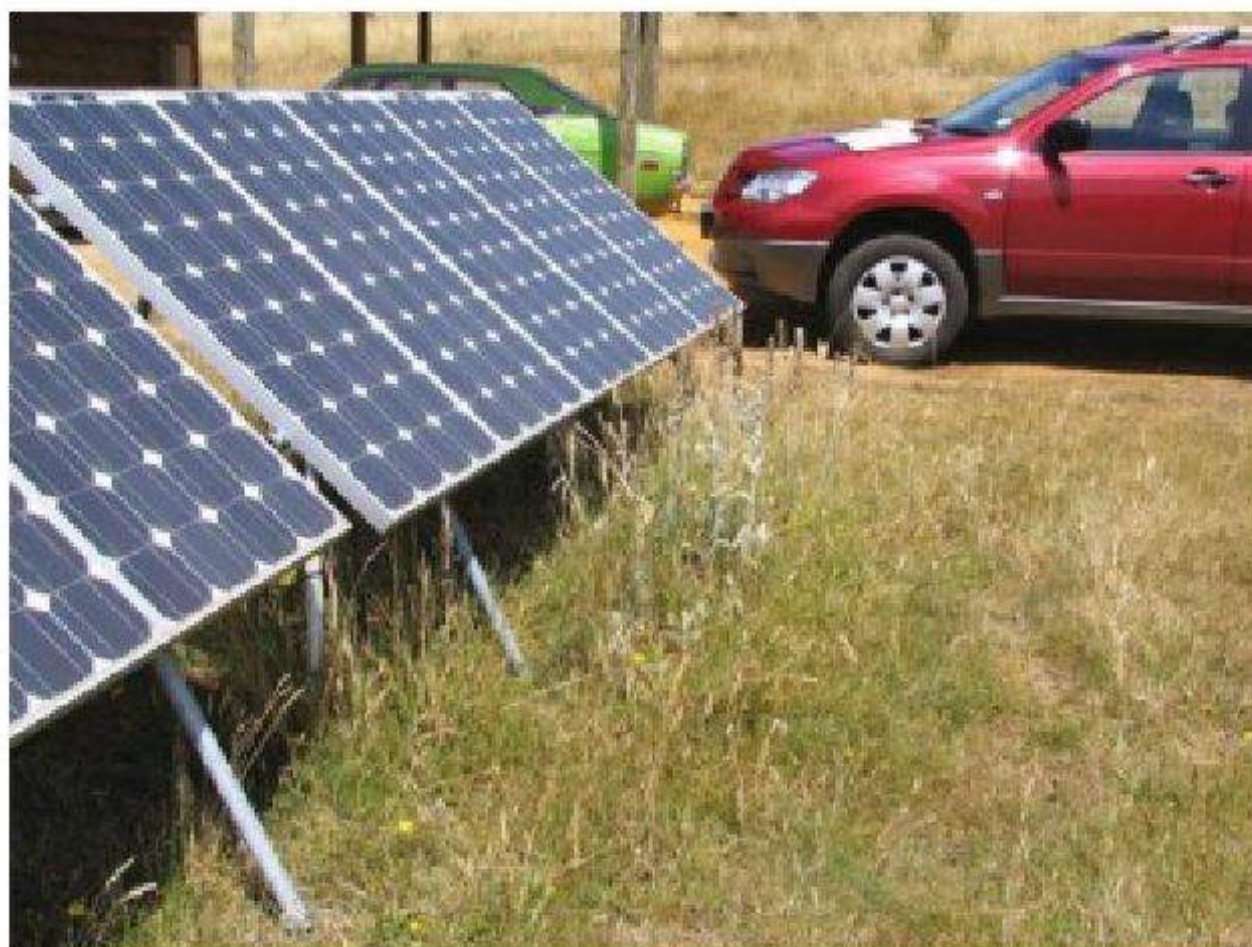
Figure 6.14 The grass is low now, but if it grows high enough it could shade the array
