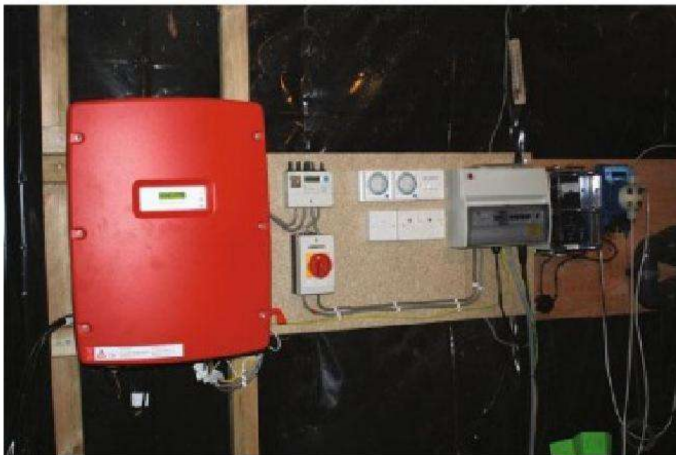
Figure 14.31 The inverter is located in the pool shed behind the PV array; the inverter is connected to a generation meter which measures the PV array's power output, then to a lockable double pole isolating switch and then directly into one of the miniature circuit breakers located on a distribution board in the shed
