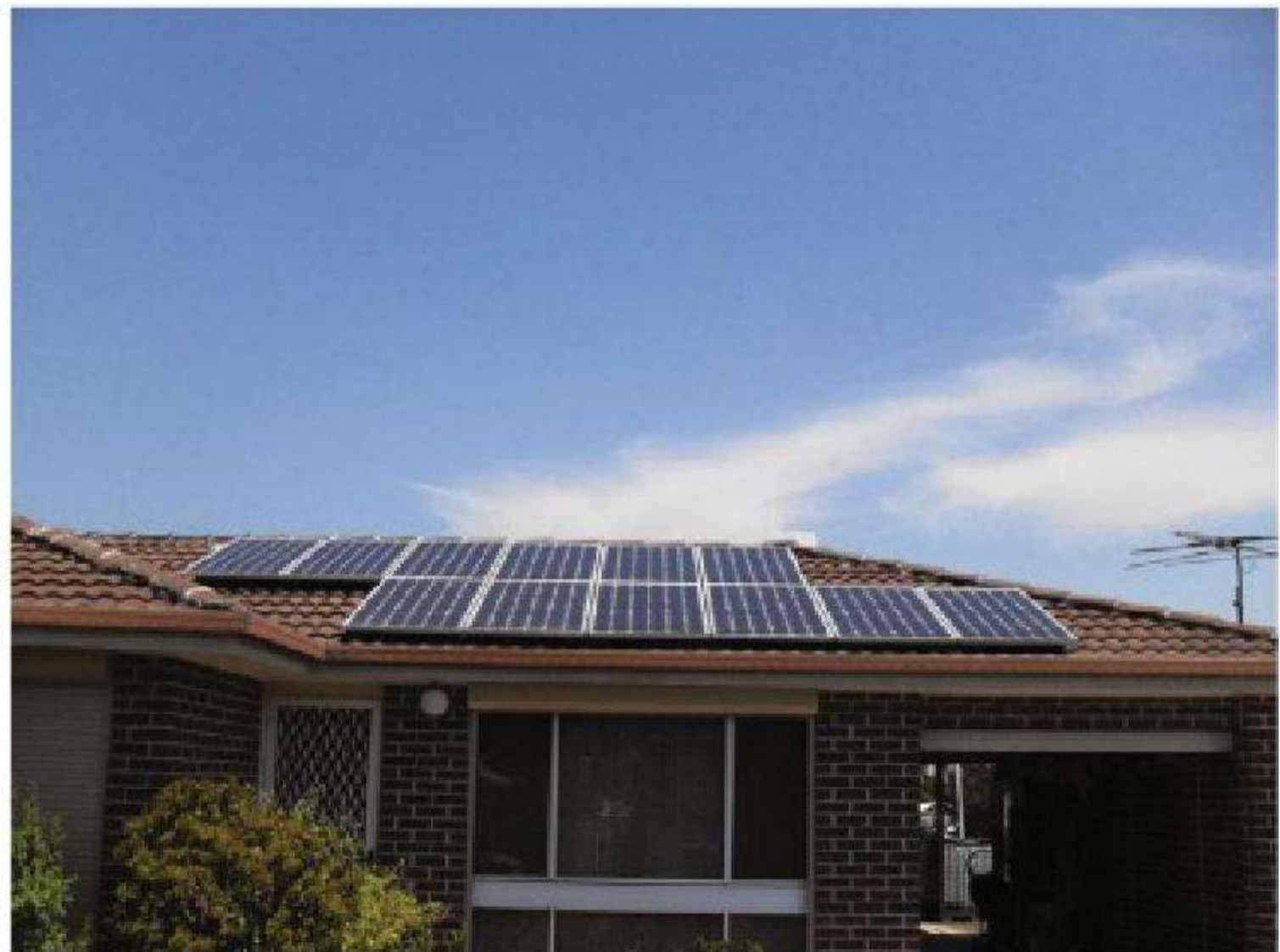
Figure 14.18 The PV array blends in with the profile of the roof and is aesthetically pleasing while allowing some cooling air flow beneath the modules
