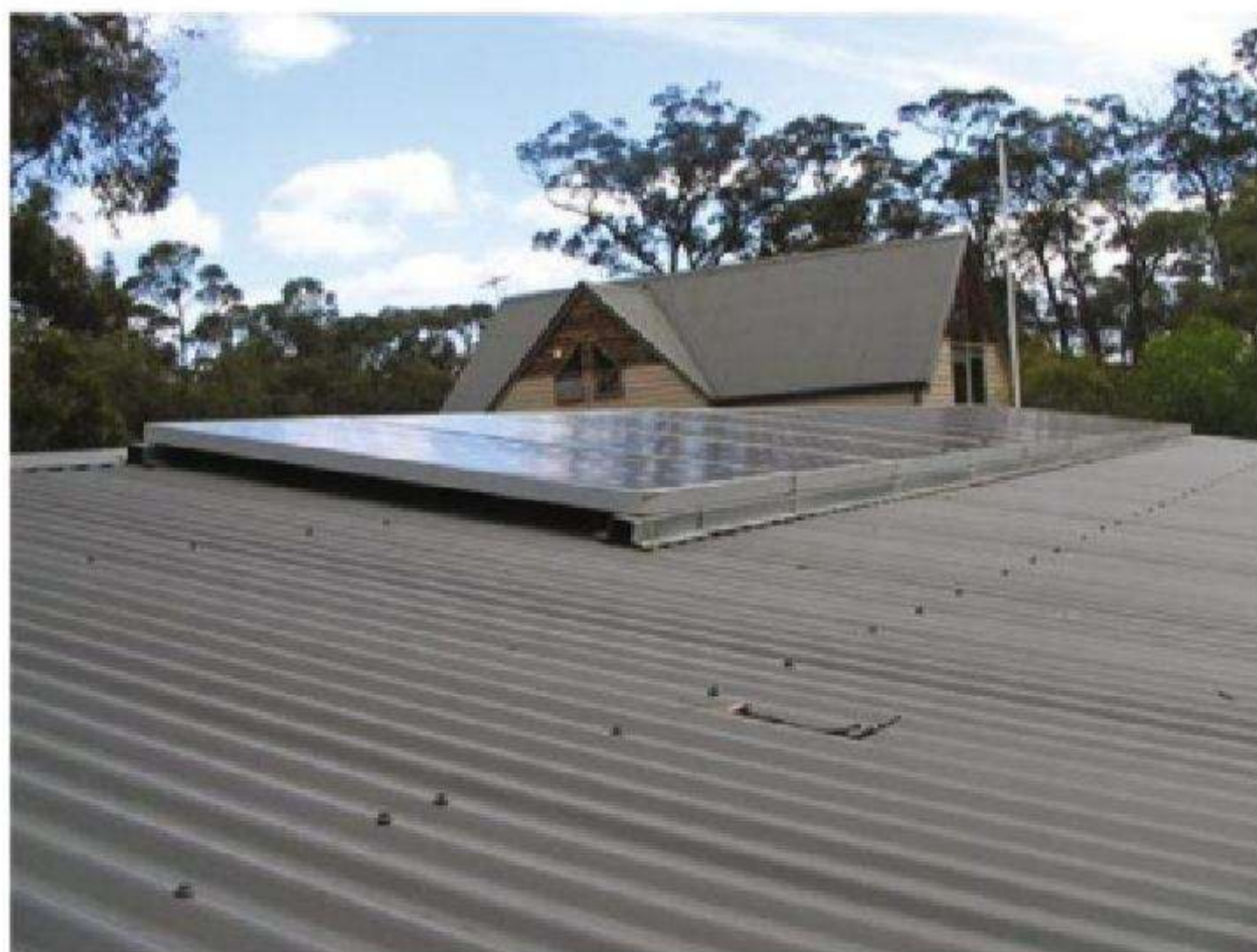
Figure 6.2 This mounting scheme will not permit good airflow
