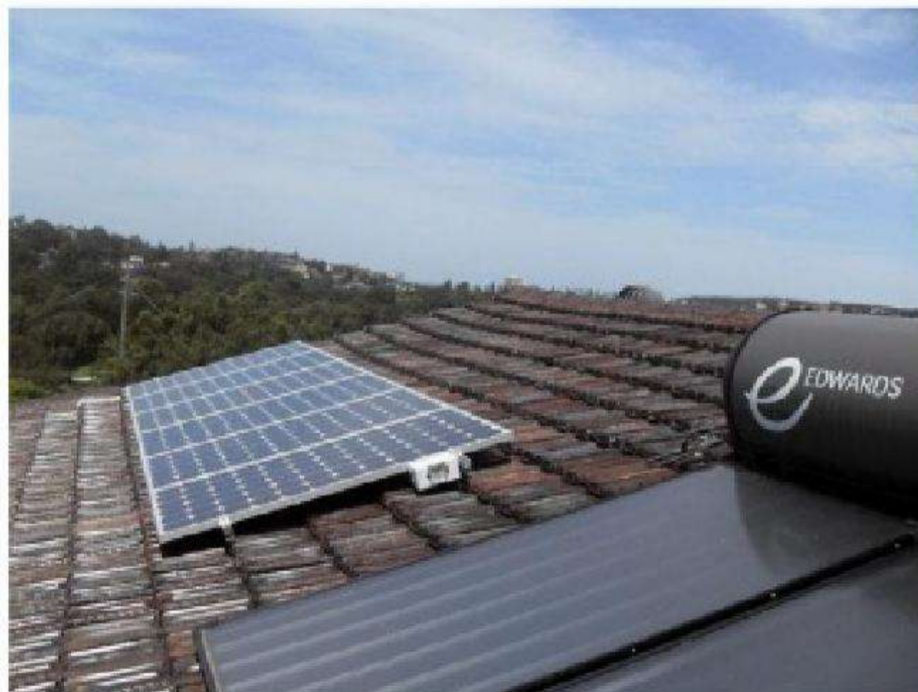
Figure 1.12 This system includes a solar electric system (back) and flat plate solar hot water system with a storage tank (front)
