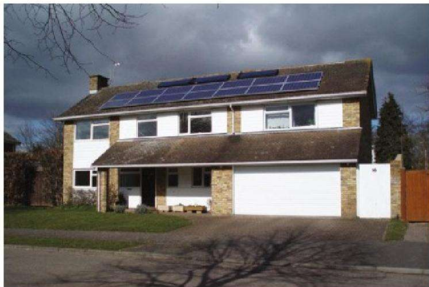
Figure 14.9 In order to meet the household energy demands 14 PV modules and 3 solar thermal collectors have been installed
