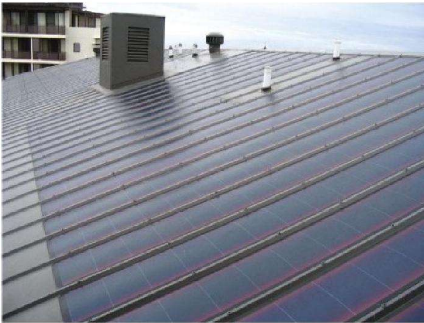
Figure 6.12 Amorphous laminates installed on metal roofing in Australia
