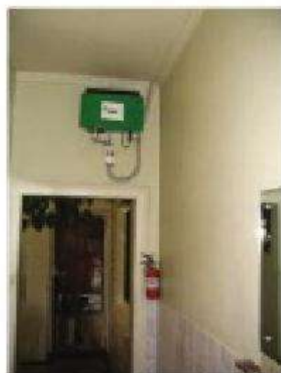
Figure 7.19 Badly located inverter; the system owners will have great difficulty accessing information from this inverter
