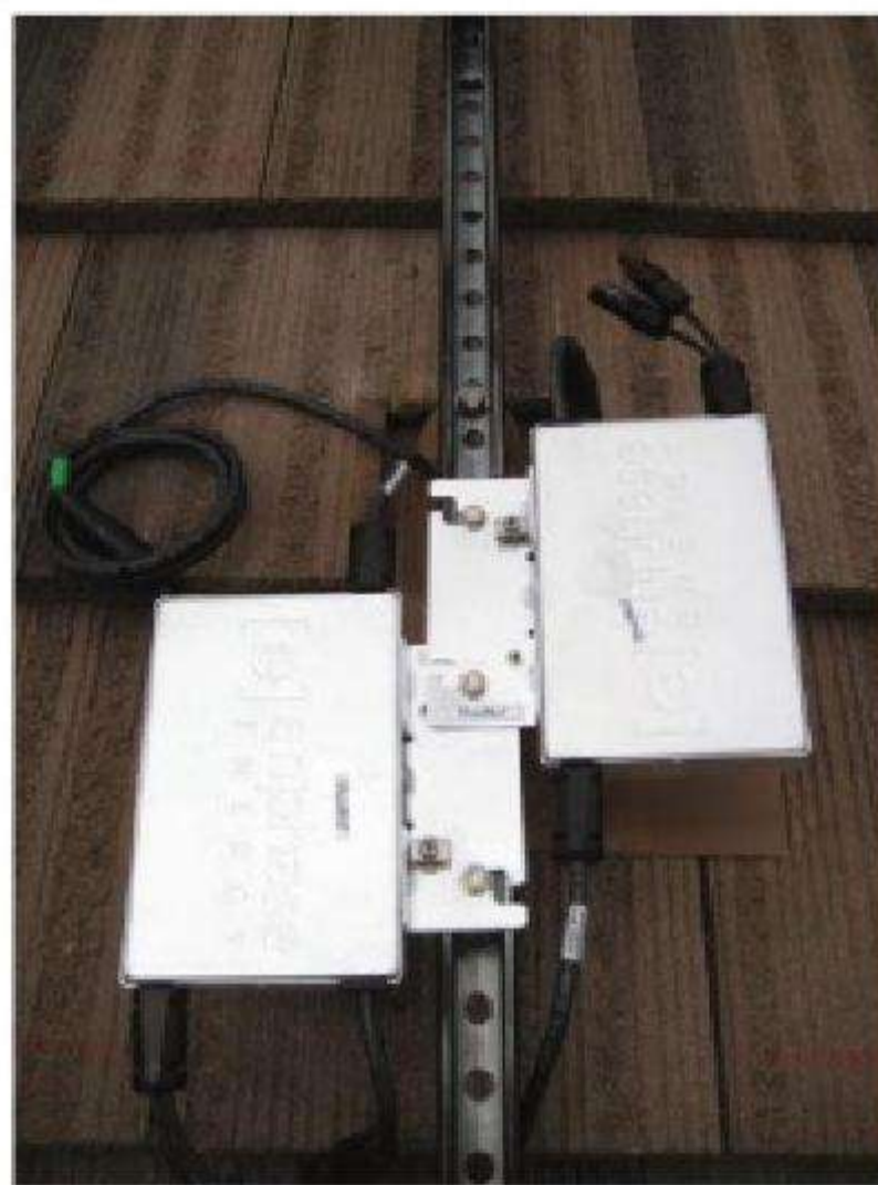
Figure 5.17 Micro-inverter available on the US market
