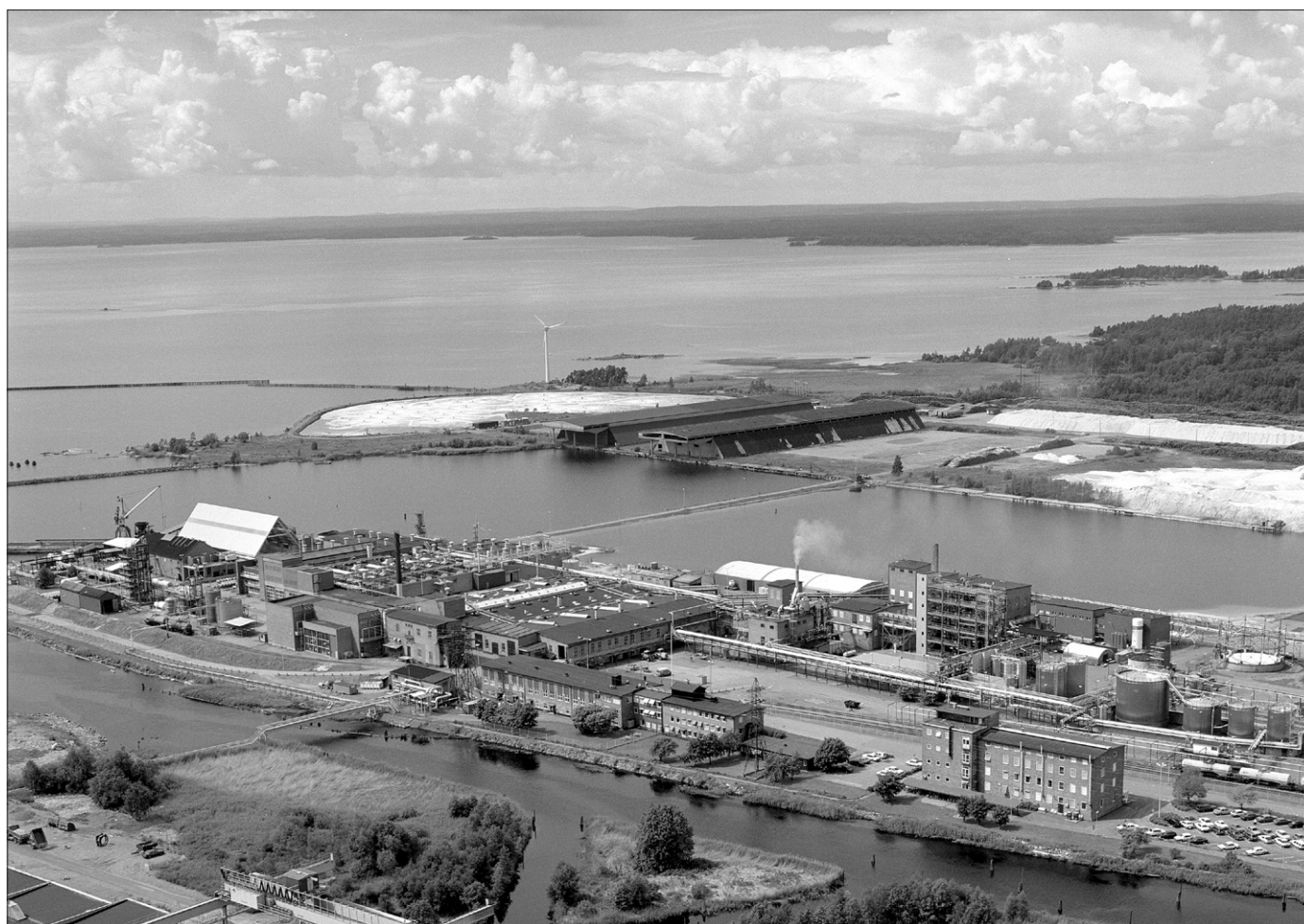
Figure 3 Changing technology. The chlor-alkali factory outside Skoghall in west Sweden once used the mercury electrode method to produce chlorine. In 1987 the new membrane-based technology was introduced, replacing all use of mercury. There has been a 100% change to this new technology in Japan, a partial change in Western Europe and USA, but no change has yet taken place in eastern and central Europe. (Photo: Courtesy of Akzo Nobel Industries)
