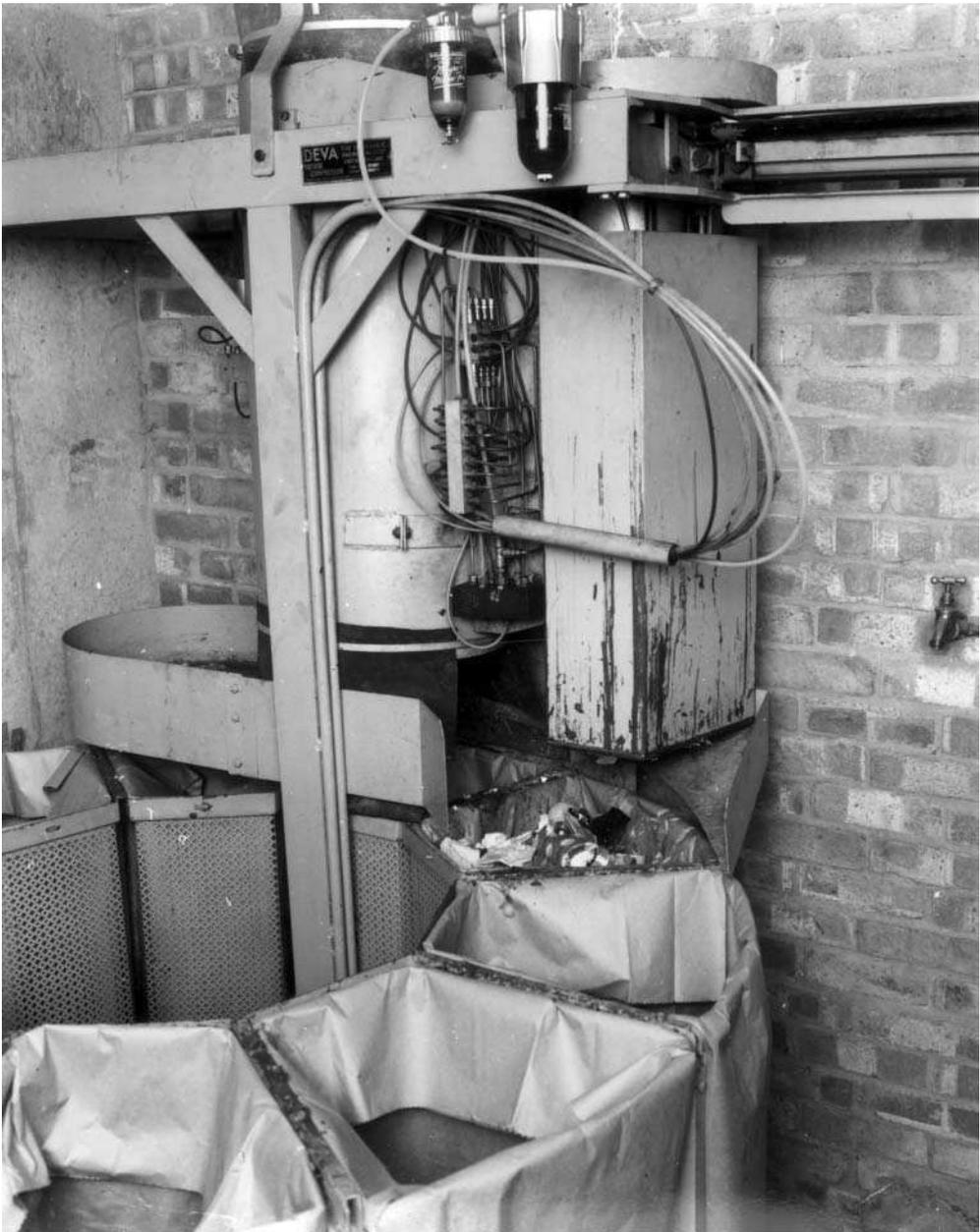
**Figure 6.4** Example of a waste compactor (DEVA) in a block of flats (Building Research Establishment; Crown Copyright)
