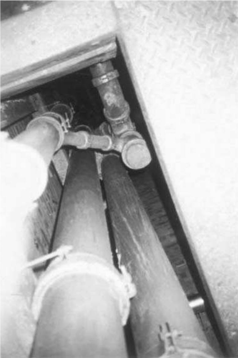
**Figure 7.6** Modified one-pipe drainage and vent system in a service shaft at the Queen's Medical Centre, Nottingham (Courtesy of Schott UK Ltd)
