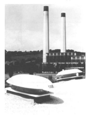
Figure 28.3 Low discharge powered roof ventilator
