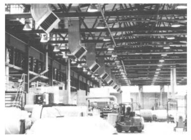
Figure 28.4 Roof inlet system
