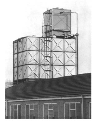
Figure 34.13 Cyclic heat load using small tower and large water storage. This is a good idea and sound engineering, but the access panel is on the wrong side (30 ft drop to ground level)
