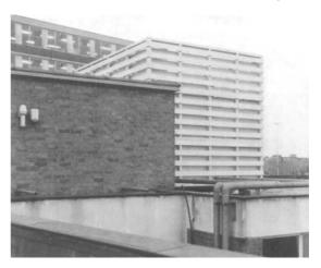
Figure 34.14 An attempt to conceal tower and reduce noise, resulting in starvation of air and failure in performance
