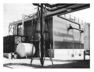
Figure 34.9 Congested site. Restrictions on air inlet, increased pressure and air velocity results in drift deposition on road
