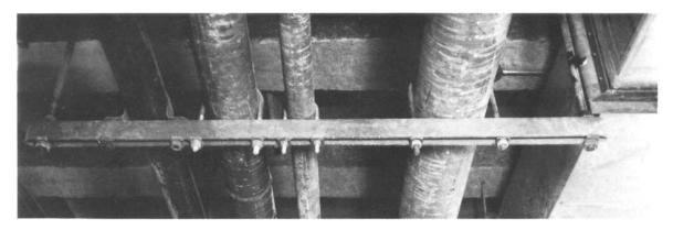
Figure 6.13 A typical multi-service gang hanger (courtesy of Industrial Hangers Ltd)
