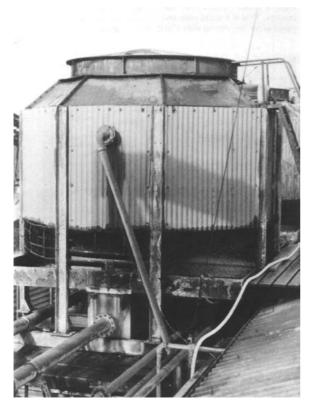
Figure 34.16 The effects of corrosion. Structural failure is visible (holes in fan casing)
