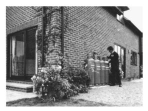
Figure 20.10 A 2  $\times$  2 LPG cylinder pack supply domestic premises. (Courtesy of the Calor Group Plc)
