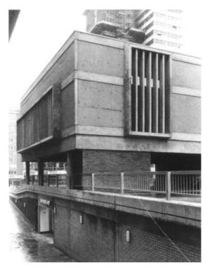
Figure 34.6 Cooling plant, including towers, installed as a separate unit on a supermarket satisfies the architect, town planners and the end-user
