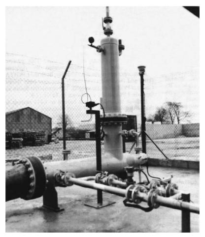
Figure 20.6 Hot-water heated LPG vaporizers. (Courtesy of Esso Petroleum Co. Ltd)
