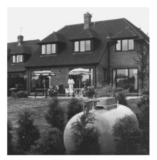
Figure 20.5 LPG storage vessel for a domestic installation. (Courtesy of the Calor Group Plc)
