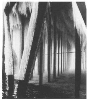
Figure 34.15 Ice on natural-draft tower (no de-icing ring fitted)
