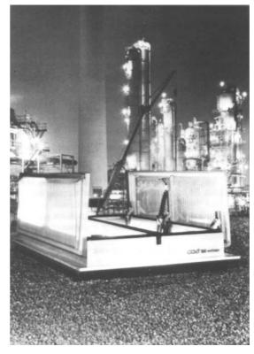
Figure 28.8 Flap type roof ventilator
