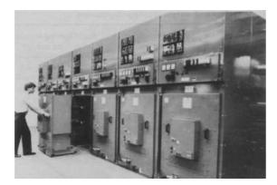
Figure 16.2 NEI Reyrolle SF<sub>6</sub> switchgear
