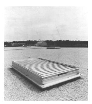
Figure 28.7 Louvered roof ventilator
