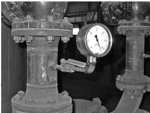
FIGURE 8.11 A ball valve used to isolate a pressure gauge. Note the lack of a pressure bleed valve on the pressure gauge, as well as the inconvenient handle position of the ball valve.
