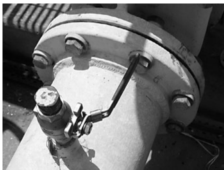
FIGURE 7.11 A dielectric connection on a flange pair.
