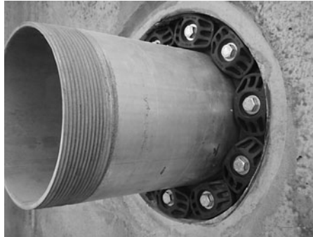
FIGURE 6.14 An elastomeric seal through a concrete containment. Artwork provided by psi—Pipeline Seal & Insulator, Inc. Link-Seal® Modular seals is a registered trademark of psi.
