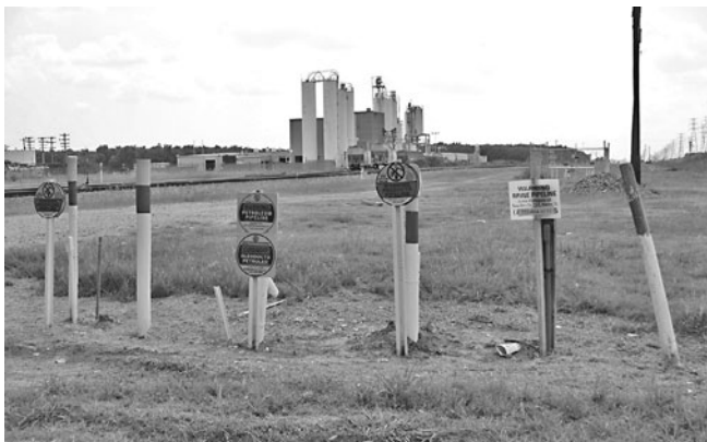
FIGURE 15.4 A densely-populated underground pipeline right-of-way is identified with above-ground markers.
