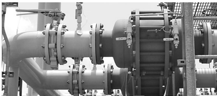
FIGURE 8.15 A lug-type butterfly valve downstream of a detonation arrestor. Note that the position of the handle indicates that this valve is open.
