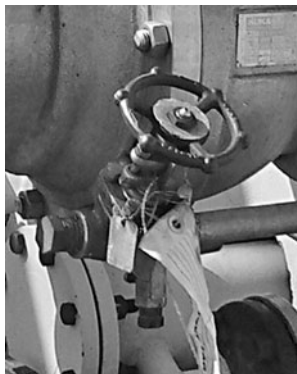
FIGURE 8.3 A 1 in gate valve used as a steam-out connection.
