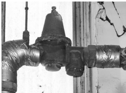
FIGURE 8.17 A pressure regulating valve on a cooling water line.
