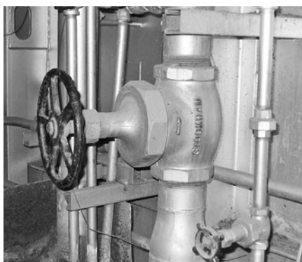
FIGURE 8.5 A globe valve with a union bonnet. Note the direction arrow embossed on the body.
