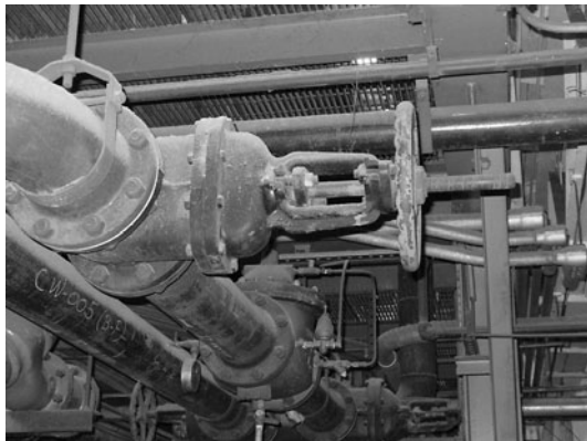
FIGURE 8.2 A rising stem gate valve in the open position. Note the full face gasket on the near flange pair.
