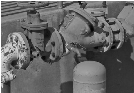
FIGURE 8.36 A reduced pressure backflow preventer with a hose bibb attached. The hose bibb constitutes a cross connection since the potential exists to attach a hose upstream of the backflow preventer.
