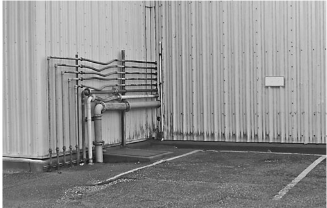
FIGURE 15.6 No protection at a parking area from physical damage of utility lines. Some of these lines contained oxygen and flammable gases.
