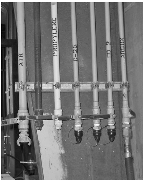
FIGURE 16.1 A typical utility drop with valves and identification of services.
