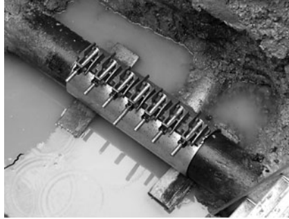
FIGURE 6.2 A hubless coupling used to repair a failed bell-and-spigot joint.
