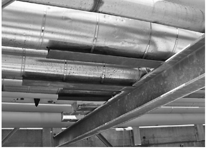
FIGURE 9.8 A shoe that has slipped off of support steel will place high stress on pipe and support steel upon cooling.
