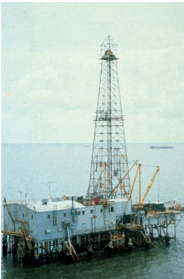
Fig. 14.1—Breton Rig 20, a converted “posted” swamp drilling barge capable of drilling in open Louisiana water depths up to 20 ft in 1949. Retired in 1962.
