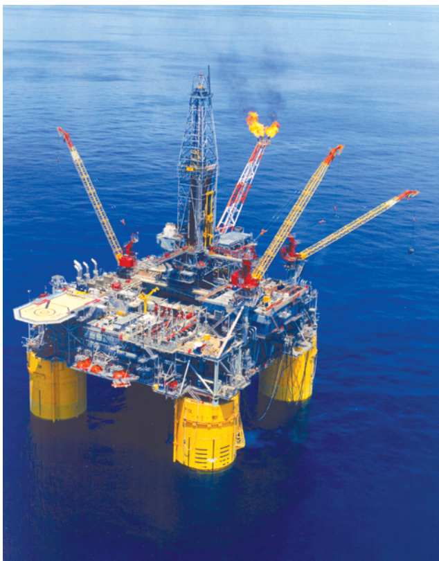
Fig. 14.15—Example of highly specialized and site-specific modular fixed-platform rigs used on spars, deepwater fixed platforms, and TLPs. This unit is on a TLP in the GOM. Courtesy Helmerich & Payne Intl. Drilling Co.
