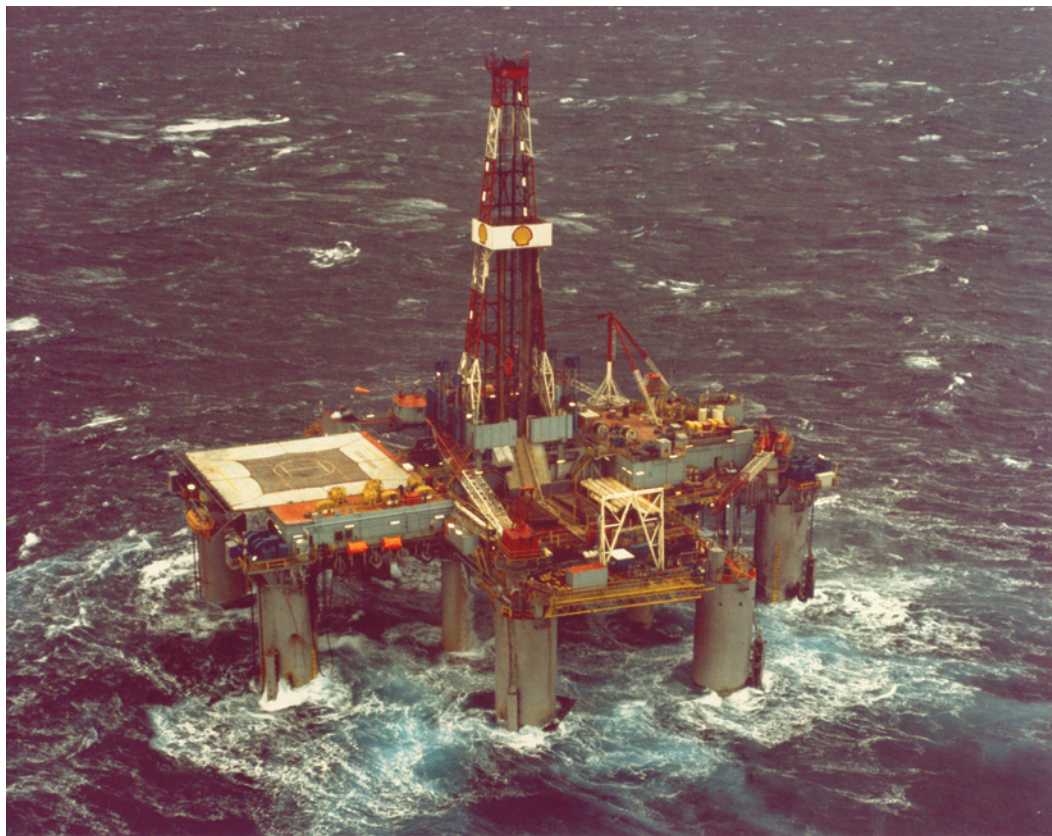
Fig. 14.12—ODECO's multicolumn second-generation semi Ocean Victory class of early 1970s. Unit shown is the Ocean Voyager , drilling in the North Sea in the early 1970s. This design proved structurally very attractive for upgrade to fourth- and fifth-generation units (see Fig. 14.14).
