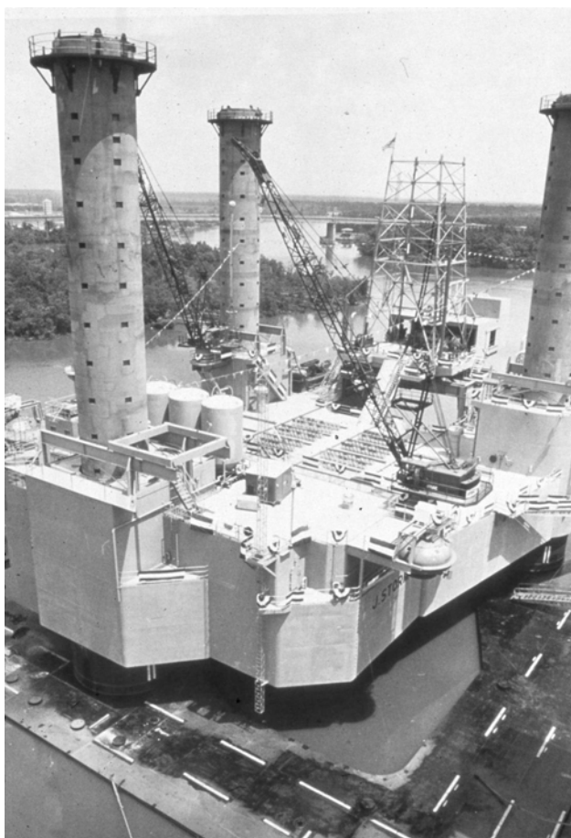
Fig. 14.19—Typical Bethlehem mat-type jackup under construction. Note size of mat and why workboats and tugs may damage it in shallow water.
