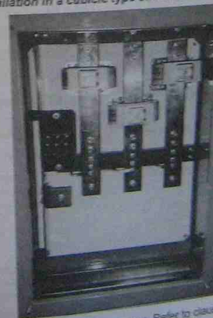
Figure 4.15: Typical CT Installation in a cubicle type switchboard
