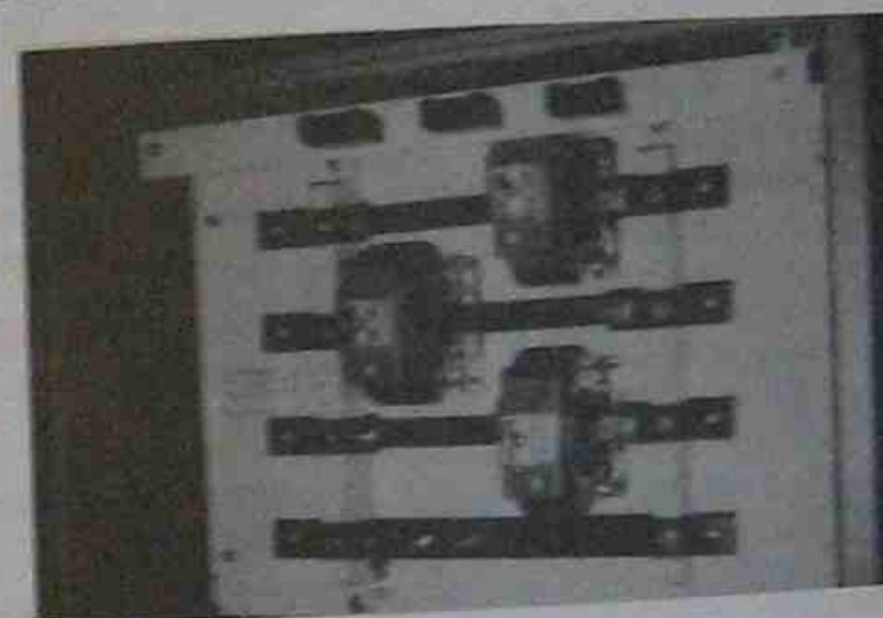
Figure 4.15: Typical CT Installation in a cubicle type switchboard
