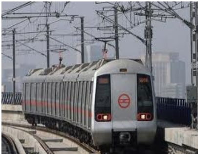
Overhead Catenary System
