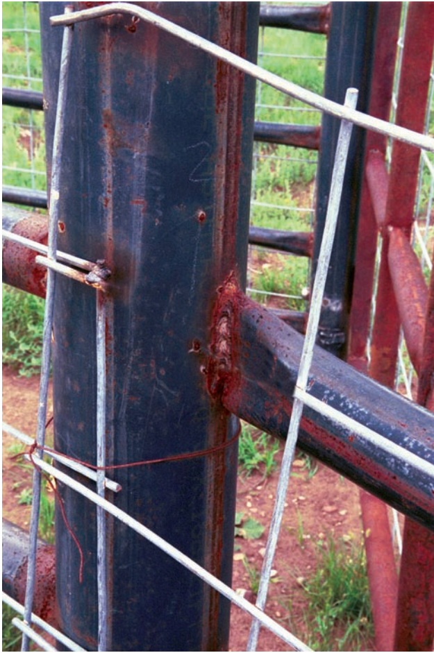
FIGURE 10-45 Pipe end bent to form a rail in a stock pen. Courtesy of Larry Jeffus.
