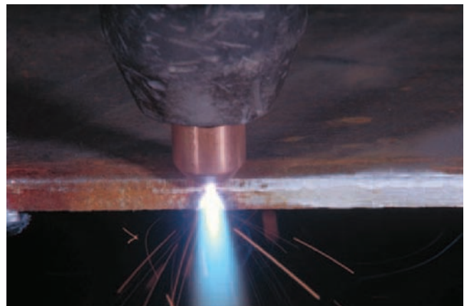
FIGURE 7-29 When the plasma cut begins, move the torch at a constant speed down the plate.
