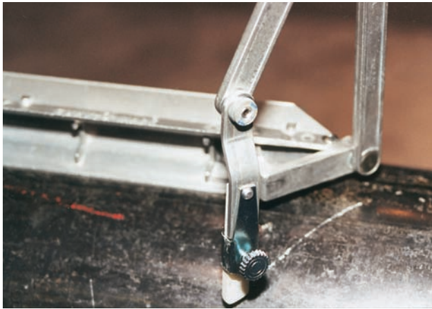
FIGURE 17-61 Pipe lateral being laid out with contour marker. Courtesy of Larry Jeffus.
