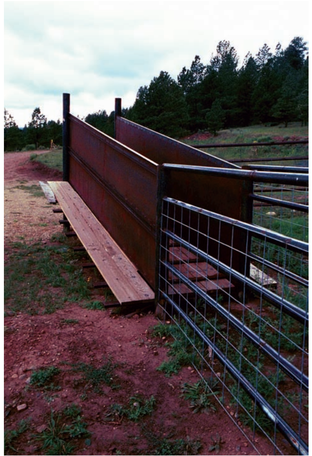
FIGURE 17-40 Wooden flooring on a metal cattle chute. Courtesy of Larry Jeffus.
