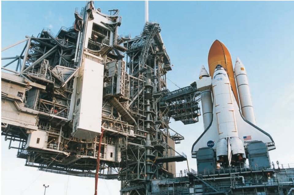
FIGURE 10-4 Space shuttle launch tower is constructed using round and rectangular tubing. Courtesy of NASA.
