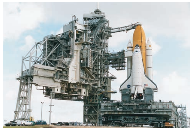
FIGURE 1-3 Space shuttle being made ready for its launch into space. Notice the large welded support structure used to prepare the shuttle for launch. Courtesy of NASA.
