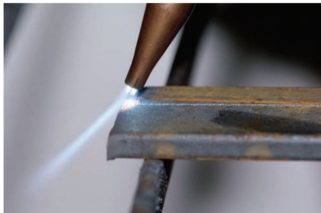
FIGURE 6-57 Beginning a cut with the torch concentrating the flame on the thin edge to speed starting.
