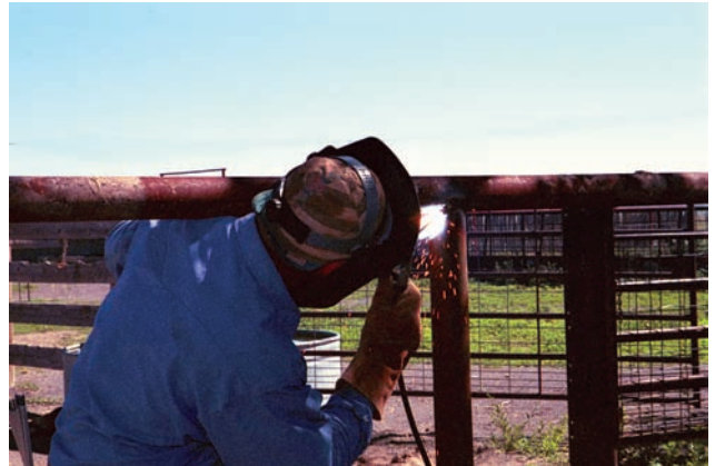
Rancher Randy Glover builds a fence, Grenville, New Mexico.
