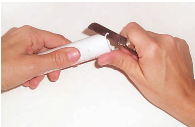
FIGURE 18-34 Chamfer the end of the PVC with a utility knife or file. Courtesy of Larry Jeffus.
