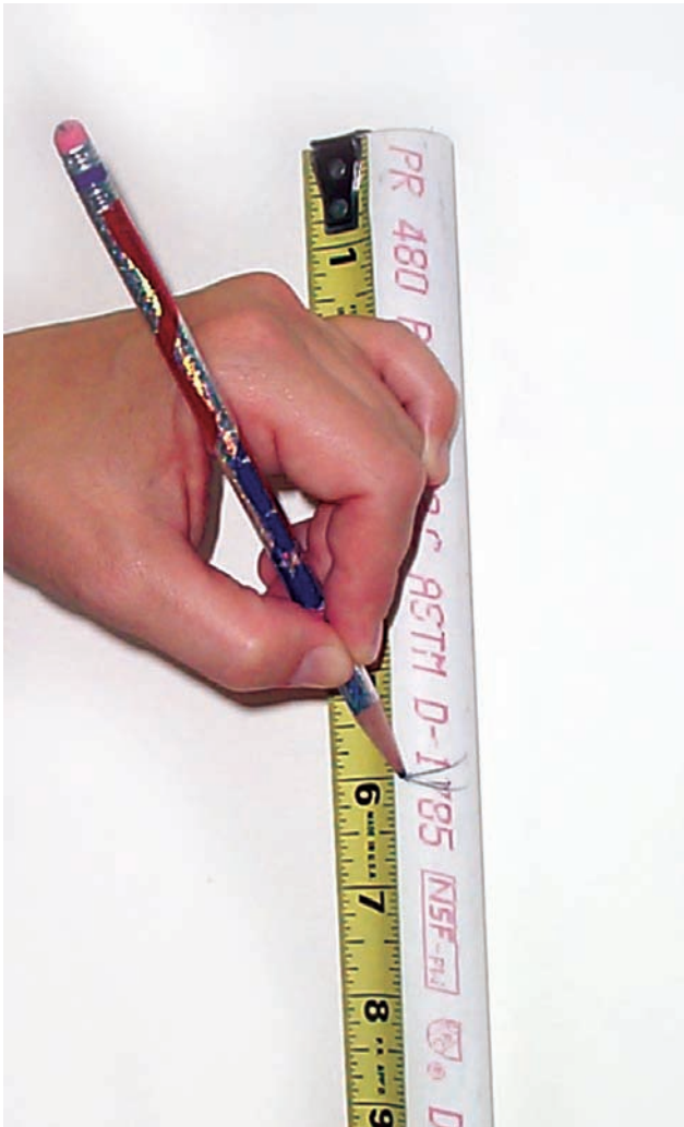
FIGURE 18-23 Measure PVC 6 in. long; make a mark to be cut. Courtesy of Larry Jeffus.
