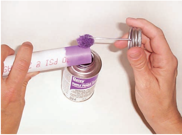
FIGURE 18-76 When the lettering has been removed, the pipe end is clean. Courtesy of Larry Jeffus.
