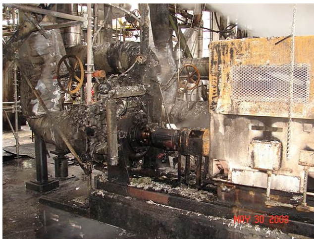
Figure 7-24: Catastrophic HVGO pump seal failure consequences.
