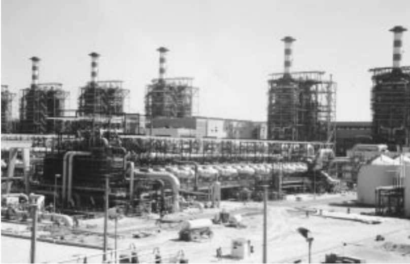
FIGURE 20.6.2 One of the six units of the 346,000 m 3 /day MSF desalination plant Al Taweelah B in Abu Dhabi, United Arab Emirates. (Courtesy of Italmimpianti S. p. A.) It is a dual-purpose plant, composed of six identical power and desalination units. Five of the six boilers are seen in the background. The desalination units were in 1996 the largest in the world. They have 17 recovery and 3 reject stages and a performance ratio (PR) of 8.1. The plant also produces 732 MWe of power.
