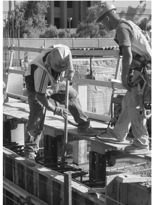
FIGURE 7.11 Consolidating concrete with an internal vibrator.
