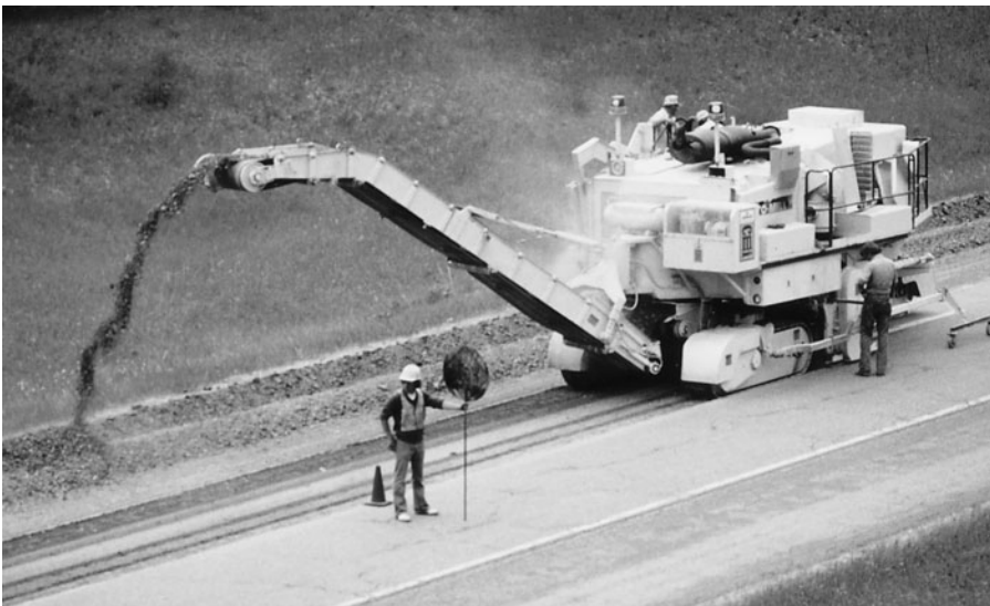
FIGURE 9.42 Milling old pavement.
