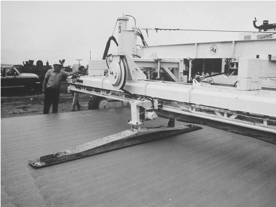
FIGURE 7.20 Finishing concrete pavement with a mechanical straightedge.
