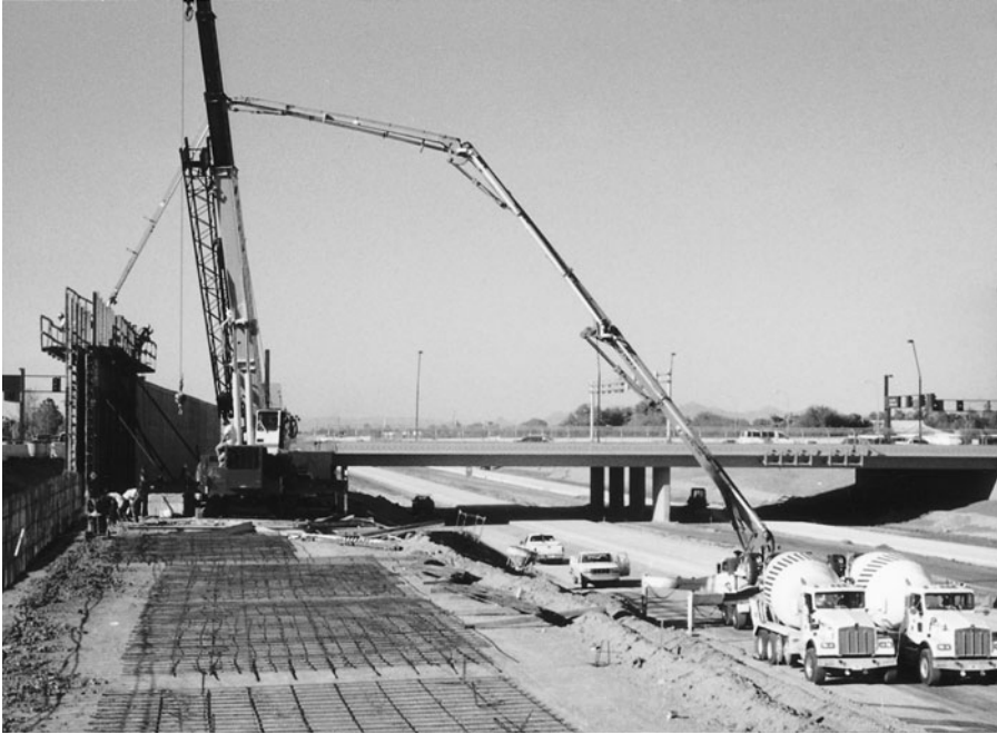
FIGURE 7.10 Pumping concrete in a retaining wall.
