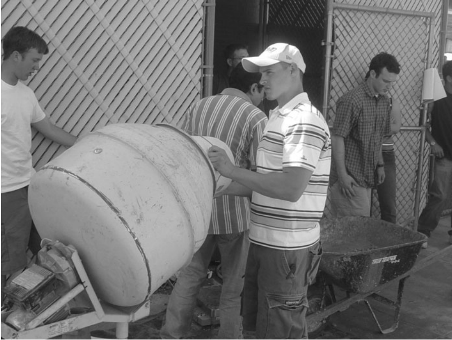
FIGURE A.27 Mixing concrete in a mixer.
