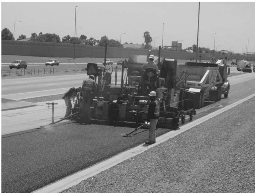
FIGURE 9.5 Placing hot mix asphalt (asphalt concrete) used for the surface layer of asphalt pavement.
