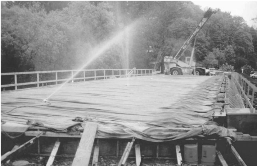
FIGURE 7.25 Curing concrete by wet covering.
