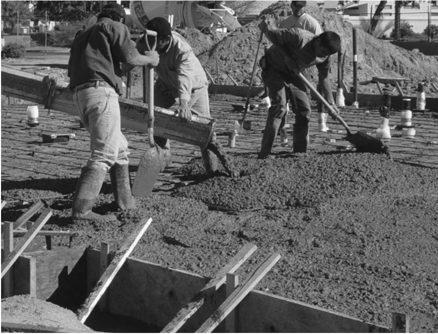
FIGURE 7.7 Placing concrete slab.
