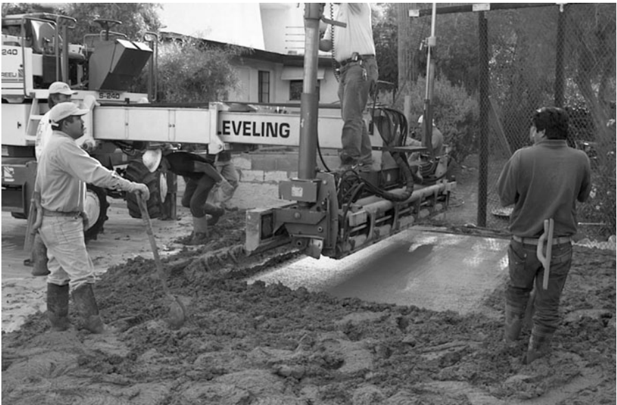
FIGURE 7.21 Using laser level to establish elevation for finishing concrete.
