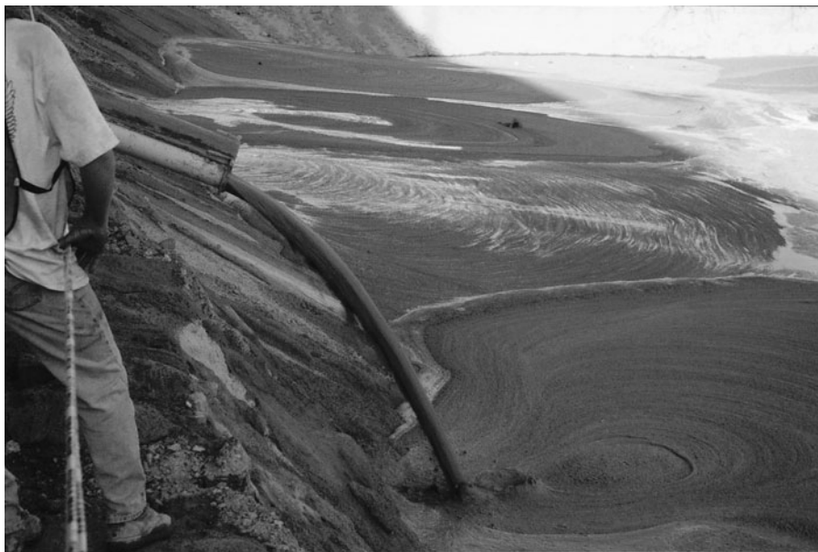
FIGURE 7.43 Filling a sink hole with flowable fill.
