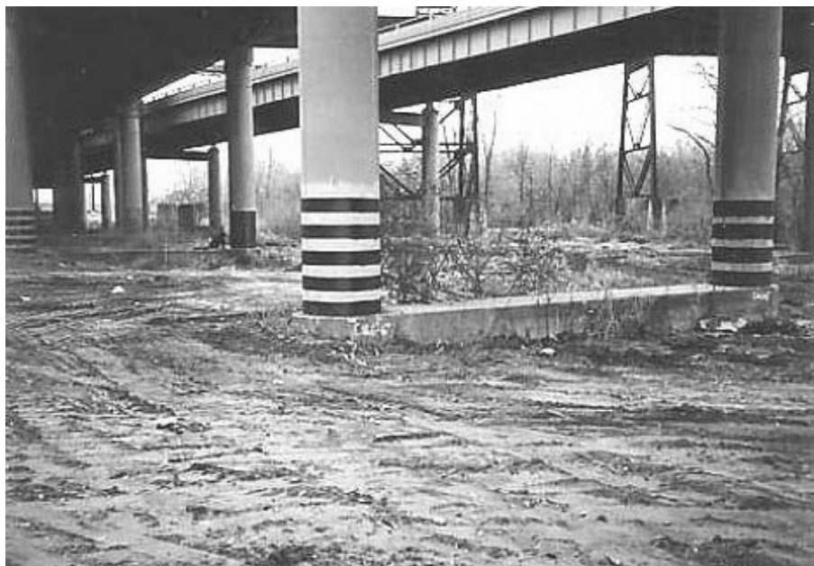
FIGURE 11.8 Wrapping columns of a bridge with FRP composites.
