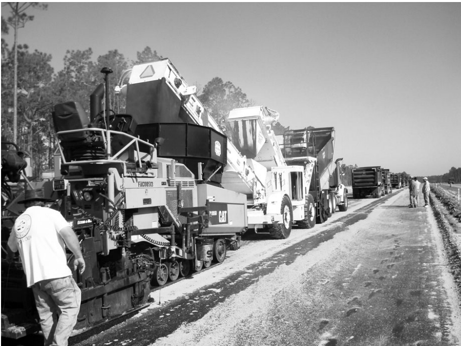
FIGURE 9.41 Material transfer devices used to transfer the HMA from the trucks to the paver.
