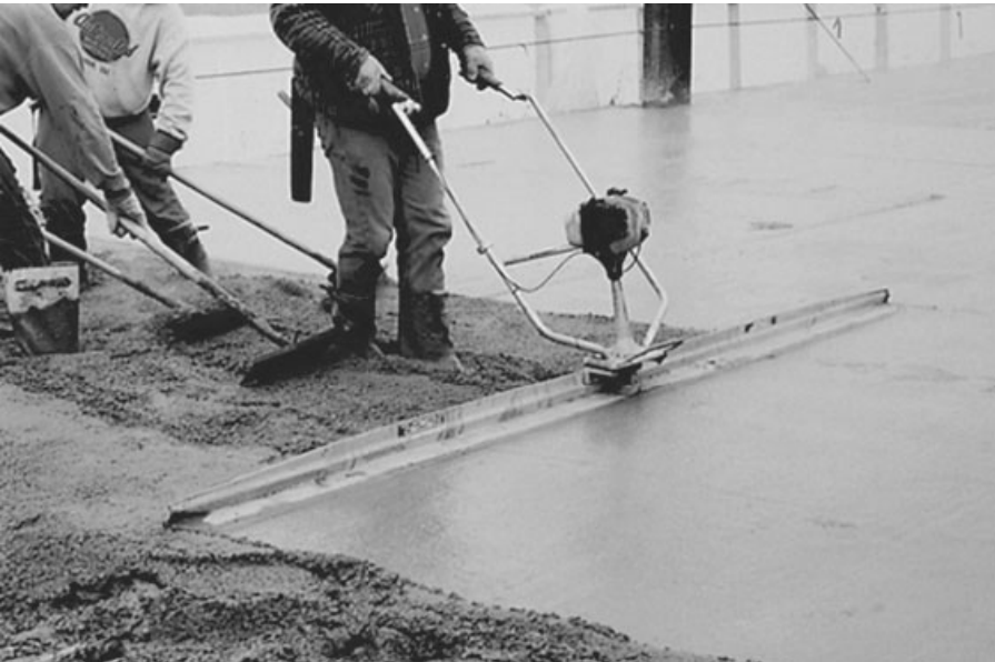
FIGURE 7.19 Finishing concrete with a vibratory screed.
