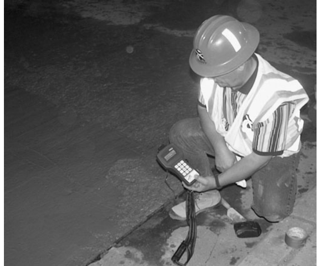
FIGURE 7.40 Checking the maturity of fresh concrete using the maturity meter.
