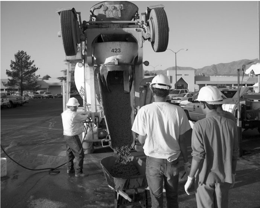
FIGURE 7.6 Loading concrete in a wheelbarrow.
