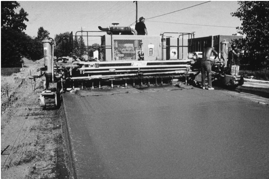
FIGURE 7.8 Placing concrete pavement with a slip-form paver.
