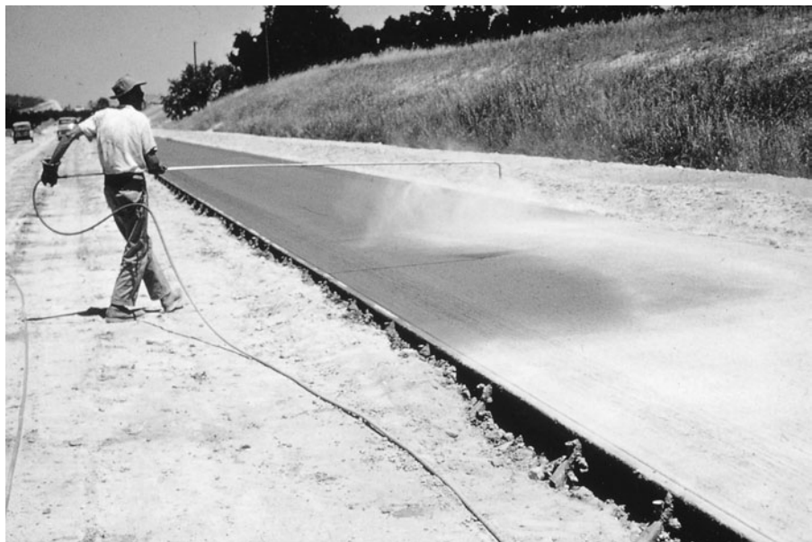
FIGURE 7.28 Curing concrete by manually applying membrane forming compound.
