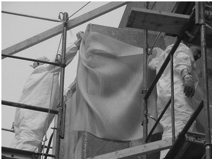
FIGURE 11.7 Wrapping an old structure with glass fiber-reinforced polymer composite (Wabash Avenue pier, Baltimore, MD).
