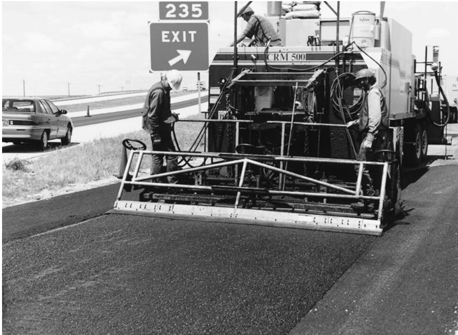
FIGURE 9.10 Applying microsurfacing for preserving existing pavement.
