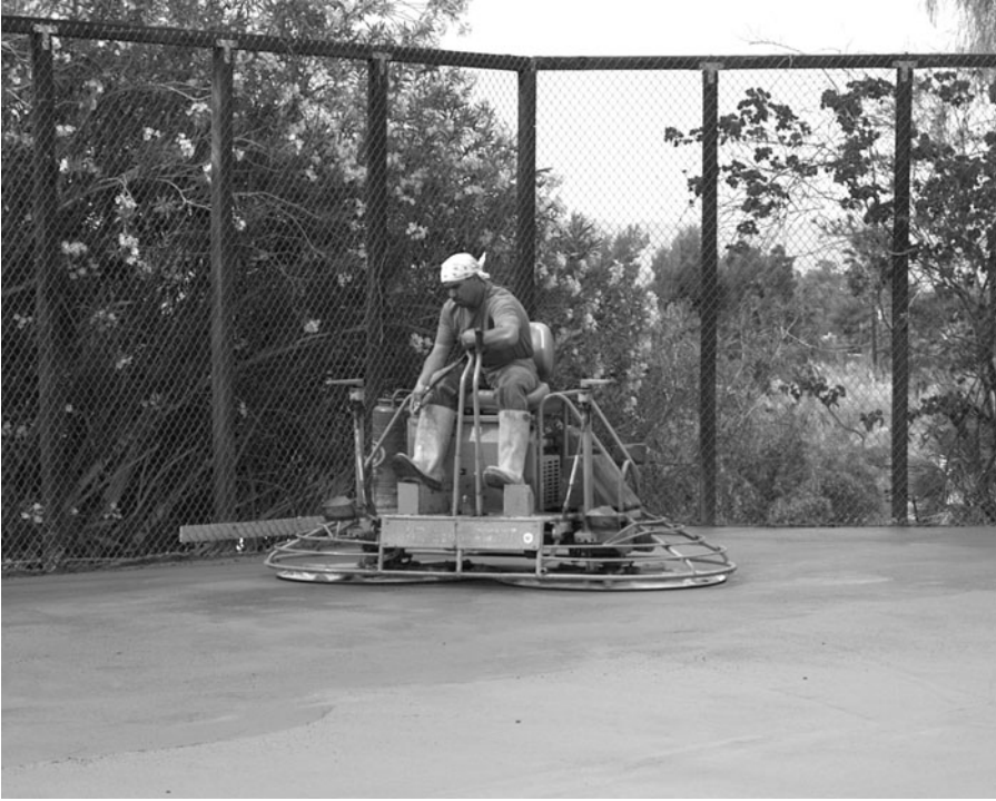
FIGURE 7.18 Finishing concrete with a power float.
