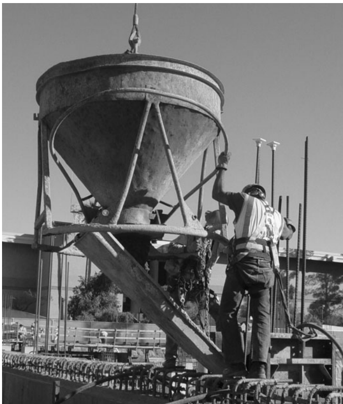
FIGURE 7.9 Depositing concrete using a 2-1/2 cubic yard bucket.
