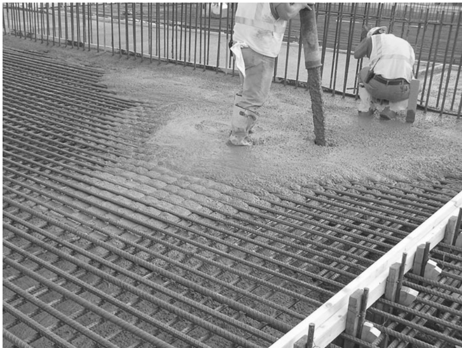
FIGURE 7.41 Placing self-consolidating concrete in a heavily reinforced slab.
