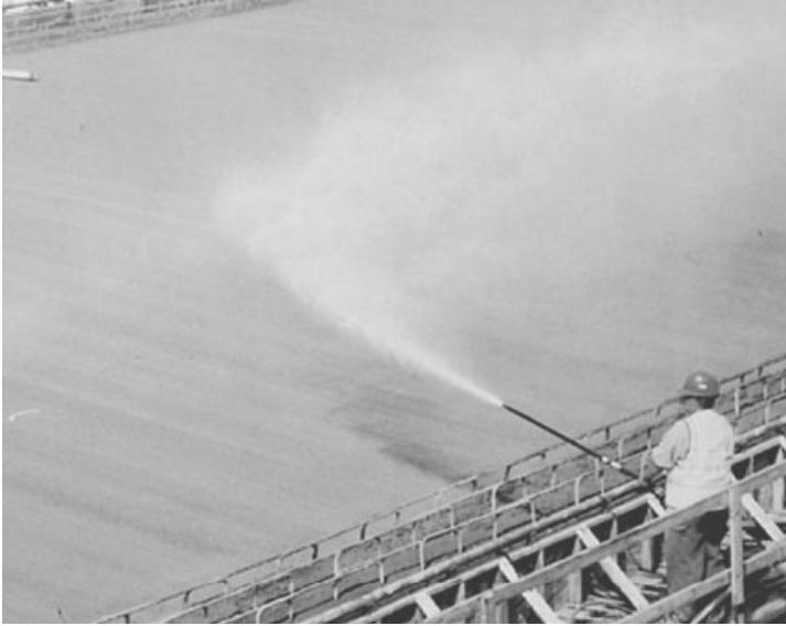
FIGURE 7.24 Curing concrete by fogging.
