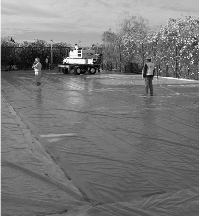
FIGURE 7.27 Curing concrete with plastic sheets.
