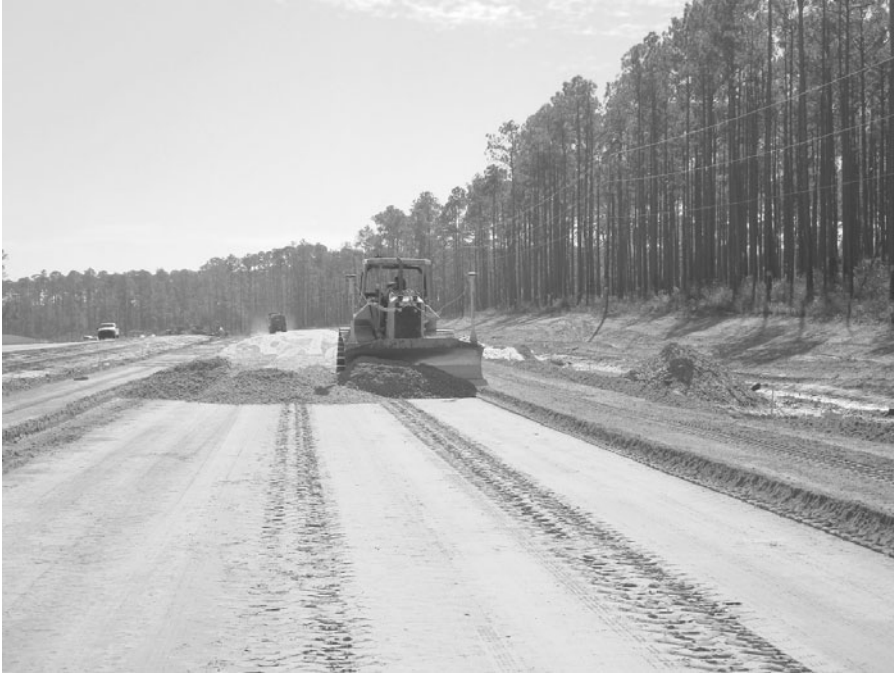
FIGURE 5.2 Constructing aggregate base before placing the hot-mix asphalt or portland cement concrete layer of a paved road.
