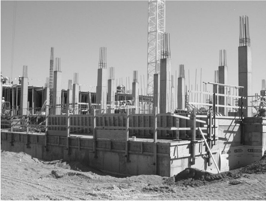
FIGURE 3.13 Steel rebars used to reinforce PCC columns.
