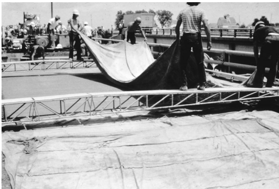
FIGURE 7.26 Curing concrete with impervious fabrics.
