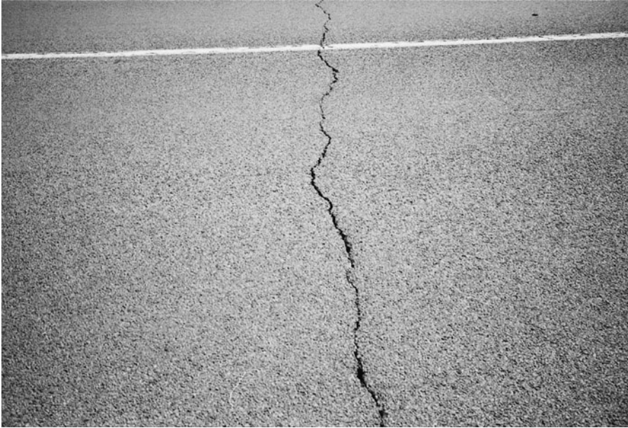
FIGURE 9.12 Thermal cracking resulting from the use of too-stiff asphalt in a cold climate area.
