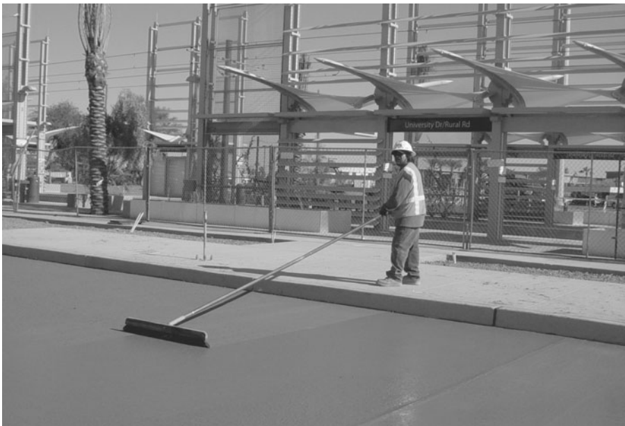
FIGURE 7.17 Finishing concrete manually with a straightedge.
