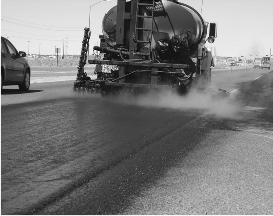
FIGURE 9.8 Spraying tack coat (emulsion) on existing asphalt pavement before placing an asphalt overlay.
