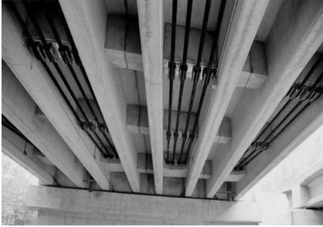
FIGURE 11.10 Strengthening a concrete bridge with FRP polymer bars.
