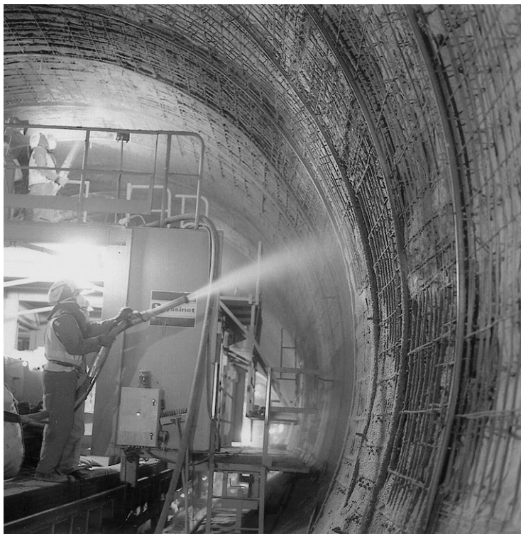
FIGURE 7.45 Shotcrete used in lining a tunnel (Courtesy of the American Shotcrete Association).
