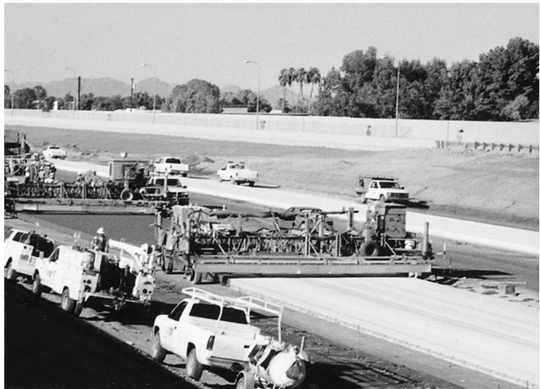
FIGURE 7.29 Curing concrete by machine applying membrane forming compound.
