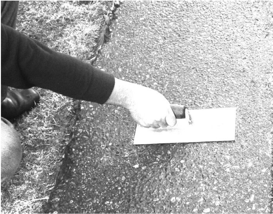
FIGURE 7.16 Finishing concrete with a trowel.
