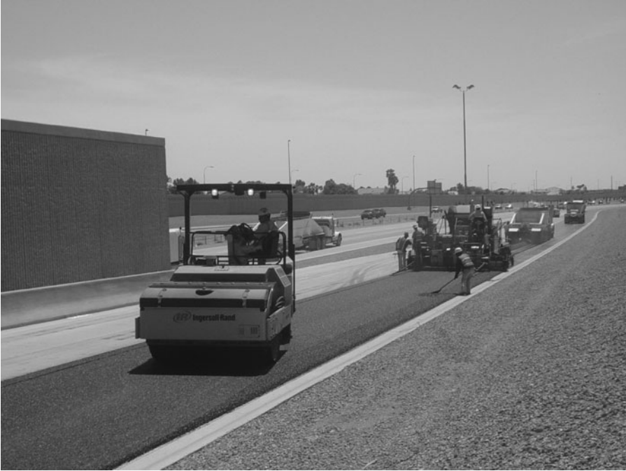
FIGURE 9.6 Compaction of hot mix asphalt.
