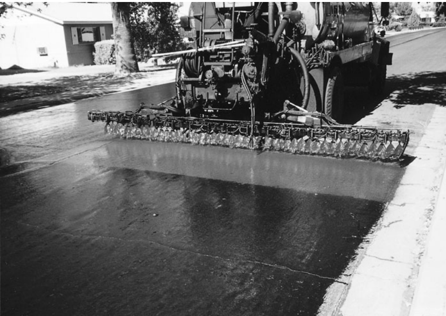
FIGURE 9.7 Applying fog seal (diluted emulsion) for preserving existing pavement.
