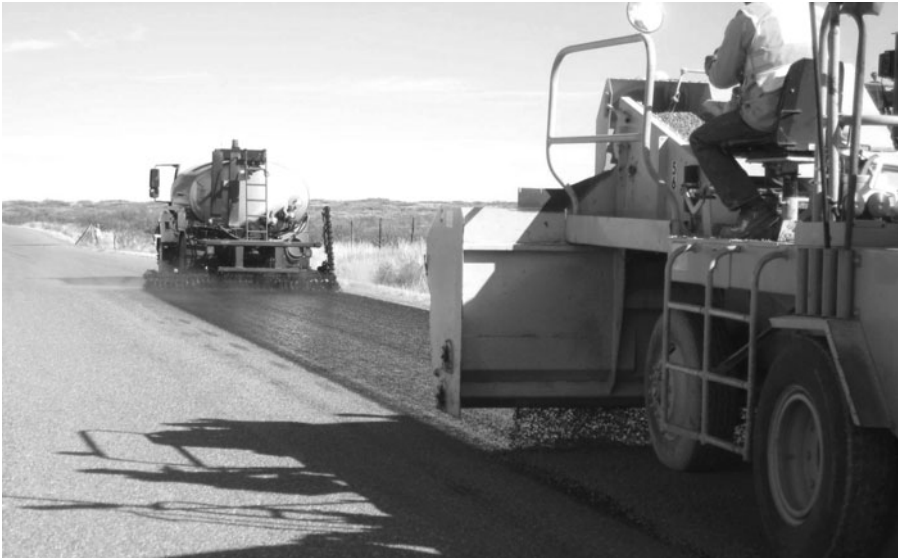
FIGURE 9.9 Applying chip seal (emulsion followed by aggregates) for preserving existing pavement.
