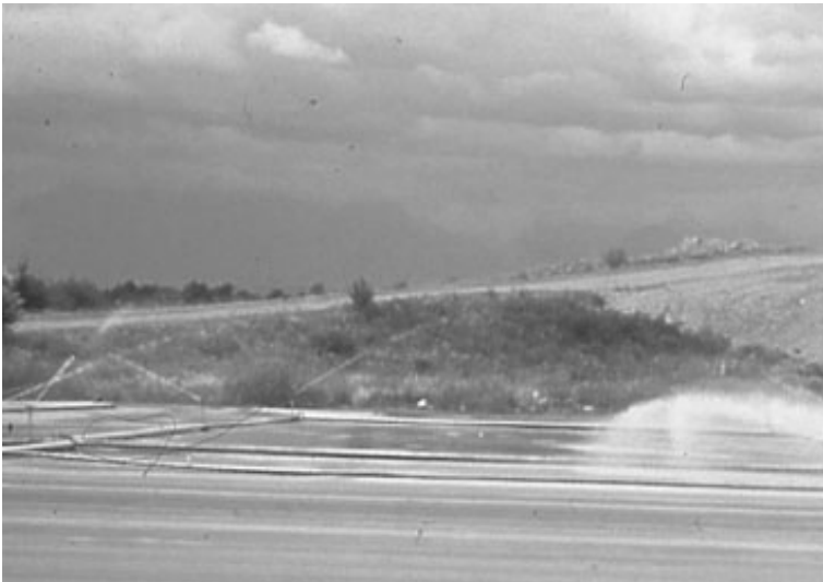
FIGURE 7.23 Curing concrete by spraying.
