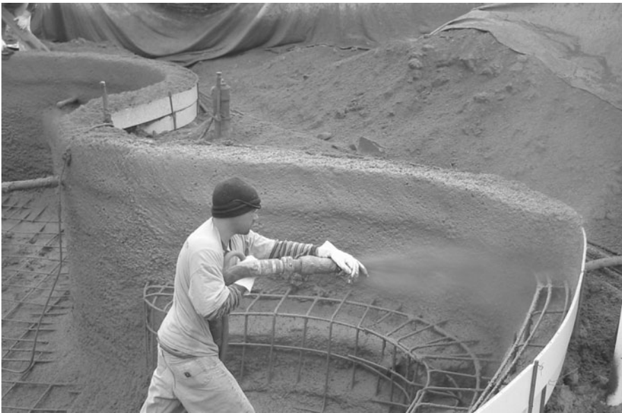
FIGURE 7.44 Constructing a swimming pool using shotcrete (Courtesy of the American Shotcrete Association).
