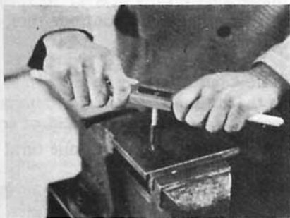
Figure 10 Starting the tap
