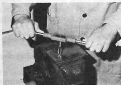
Figure 11 Tapping the hole
