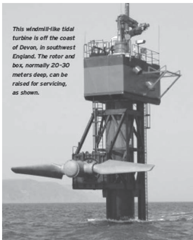
Figure 3-6. Underwater turbine and column-mounted generator. (From [6], © IEEE 2003.)
