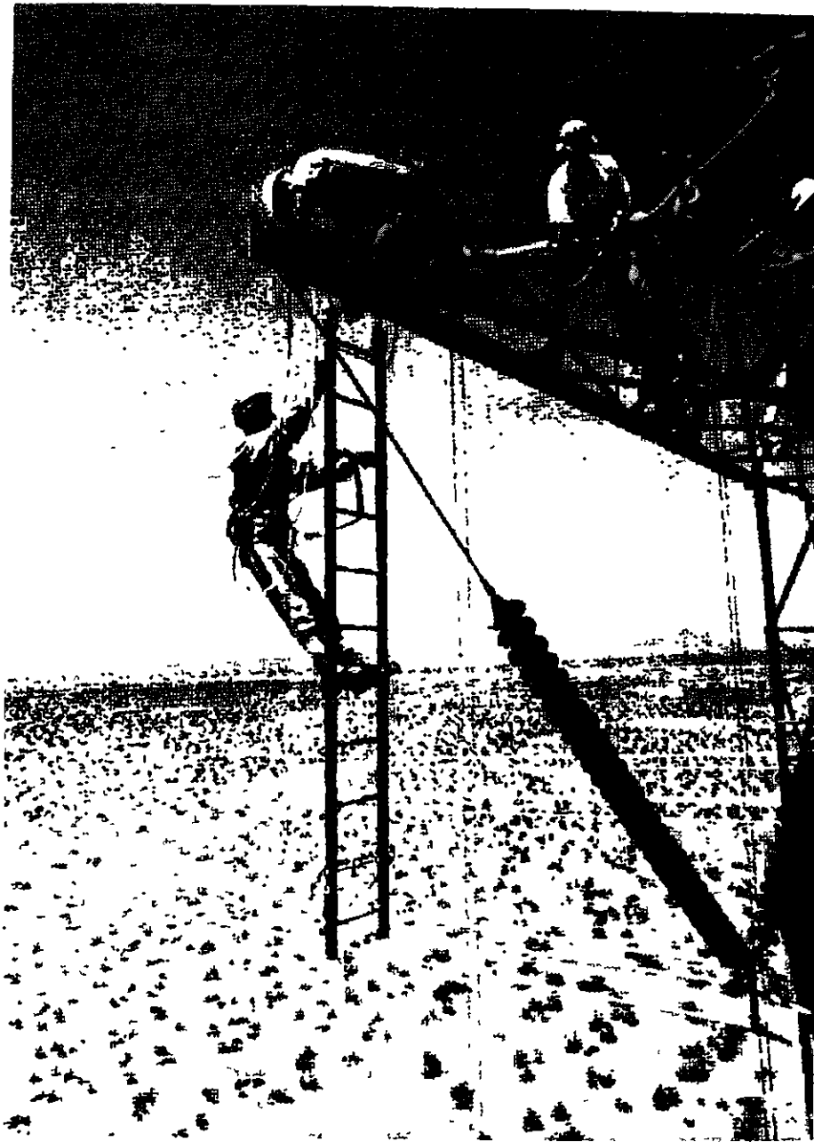
Figure 9.20. Installing vee arrangement of suspension insulator strings carrying four bundled conductors per phase at 500 kV. (Courtesy of Ohio Brass Company.)
