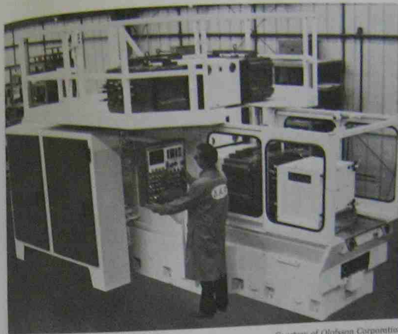
Fig. 9-9. Large multispindle heads are changed automatically with the machine shown above. Although, in this instance, the parts are not automatically changed as described in the other figures, 9-7 through 9-13, the machine is well suited to medium volume applications as are the other machines shown in Figs. 9-7 through 9-13.
