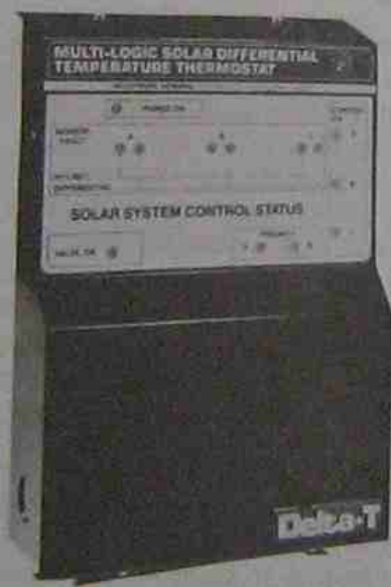
Figure 34-29. A typical modern controller for a space-heating-solar system. Courtesy Heliotrope General
