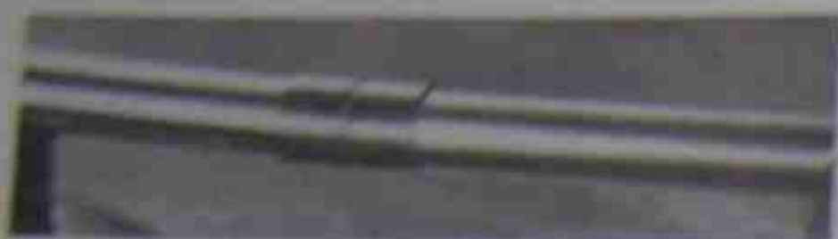
Figure 6-19B. A properly assembled and supported joint ready to be soldered. Photo by Bill Johnson.
