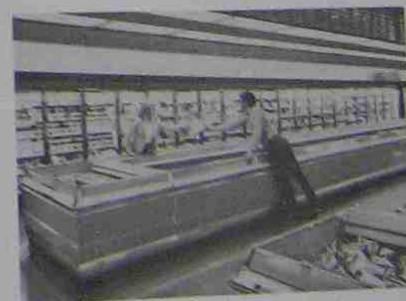
Figure 24-1. Display cases used to safely store food displayed for sale. Some display cases are open to allow the customer to reach in without opening a door; some have doors. Closed cases are the most energy efficient. Courtesy Hill Refrigeration
