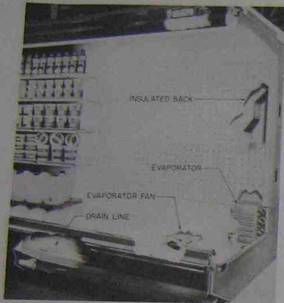
Figure 24-13. Dairy case showing the location of the evaporator. Courtesy Hill Refrigeration
