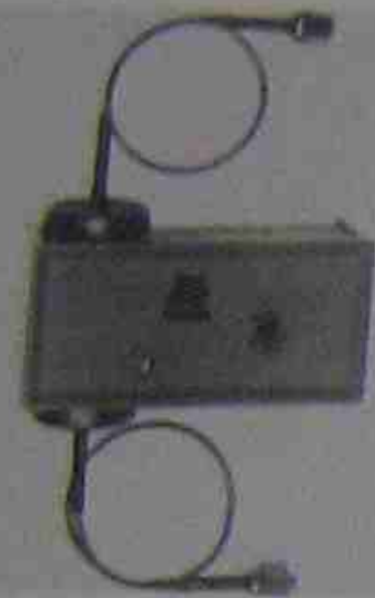
Figure 23-26. Oil safety controls have a bellows on each side of the control. They are opposed in their forces and serve to measure the net oil pressure; the difference in the suction pressure (oil pump inlet) and the oil pump outlet pressure. This control has a 90 second time delay to allow the compressor to get up to speed and establish oil pressure before it shuts down. Courtesy: Ranco
