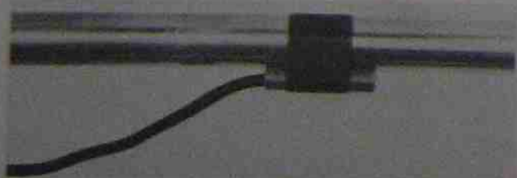
Figure 12-24. Thermistor application. Photo by Bill Johnson
