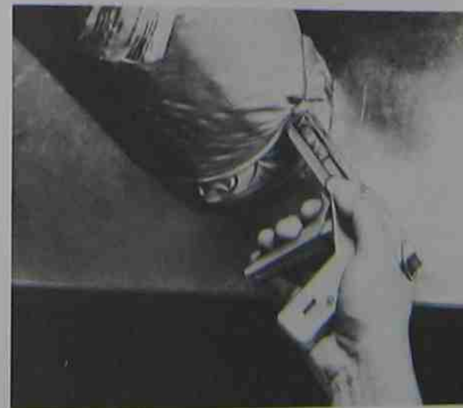
Figure 5-18. A system for fastening round flexible duct to a sheet metal collar. Courtesy Panduit Corporation
