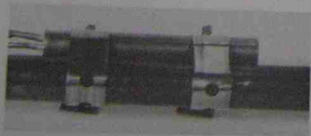
Figure 14-12. Correct way to get good contact with a sensing bulb and the suction line. Bulb is mounted on a straight portion of the line with a strap that holds it secure against the line. Photo by Bill Johnson
