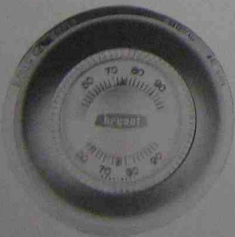
Figure 41-14. This is a typical room thermostat. It is a combination heating and cooling thermostat with a bimetal element for sensing room temperature. Photo by Bill Johnson
