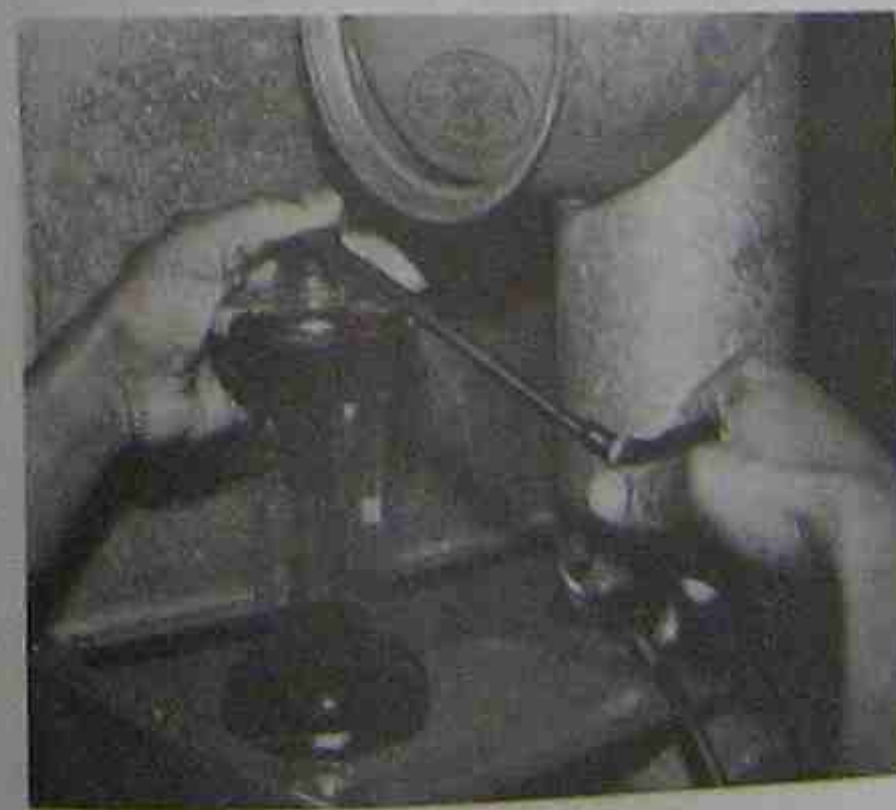
Figure 32-60. Making CO 2 test. Photo by Bill Johnson
