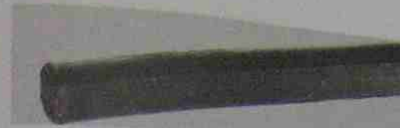
Figure 29-5. Motor shaft damaged from trying to drive it through the pulley. Photo by Bill Johnson
