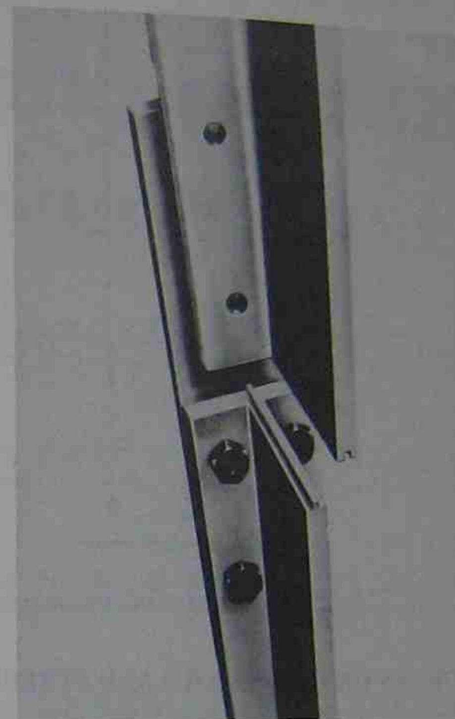
Fig. 7.2 — Guide-rail jointing.
