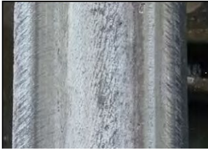
Light Spalling
