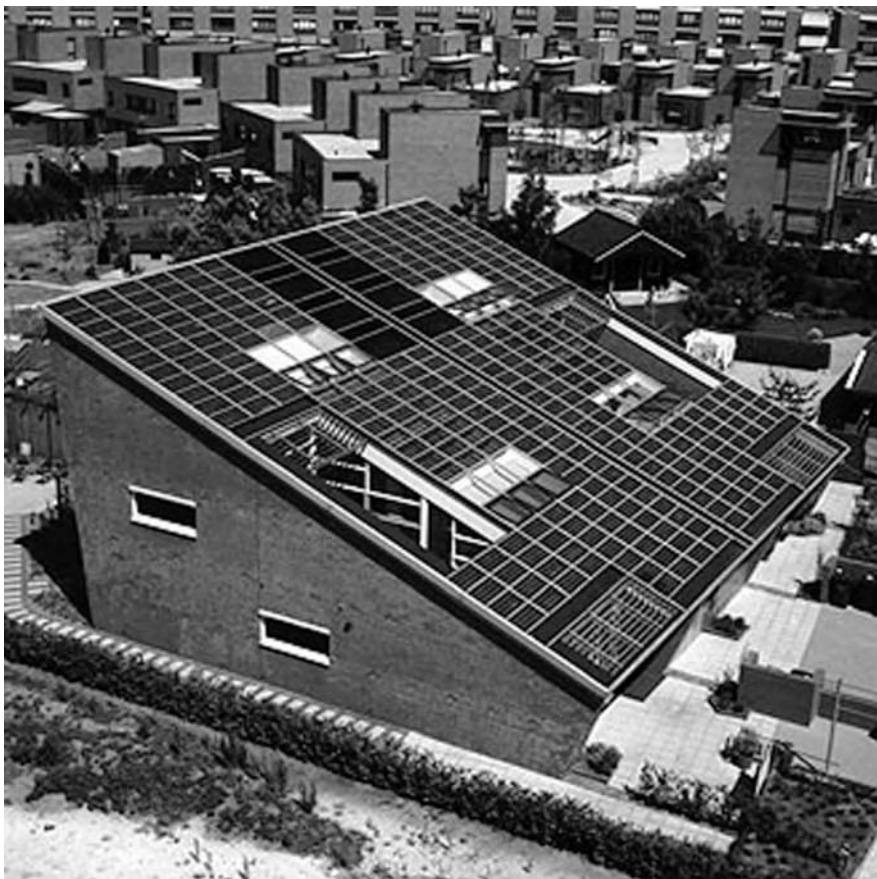
FIGURE 2.3 Roof-mounted Dutch PV subdivision, Nieuwland, in Amersfoort.
