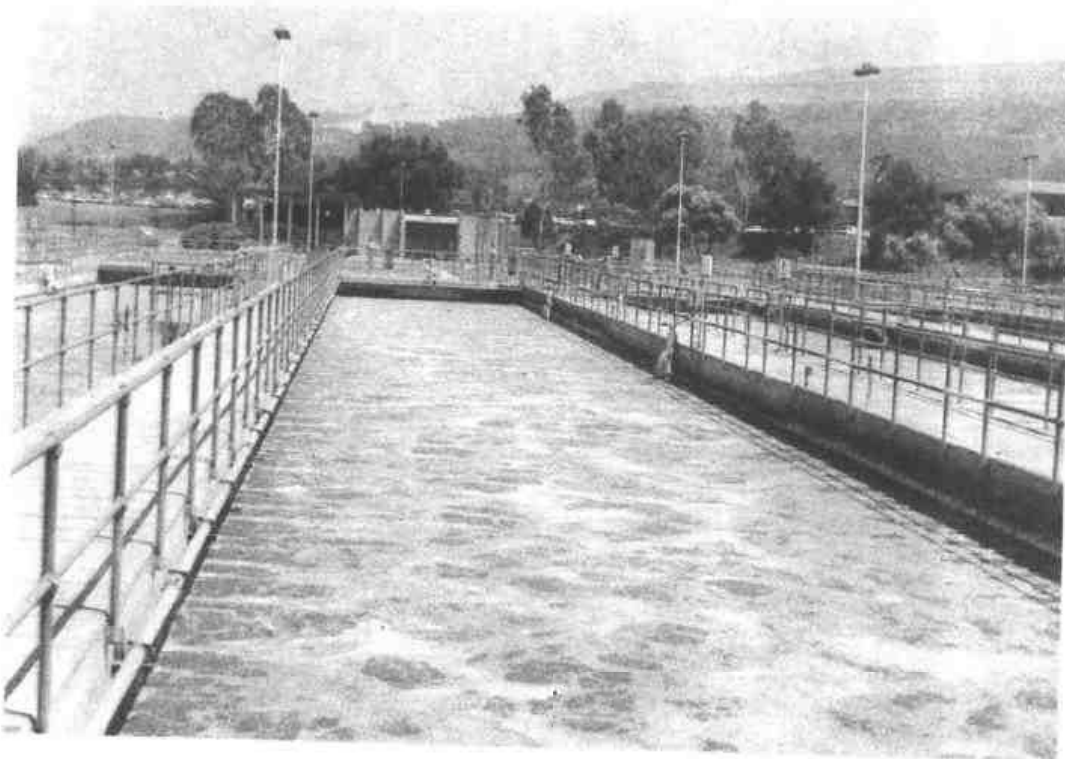
FIGURE 7.16 Plug flow activated sludge process.
