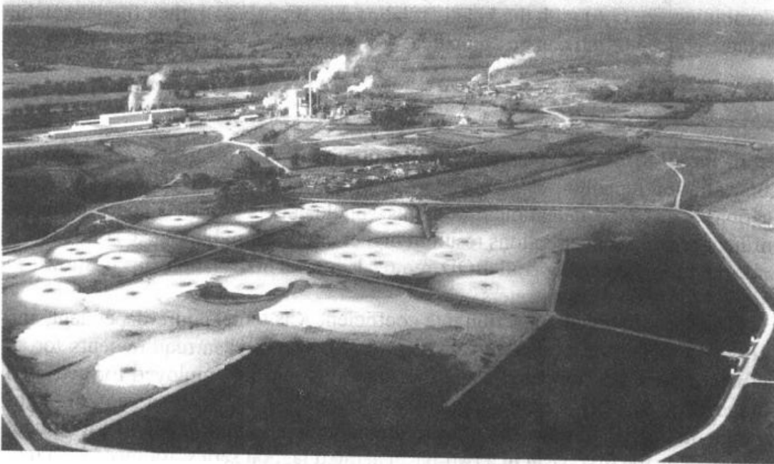
FIGURE 7.7 Aerated lagoon treating pulp and paper mill wastewater.
