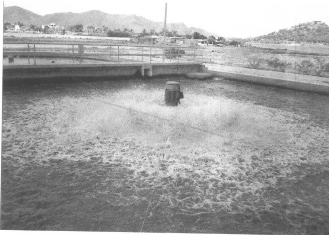
FIGURE 5.17 High speed surface aerator ( courtesy of Aqua Aerobic Systems Inc. ).
