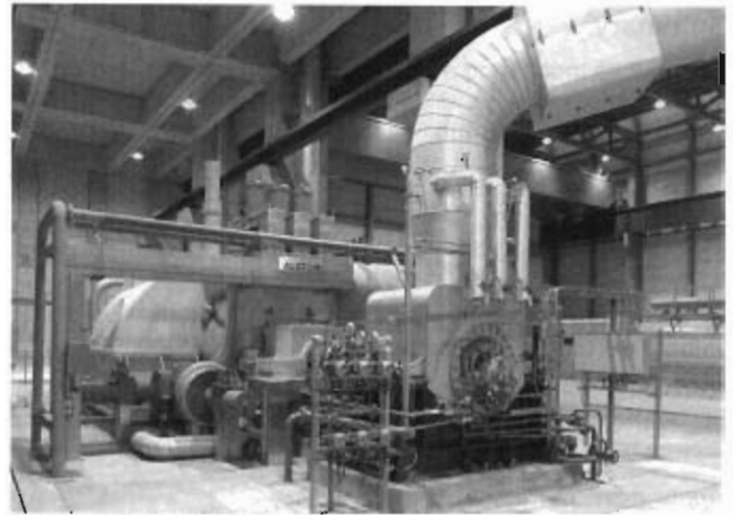
Figure 16.78 A booster pump Courtesy KSB AG
