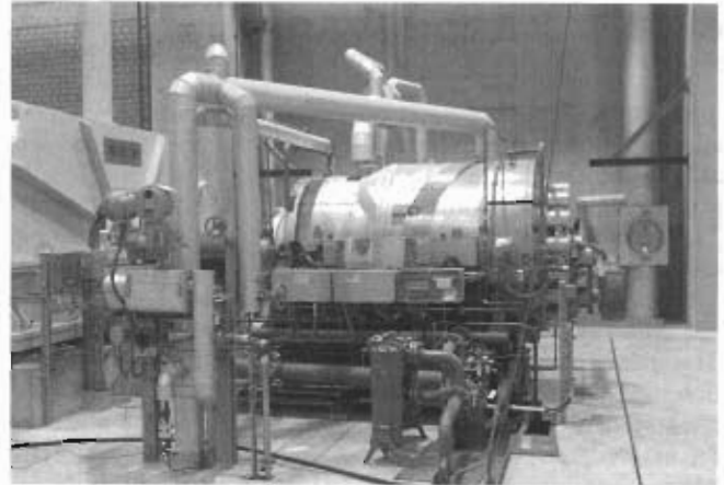
Figure 16.88 Side view of the boiler feed pump Courtesy KSB AG
