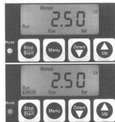
Figure 16.71 Display when pump is functioning correctly (upper). Display when there is a flow error (lower) Courtesy of Aildos Ltd
