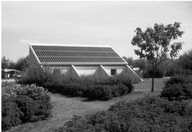
**Figure 22.13** A naturally integrated PV system that is clearly part of the building. This system is located in Poitiers (FR). Reproduced with permission by ECN J. Beurskens
