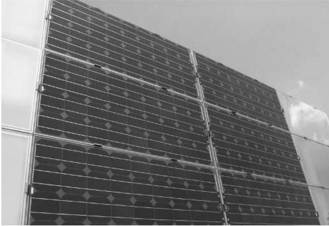
**Figure 22.40** BP Solface vertical wall system at the Demosite in Lausanne (CH). Reproduced with permission by EPFL-LESO-PB
