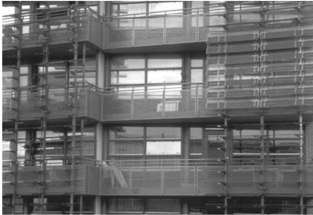
**Figure 22.41** ADO louver system with integrated transparent PV modules at an apartment building in Amersfoort Nieuwland (NL). The automatic louvers can switch in two positions. The horizontal position at night (left on the figure) and tilted to the sun by day (right on the figure). Reproduced with permission by BEAR Architecten T. Reijenga
