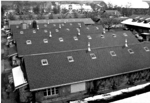
**Figure 22.15** The 80.5 kWp Atlantis Sunslates on the roof of the historic horse stables in Bern (CH). The color and texture matches so well that this PV system was allowed on a protected historic building. Reproduced with permission by Atlantis Solar Systems Ltd
