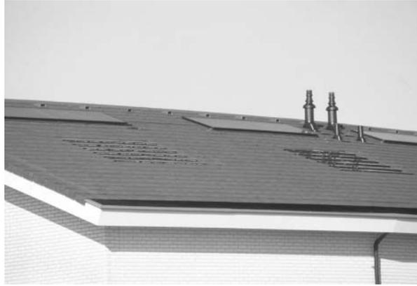
**Figure 22.12** This sustainable WWF (World Wildlife Fund) project in Harderwijk (NL) has a roof with a thermal solar collector on top and a 460 Wp PV 700 system underneath. The PV 700 system fits almost invisibly in between the tiles. Reproduced with permission by BEAR Architecten T. Reijenga
