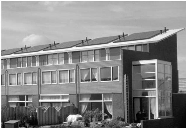
**Figure 22.22** These houses in Amersfoort Nieuwland (NL) have a roof with a white foil on top. The architect chose a color contrasting with the color of the modules to show that the PV system is an addition to his design. Reproduced with permission by REMU J. van IJken
