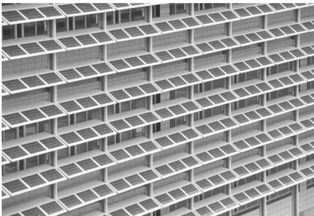
**Figure 22.11** South façade of ECN Building 31 in Petten (NL). The shading structure supports the 35 kWp Shell Solar modules. Reproduced with permission by BEAR Architecten T. Reijenga
