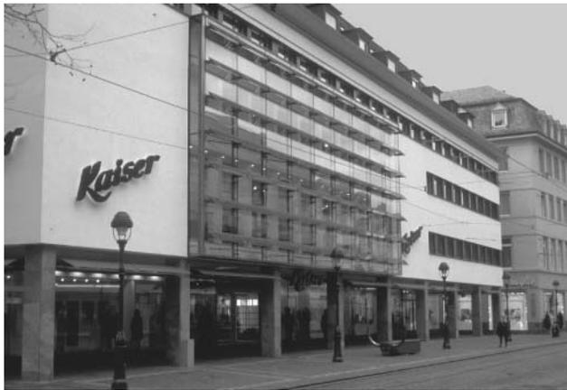
**Figure 22.10** Daylight control at the Kaiser fashion house in Freiburg (D). This 4 kWp PV system on louvers is mounted in front of the glass façade and prevents glare inside. The PV louvers are in the center of the figure. Reproduced with permission by BEAR Architecten T. Reijenga
