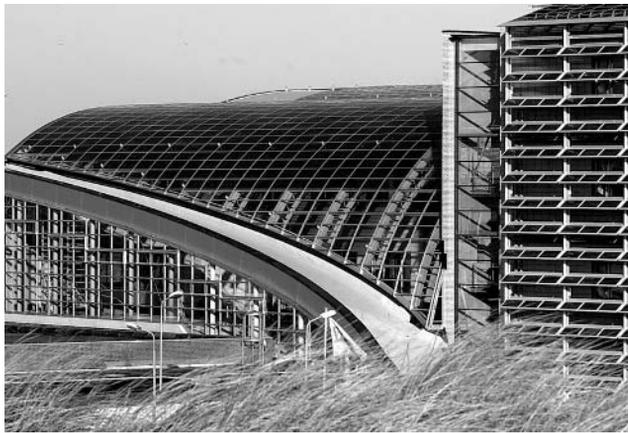
**Figure 22.43** This building, at ECN in Petten (NL) has a 43 kWp PV system integrated into the conservatory roof. The conservatory acts as a parasol in front of the offices, thus eliminating the need for air-conditioning in a moderate climate. The building on the right side has a PV shading system (see caption on Figure 22.11). Reproduced with permission by BEAR Architecten T. Reijenga
