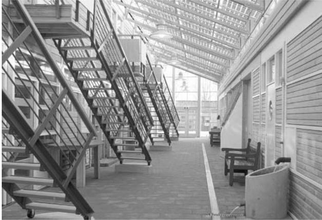
**Figure 22.14** Corridor in the Centre for Sustainability De Kleine Aarde in Boxtel (NL). The space is unheated and naturally ventilated. The 6.7 kWp PV system with transparent modules has a double function and reduces the heat load by around 70%. Reproduced from Reijnga T, Böttger W, *Proc. 2<sup>nd</sup> WC Photovoltaic Solar Energy Conversion*, 2748–2751 (1998) with permission by NOVEM, R Schropp [11]
