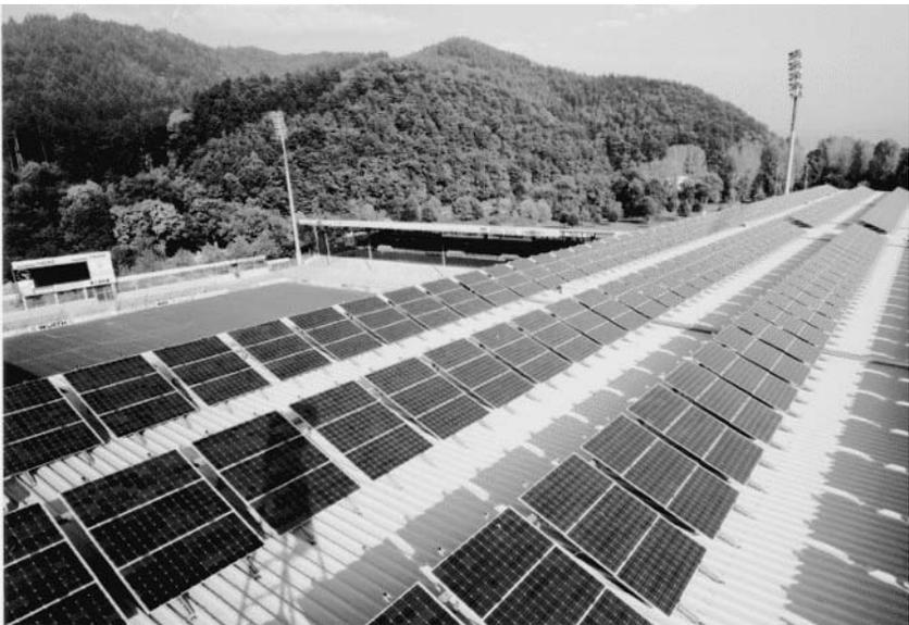
**Figure 17.30** Joint ownership PV installation of 100 kW on the soccer stadium Freiburg, Germany [27]
