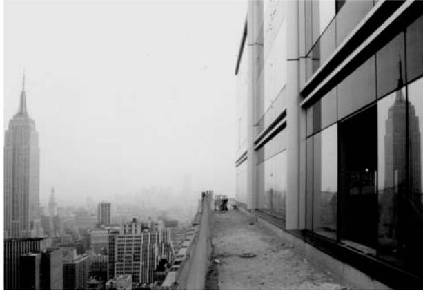
**Figure 22.2** Integrated façade system with 14 kWp amorphous silicon modules made by Energy Photovoltaics (EPV) in New Jersey, USA on top of a skyscraper at Four Times Square, New York, USA. The PV modules are the dark regions on the facade near the top. Reproduced from Kiss G, *Proc. 2<sup>nd</sup> WC Photovoltaic Solar Energy Conversion*, 2452–2455 (1998) with permission by Gregory Kiss [7]
