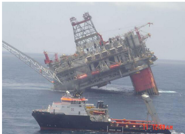
Figure 7.3 Lack of adequate buoyancy for semi-submersible platform.
