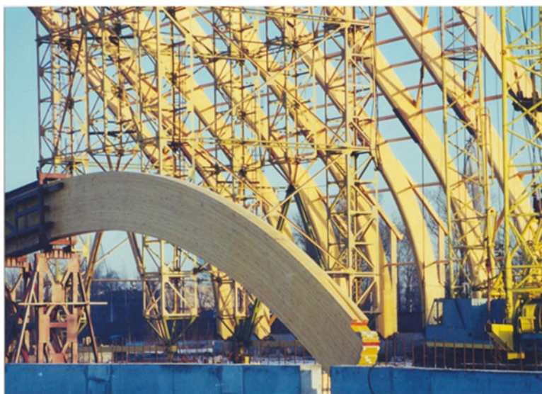
Fig. 8.2 Structure of a mineral fertilizer warehouse in the port of St. Petersburg
