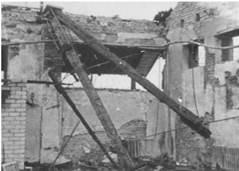
Fig. 8.4 The collapse of wooden structures in a fire due to loss of strength of steel connections
