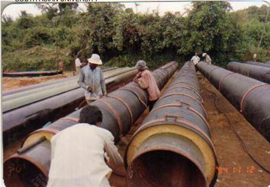
Image 2 : MS pipe with PUF insulation and HDPE jacketing.
