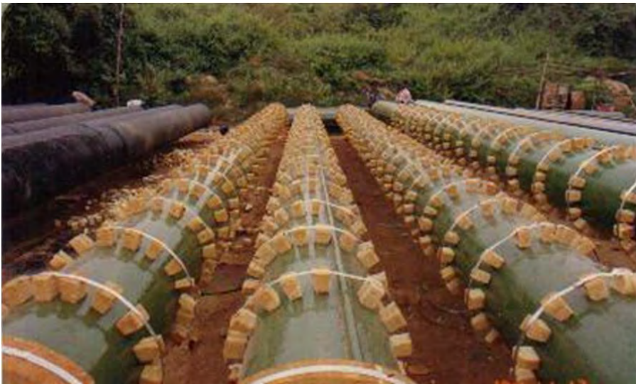
Image 1 : MS pipe with PUF spacer blocks.
