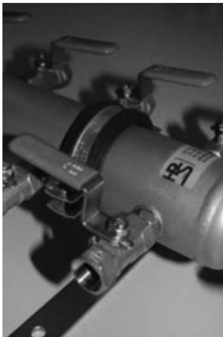
Figure 6.7 Typical pressure regulator (with kind permission from HPS).
