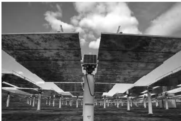
Figure 2.26 Direct solar radiation is collected by a field of 300 heliostats, each with a surface area of 40 m 2 . The heliostats are operated to follow the sun by a computer-driven servo motors, reprinted by permission of Arno A. Evers, FAIR-PR, Founder (1995) of the Group Exhibit Hydrogen and Fuel Cells at the Annual Hannover Fair.
